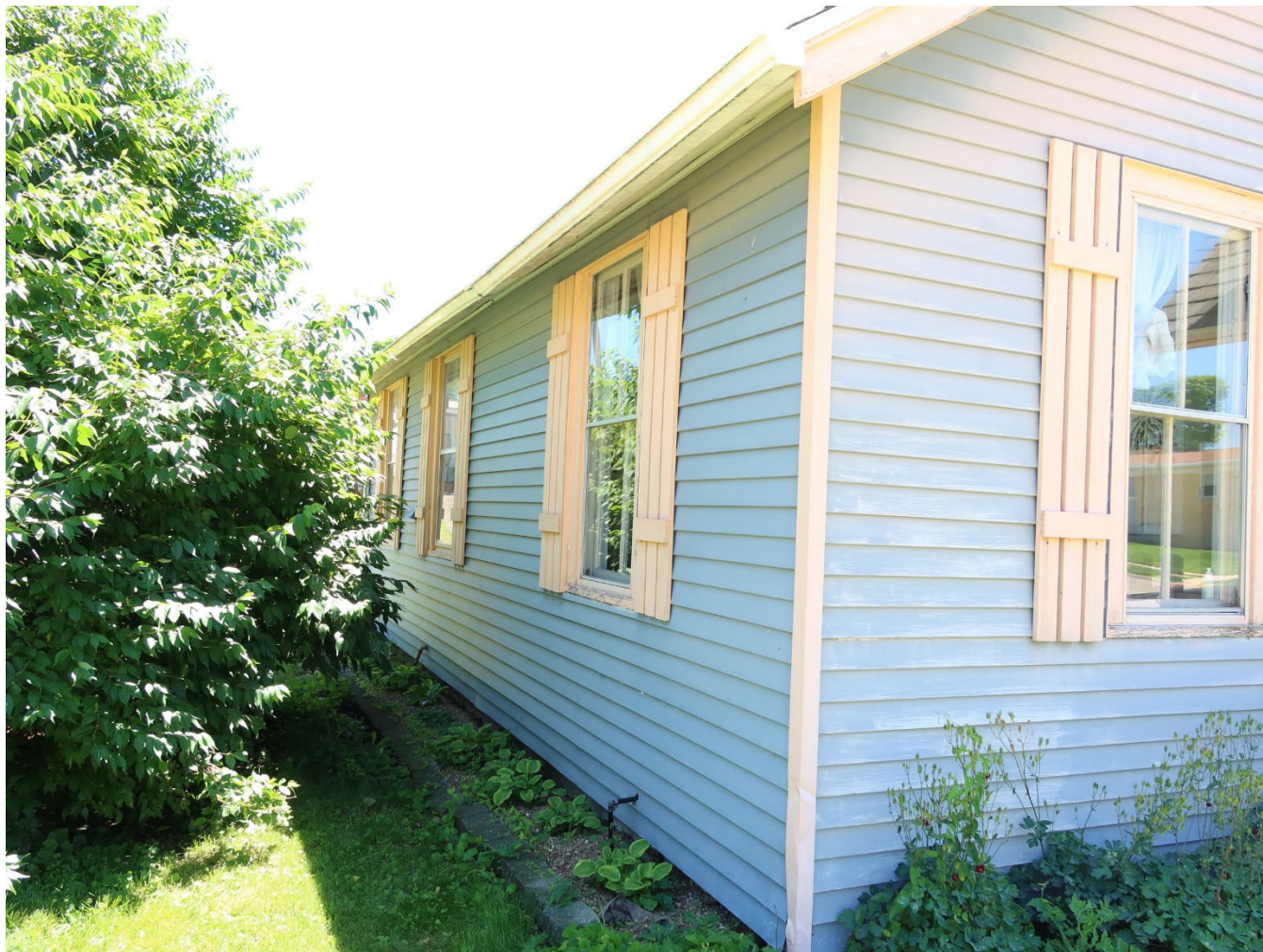
Photograph 44-02279-002. North elevation, looking southeast (June 2024)
