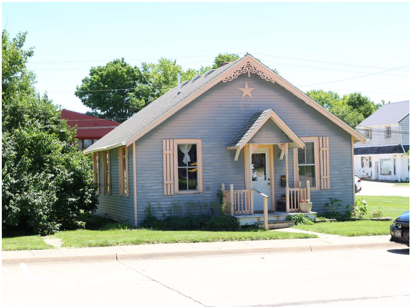
Photograph 44-02279-001. West elevation, looking southeast (June 2024)
