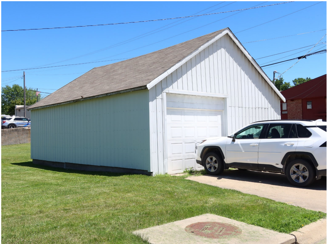
Photograph 44-02279-005. Garage, looking northeast (June 2024)
