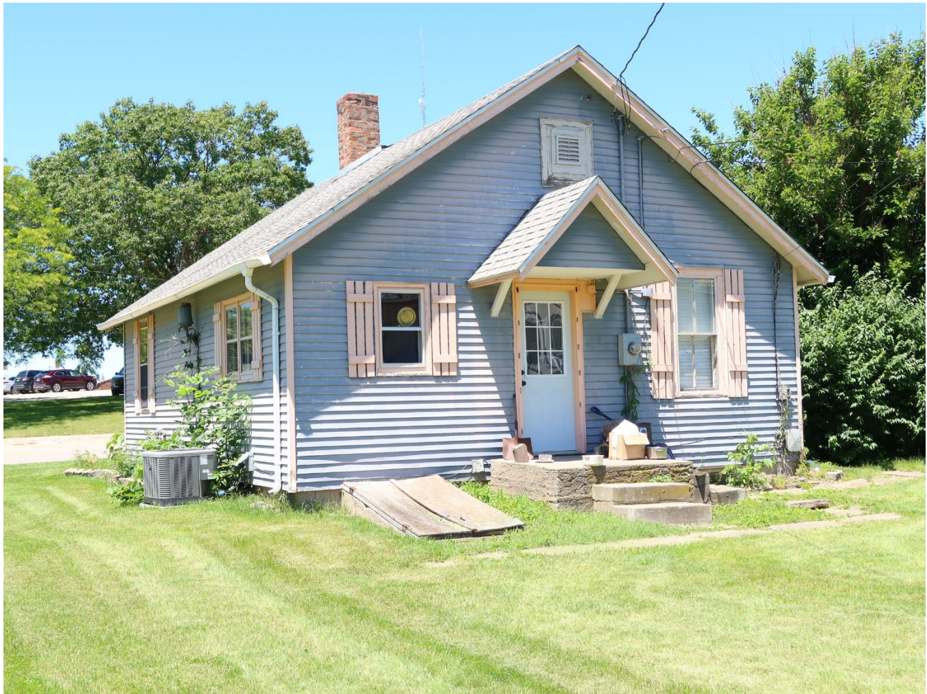
Photograph 44-02279-004. East elevation, looking northwest (June 2024)
