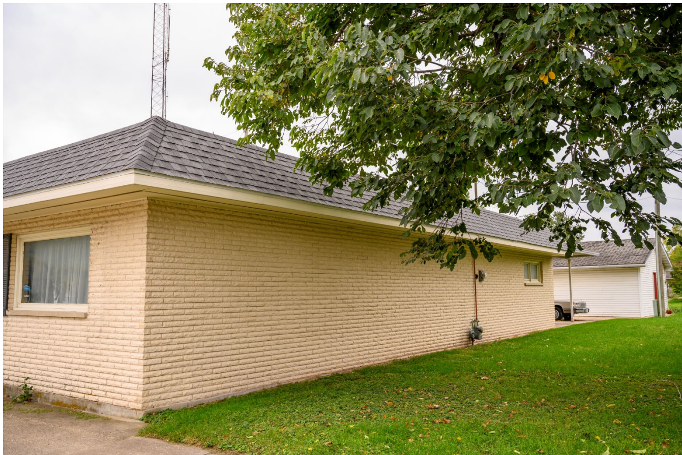
Photograph 44-02233-004. West elevation, looking southeast (October 2023)
