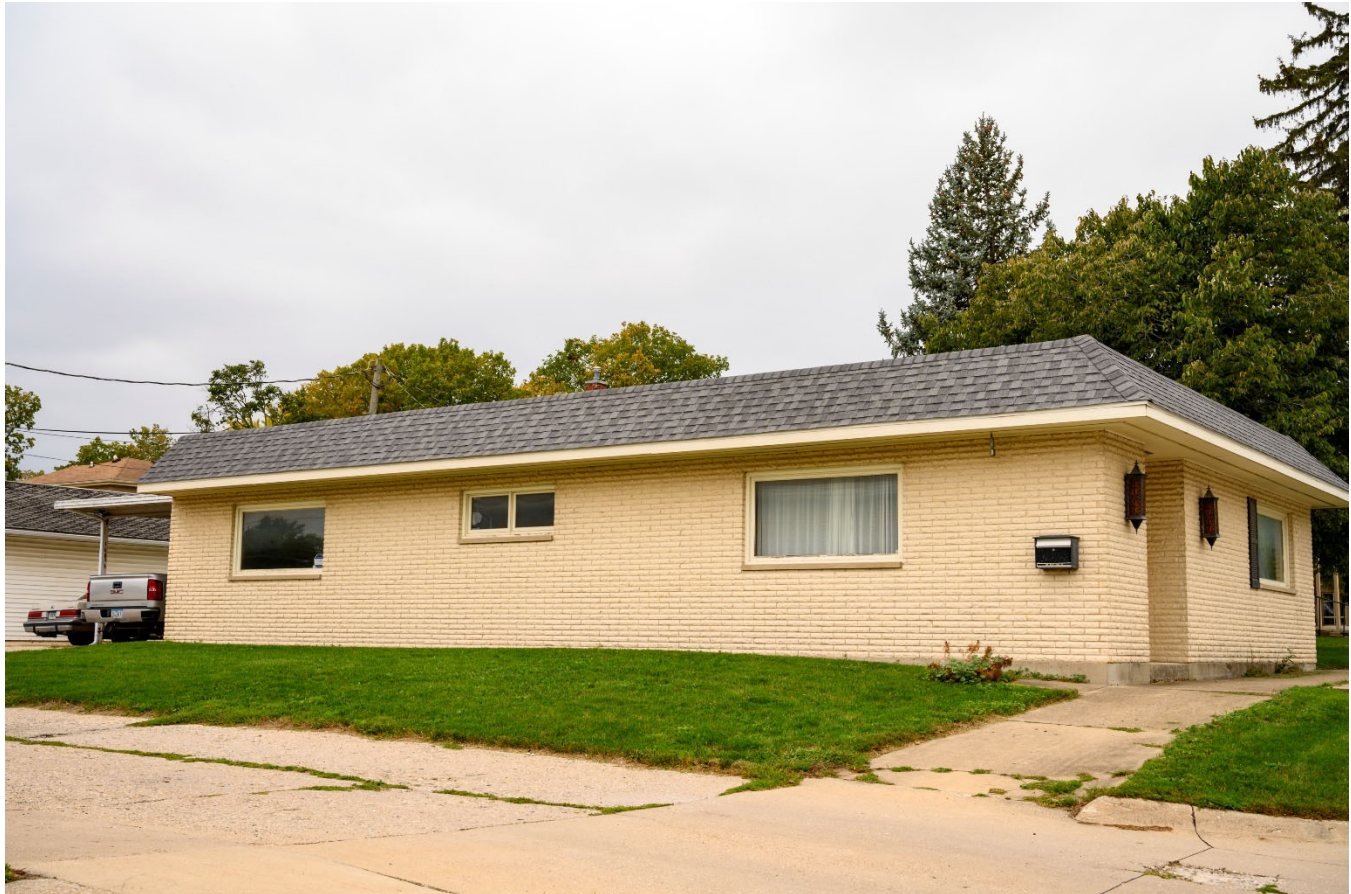
Photograph 44-02233-002. East elevation, looking southwest (October 2023)
