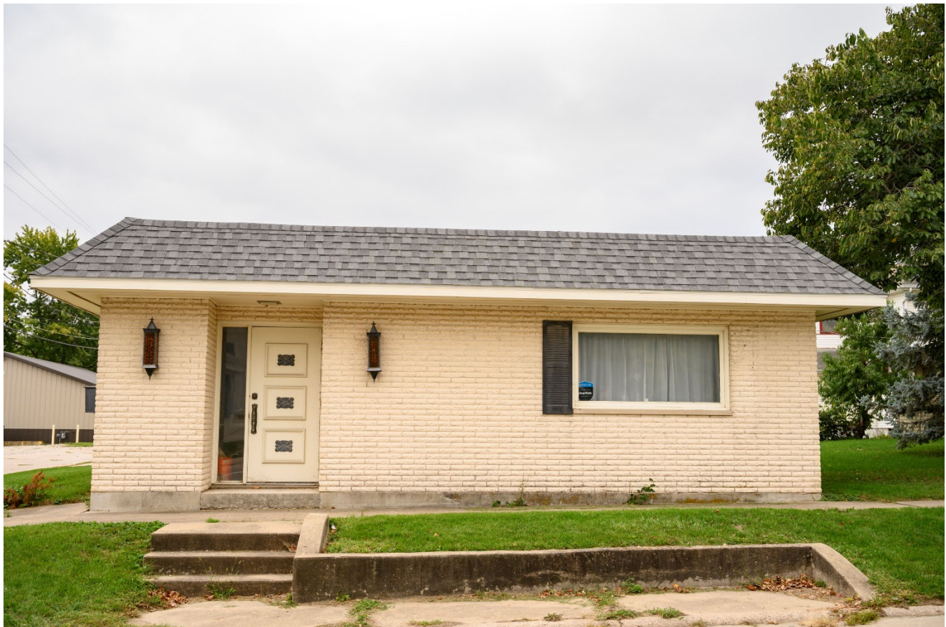
Photograph 44-02233-001. North elevation, looking south (October 2023)
