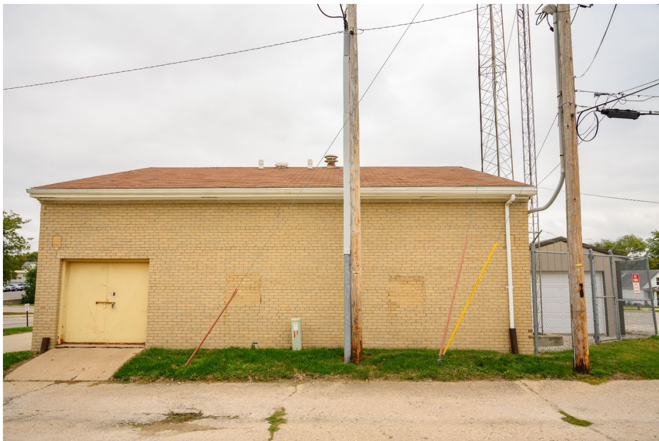
Photograph 44-02235-002. West elevation, looking east (October 2023)
