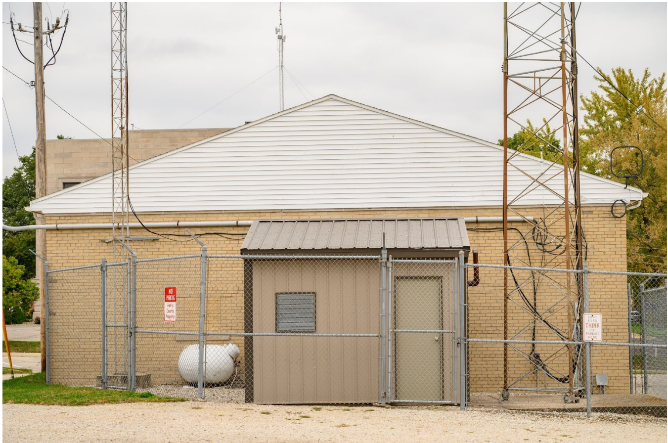
Photograph 44-02235-004. South elevation, looking north (October 2023)
