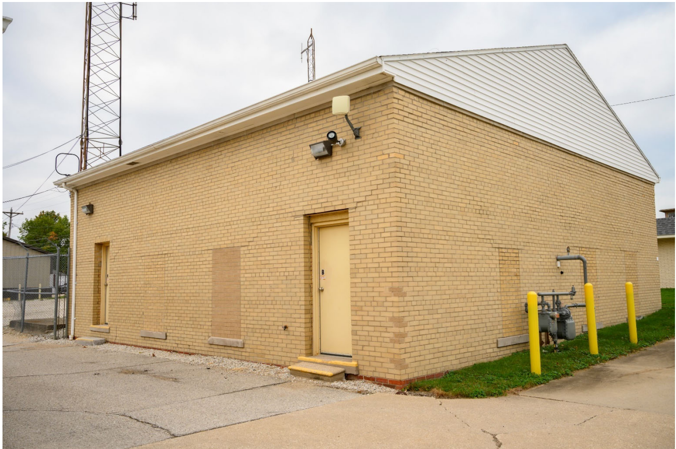
Photograph 44-02235-001. East and north elevations, looking southwest (October 2023)
