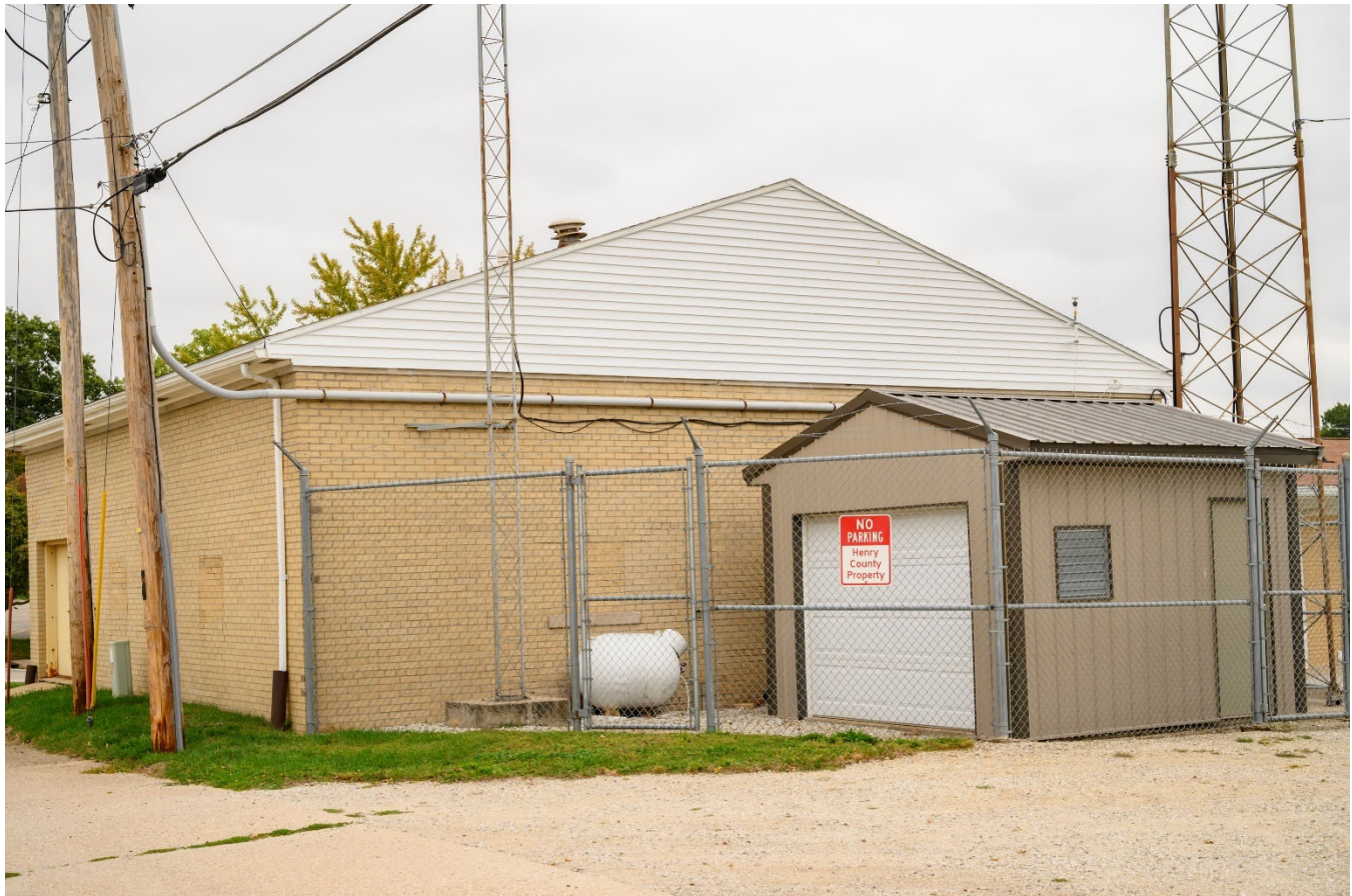
Photograph 44-02235-003. West and south elevations, looking northeast (October 2023)
