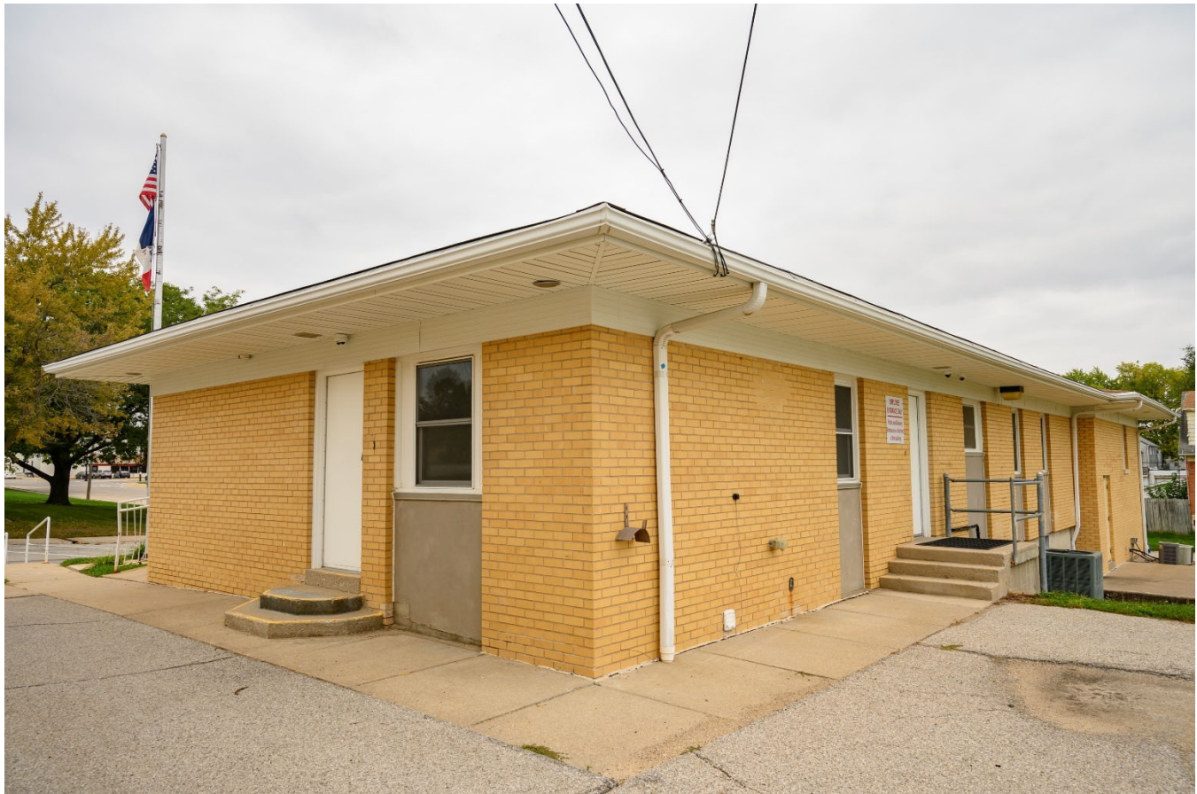
Photograph 44-02234-003. West and south elevations, looking northeast (October 2023)
