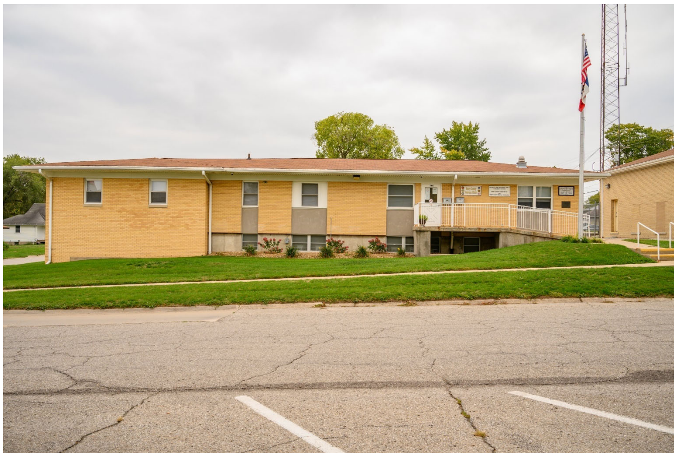
Photograph 44-02234-001. North elevation, looking south (October 2023)
