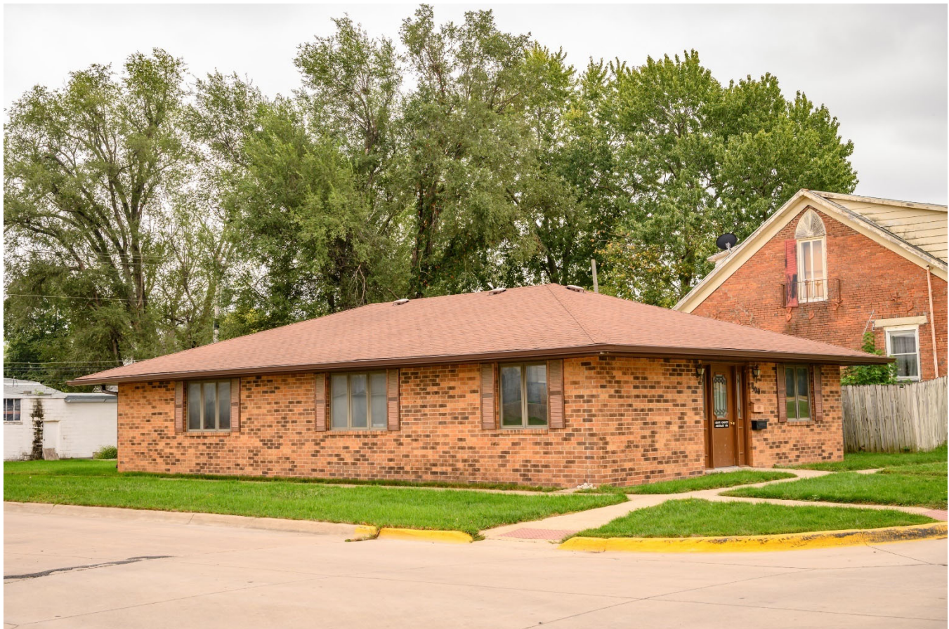
Photograph 44-02232-001. North and west elevations, looking southeast (October 2023)
