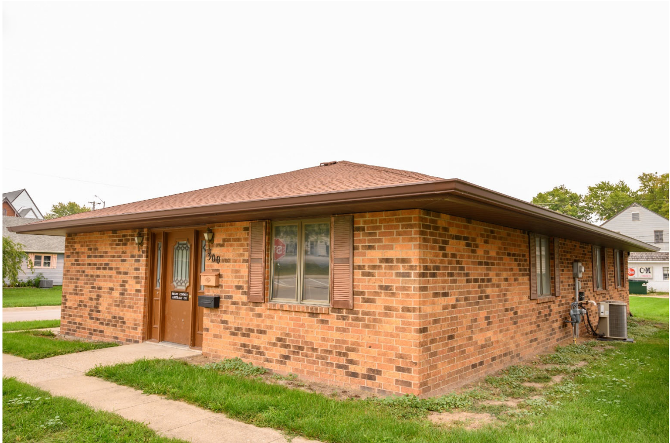
Photograph 44-02232-002. West and south elevations, looking northeast (October 2023)
