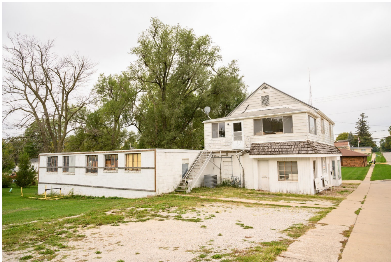
Photograph 44-02236-003. East elevation, looking west (October 2023)
