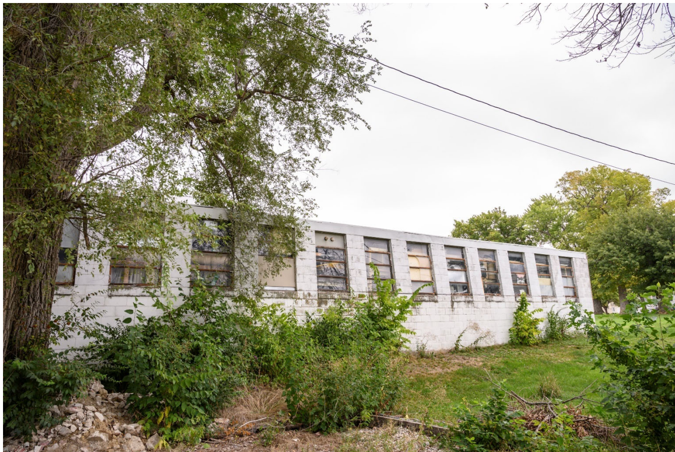
Photograph 44-02236-004. South elevation, looking north (October 2023)
