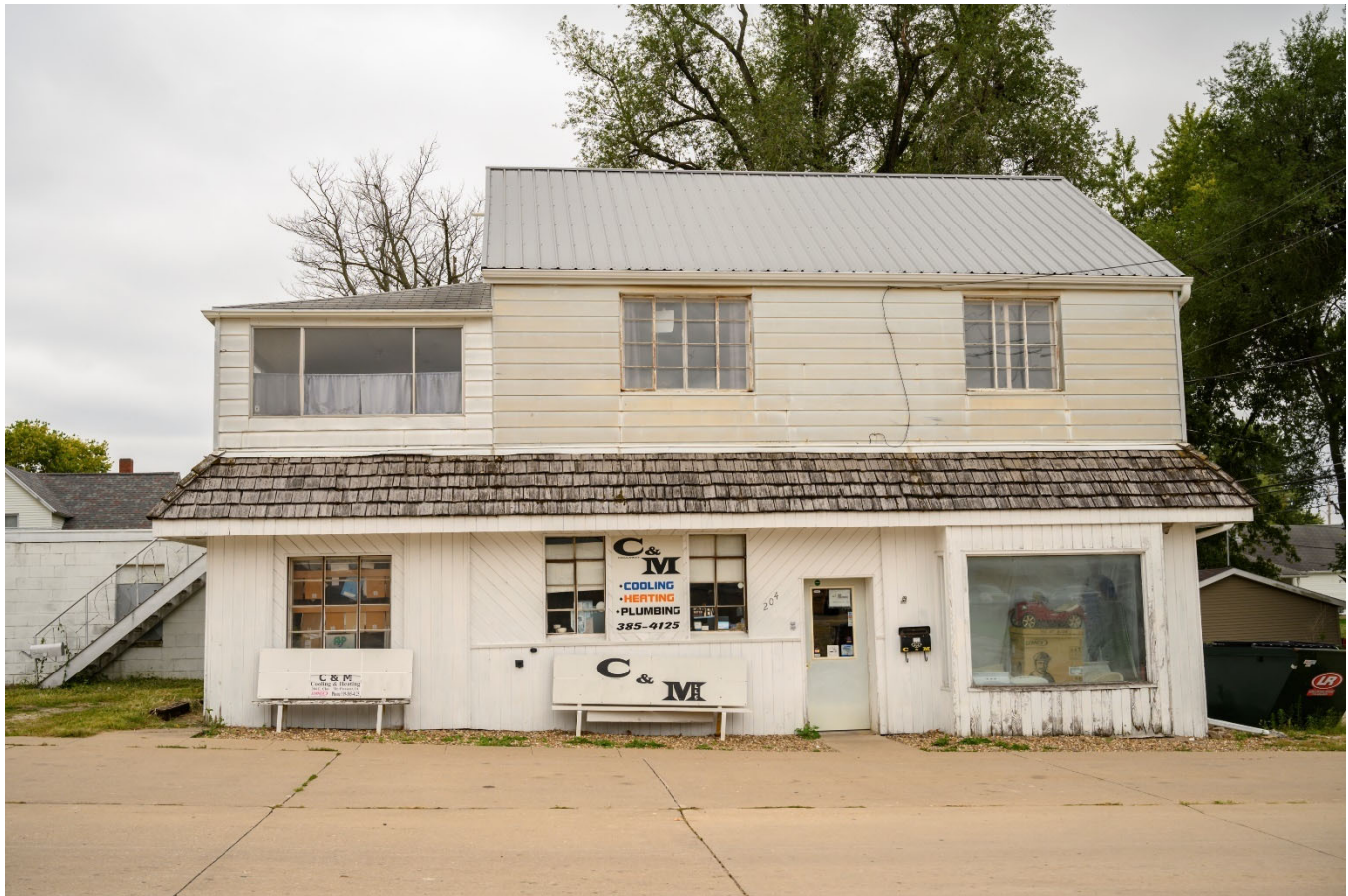
Photograph 44-02236-001. North elevation, looking south (October 2023)
