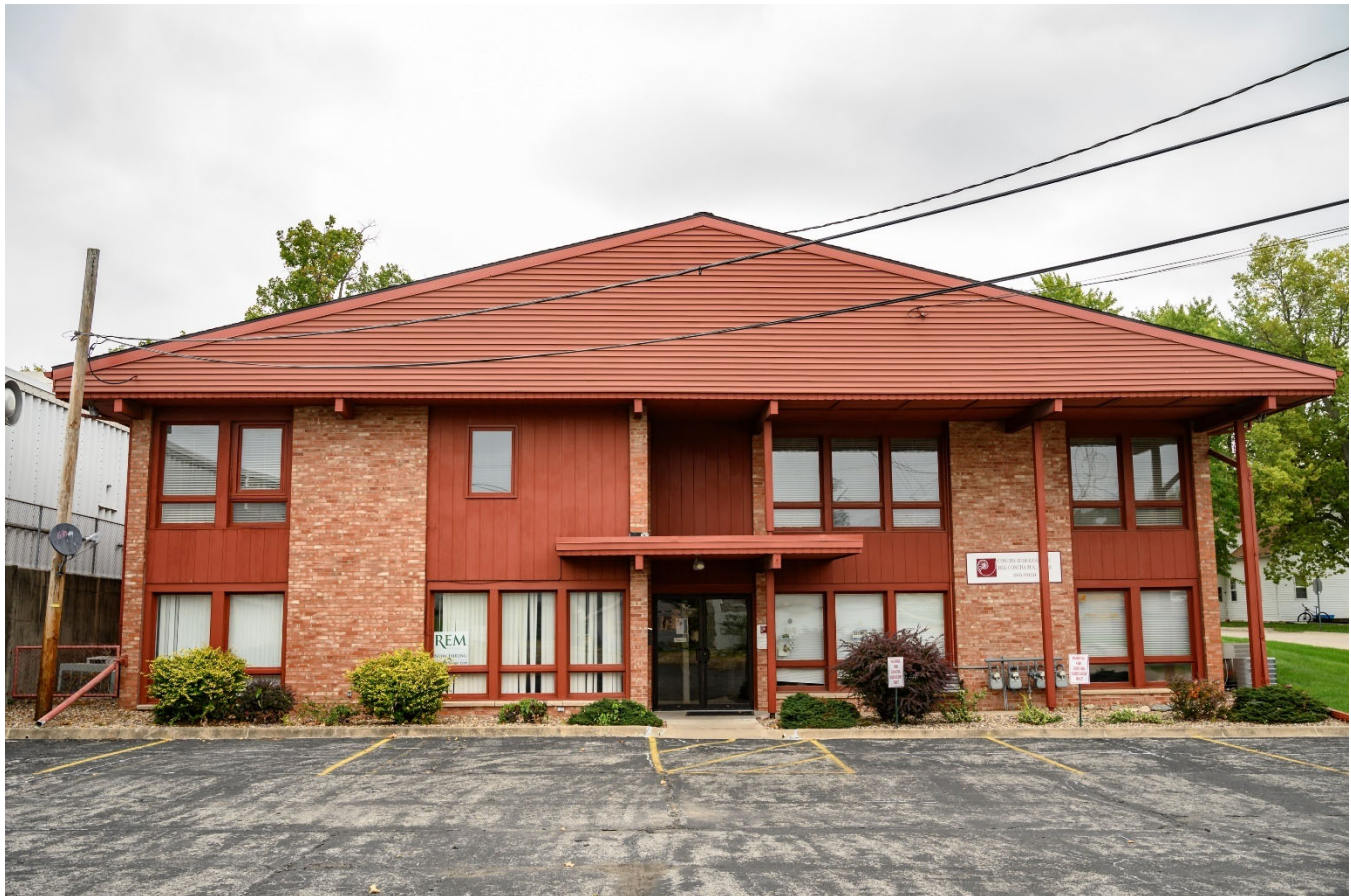
Photograph 44-02238-003. West elevation, looking east (October 2023)
