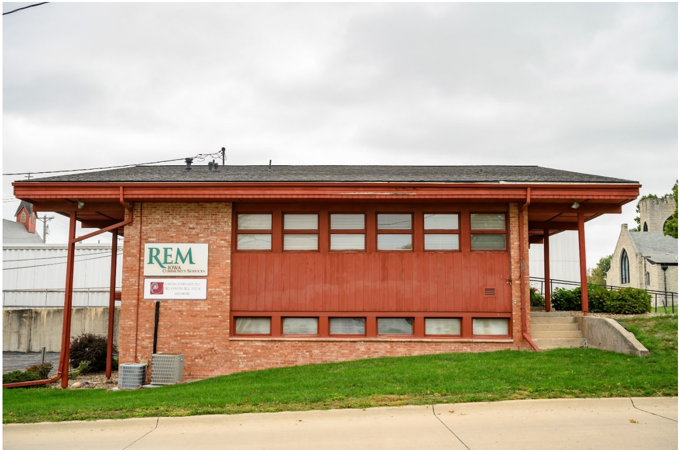
Photograph 44-02238-002. South elevation, looking north (October 2023)
