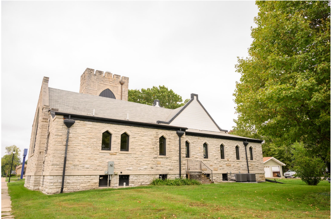
Photograph 44-02274-006. South elevation, looking north (October 2023)
