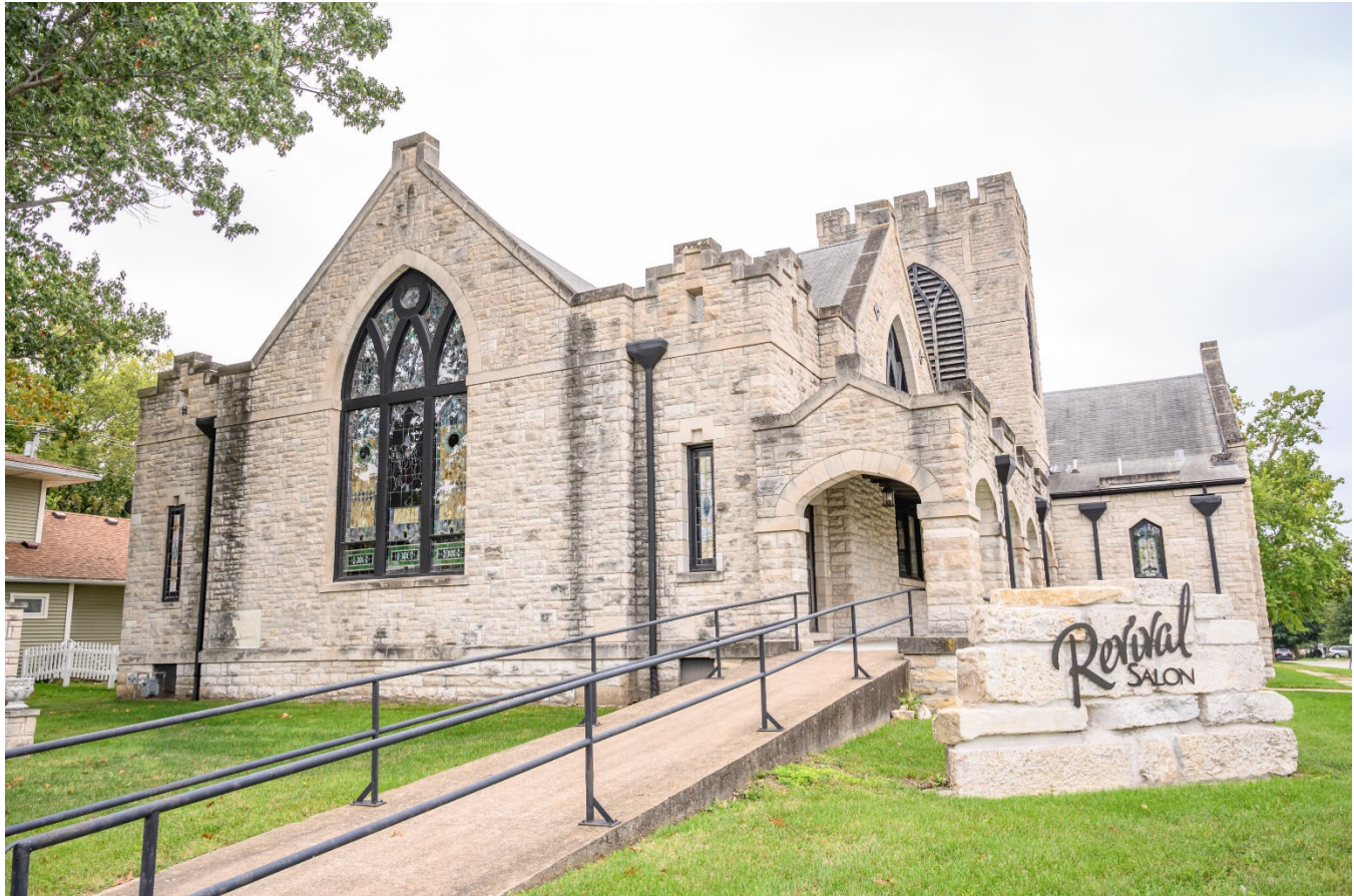
Photograph 44-02274-002. North elevation, looking southeast (October 2023)
