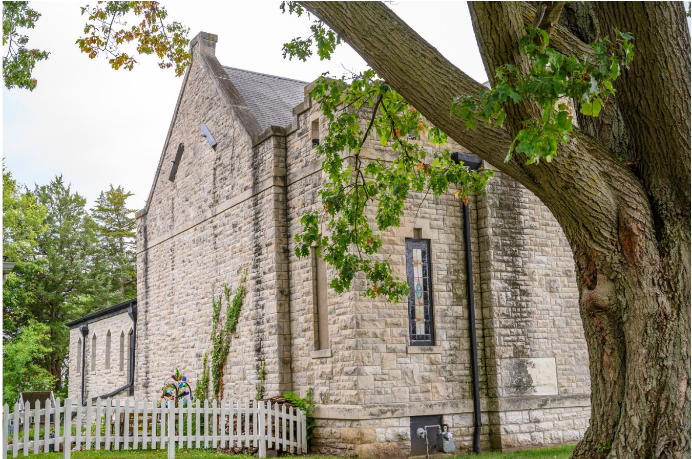
Photograph 44-02274-005. East elevation, looking southwest (October 2023)
