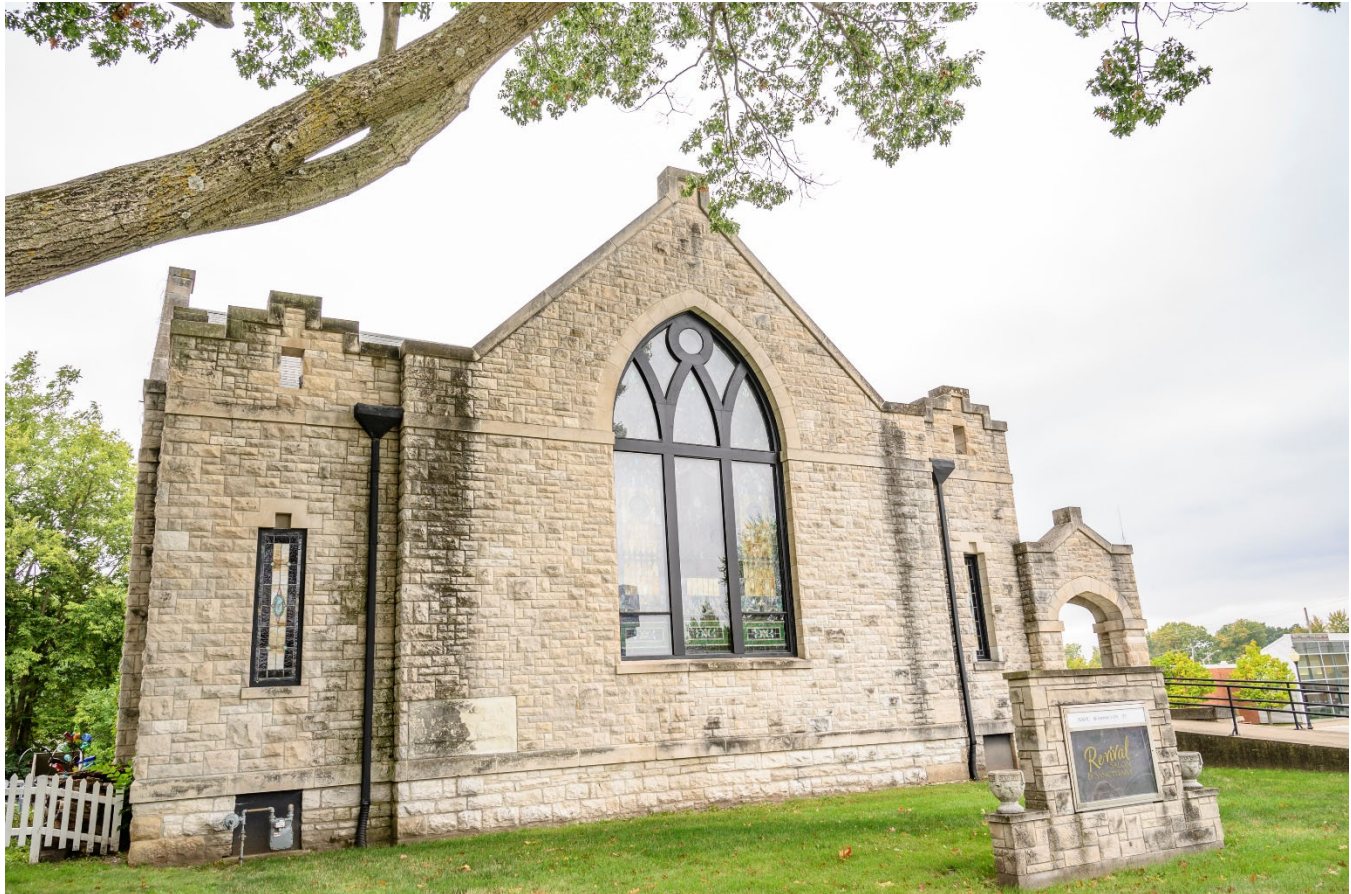
Photograph 44-02274-004. North elevation, looking south (October 2023)
