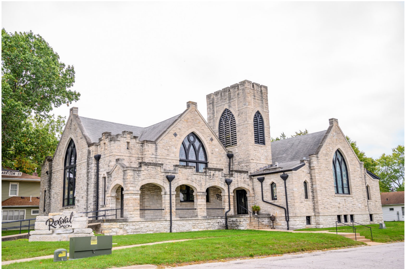
Photograph 44-02274-001. West elevation, looking southeast (October 2023)
