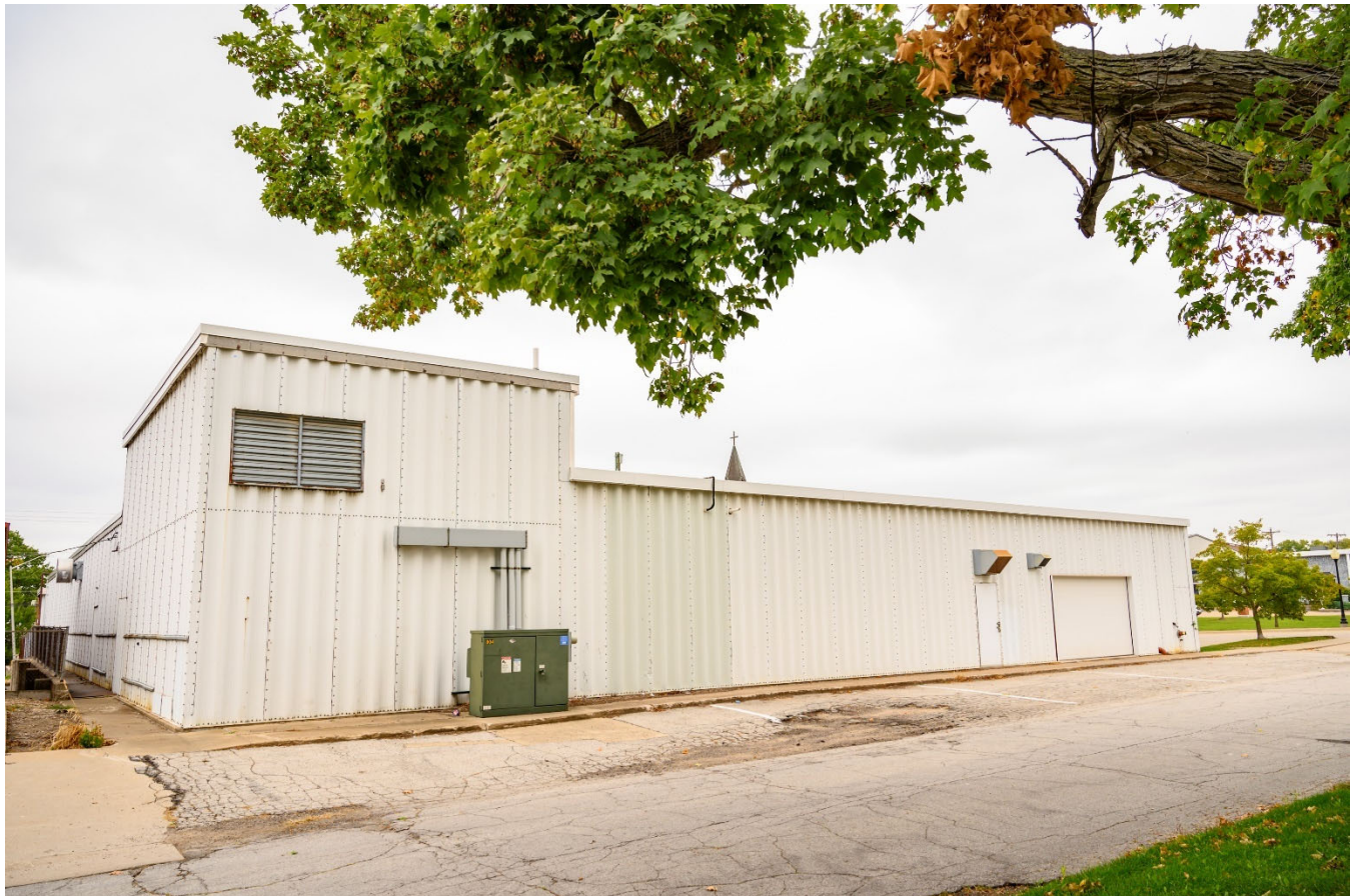
Photograph 44-02273-003. East elevation, looking west (October 2023)
