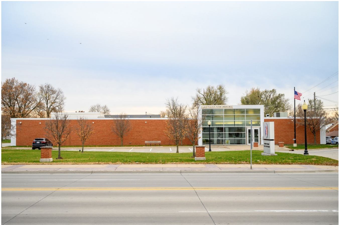
Photograph 44-02273-001. North elevation, looking south (October 2023)
