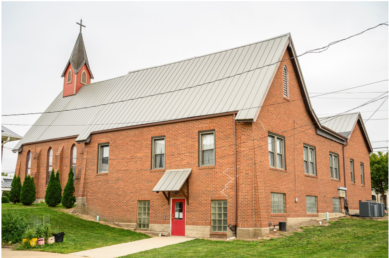
Photograph 44-02272-003. West and south elevations, looking northeast (October 2023)
