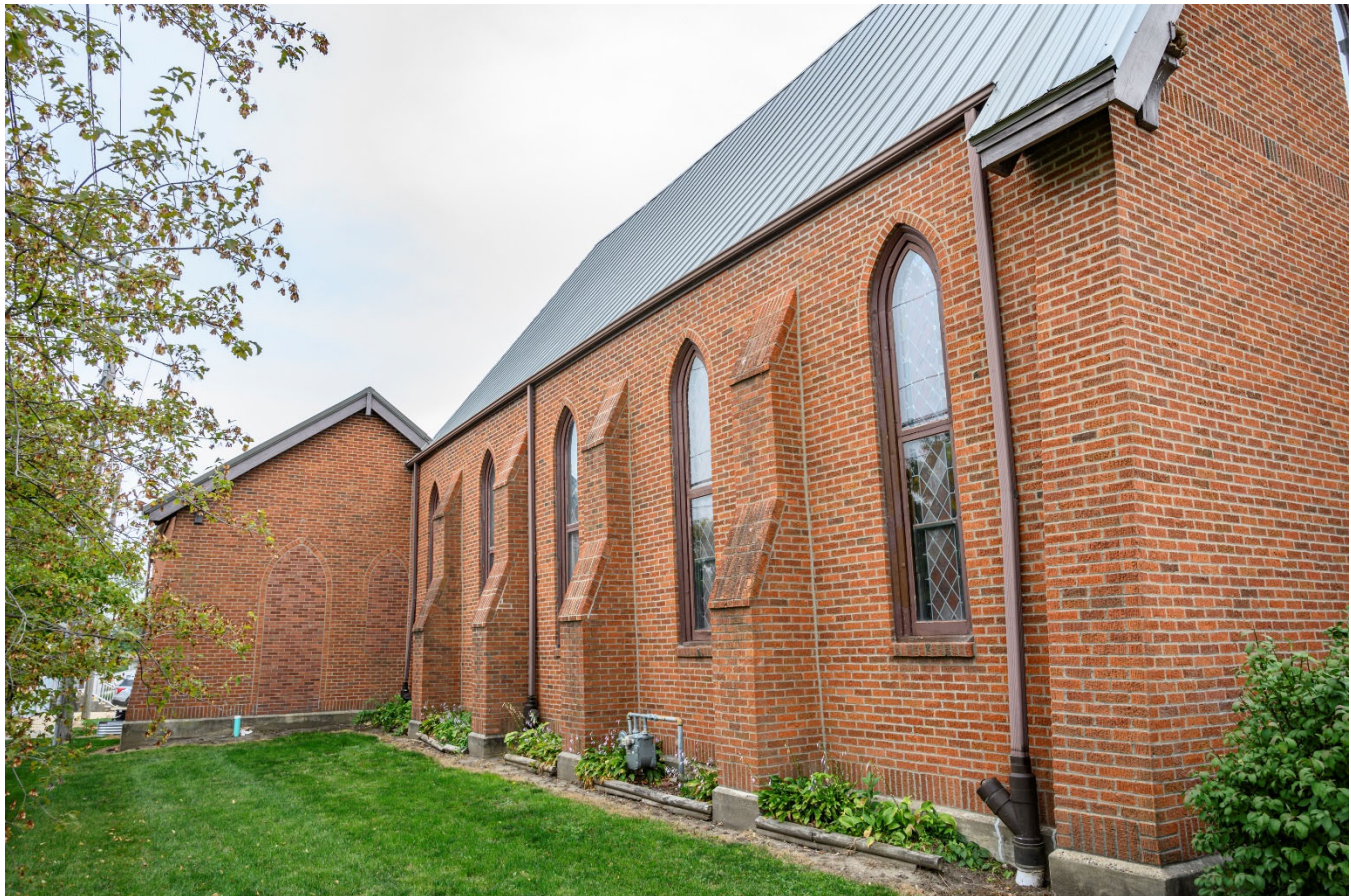
Photograph 44-02272-004. East elevation, looking southwest (October 2023)
