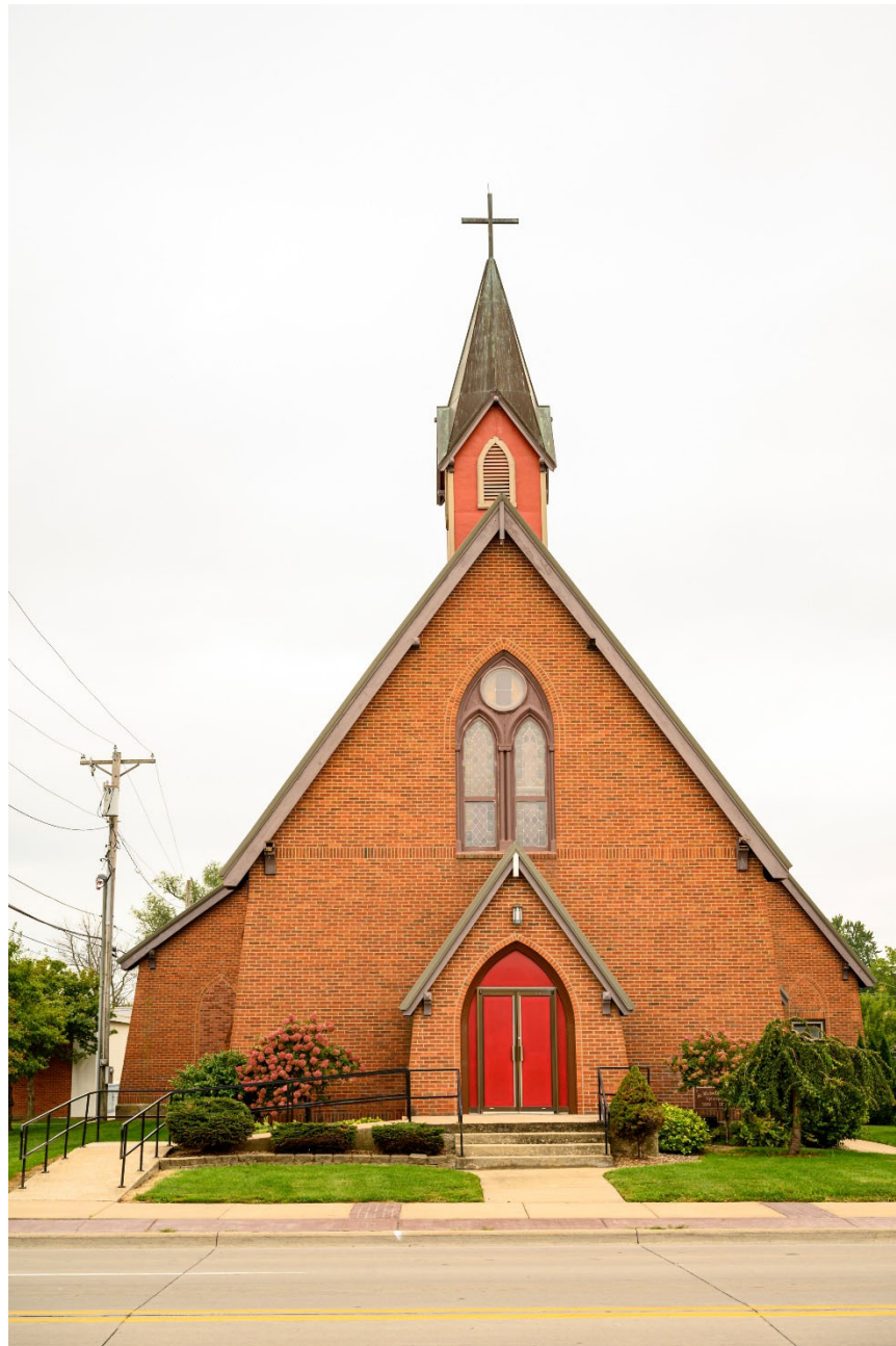
Photograph 44-02272-001. North elevation, looking south (October 2023)
