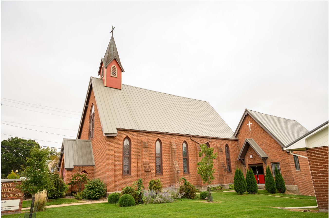
Photograph 44-02272-002. West elevation, looking east (October 2023)
