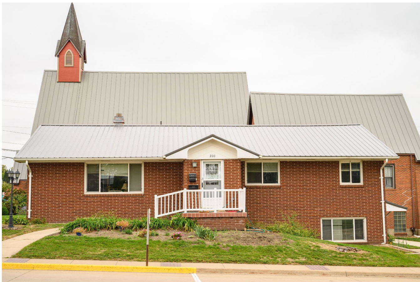
Photograph 44-02271-001. West elevation, looking east (October 2023)
