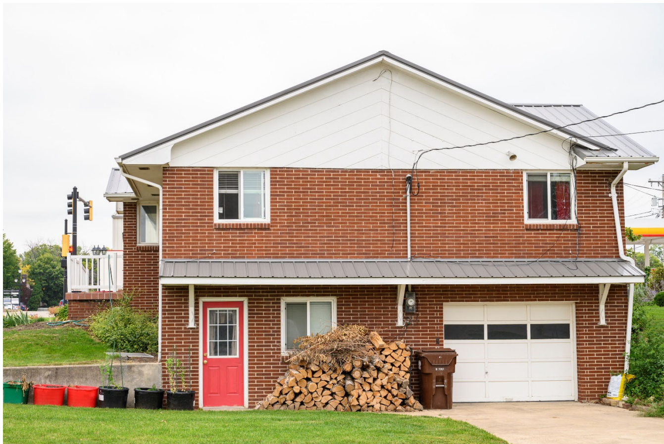
Photograph 44-02271-004. South elevation, looking north (October 2023)
