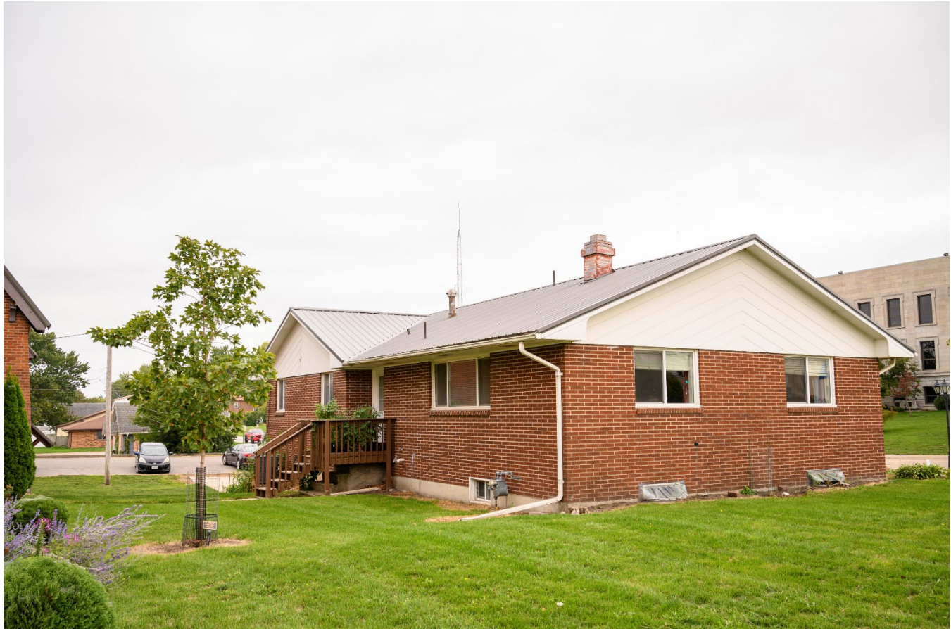
Photograph 44-02271-003. East and north elevations, looking southwest (October 2023)
