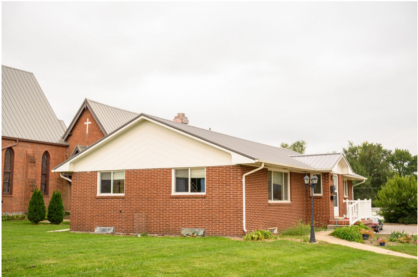
Photograph 44-02271-002. North elevation, looking southeast (October 2023)
