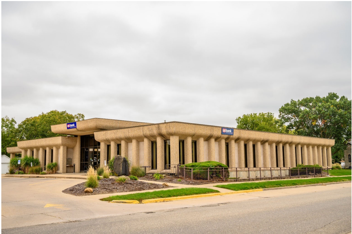
Photograph 44-02270-004. North and west elevations, looking southeast (October 2023)
