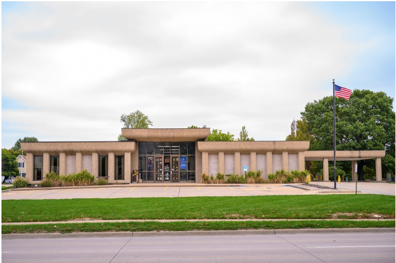
Photograph 44-02270-001. South elevation, looking north (October 2023)
