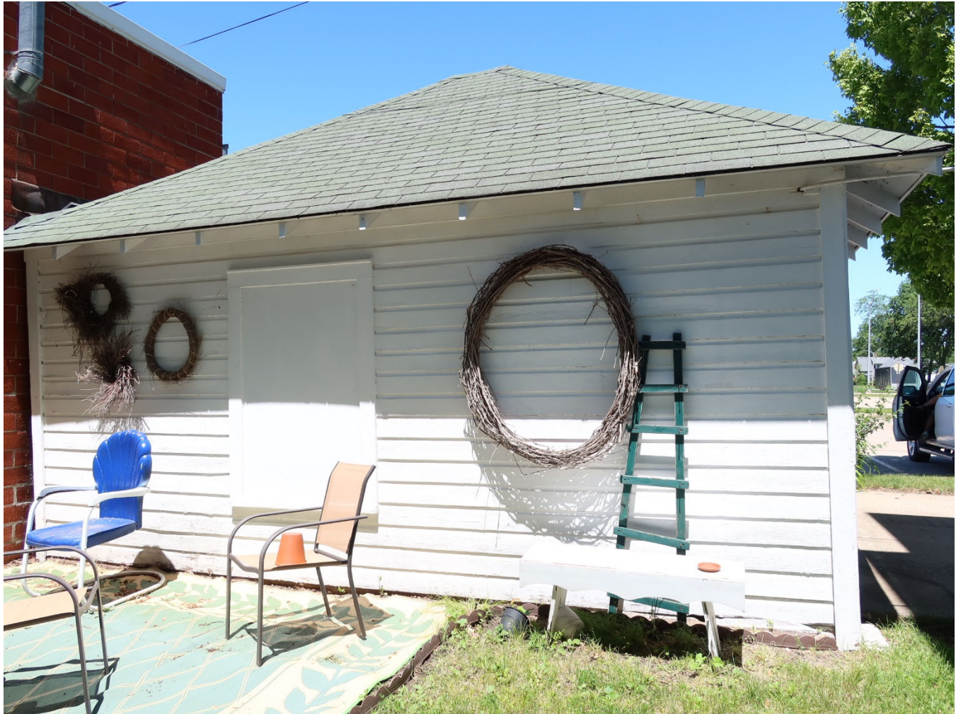
Photograph 44-02237-008. South elevation of garage, looking north (June 2024)
