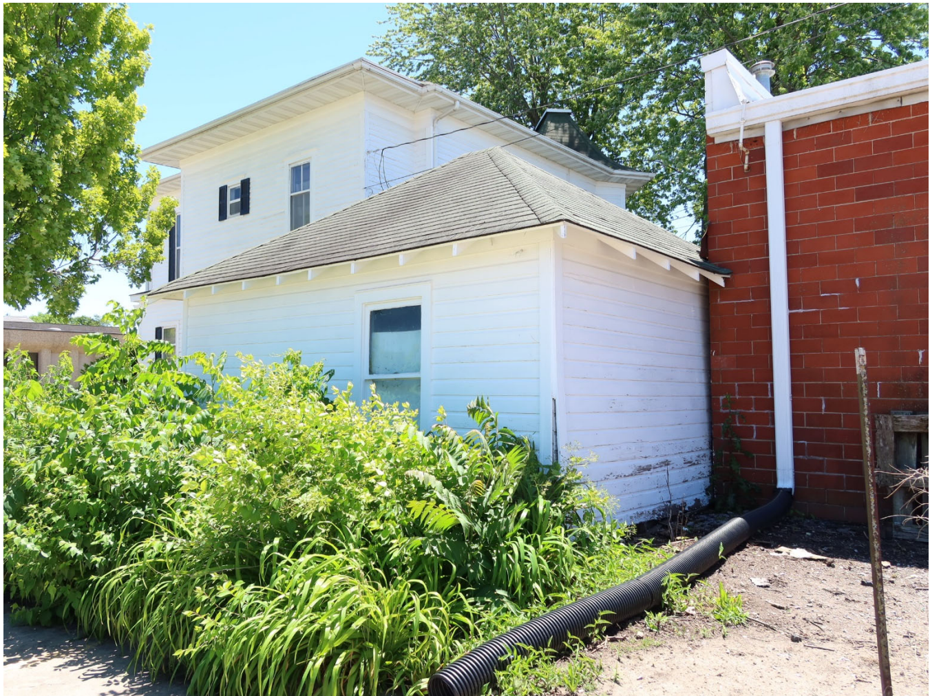
Photograph 44-02237-007. North and west elevations of garage, looking southeast (June 2024)
