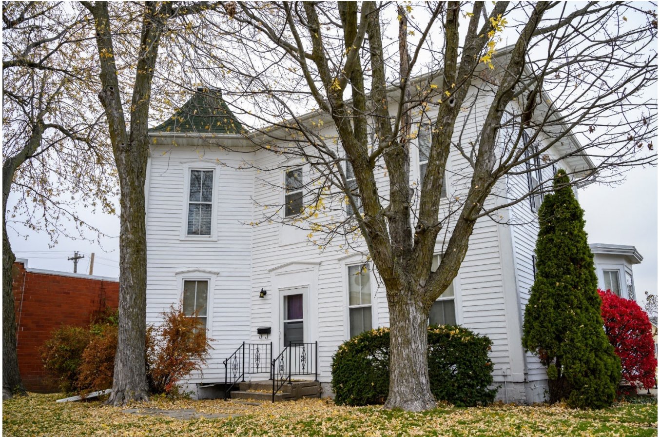
Photograph 44-02237-001. South elevation, looking northwest (October 2023)
