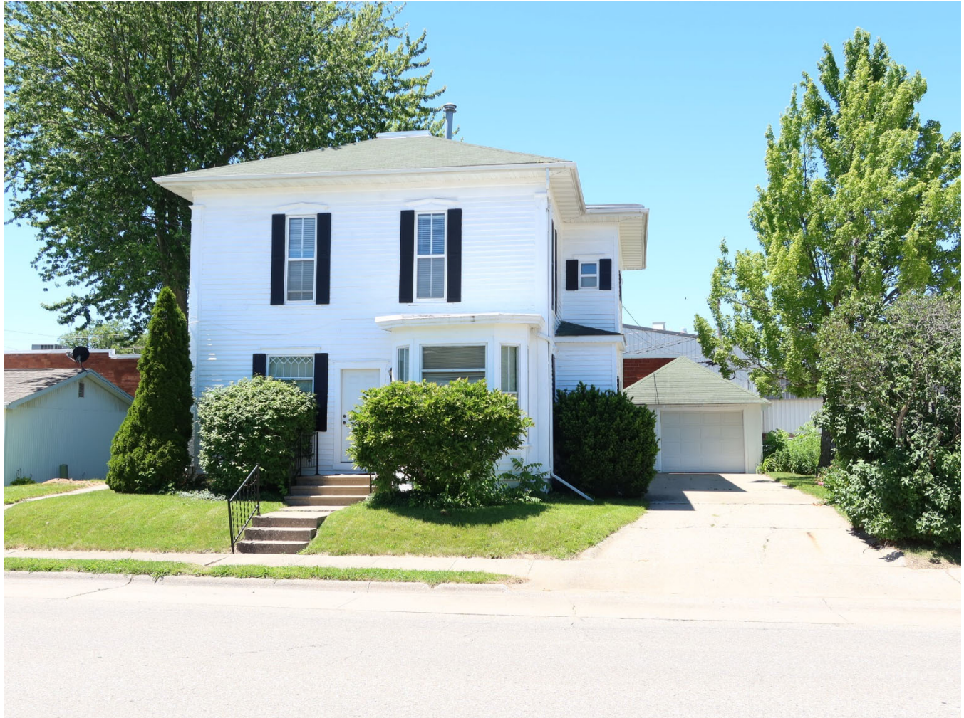
Photograph 44-02237-005. East elevation, looking west (June 2024)
