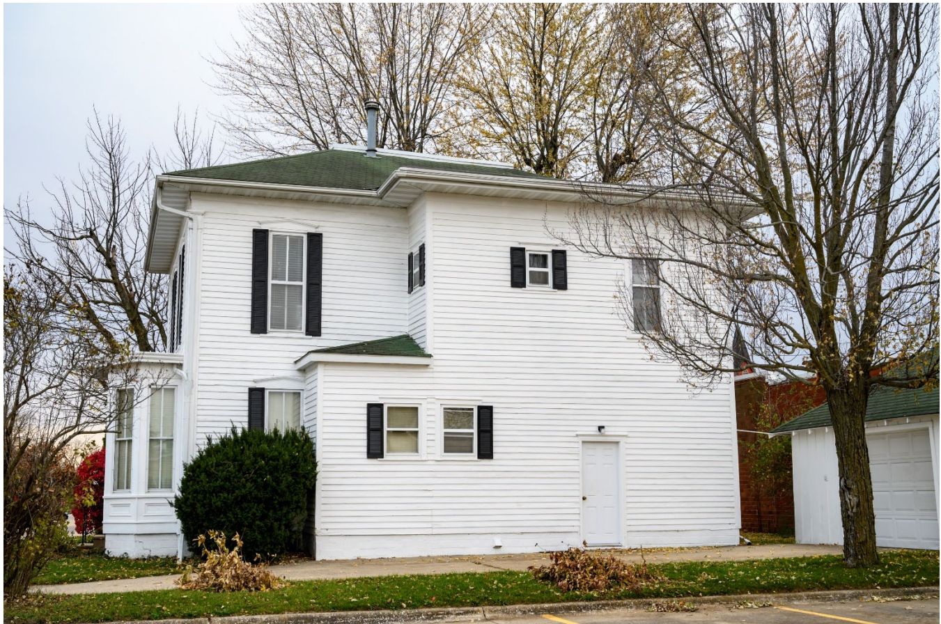
Photograph 44-02237-004. North elevation, looking south (October 2023)
