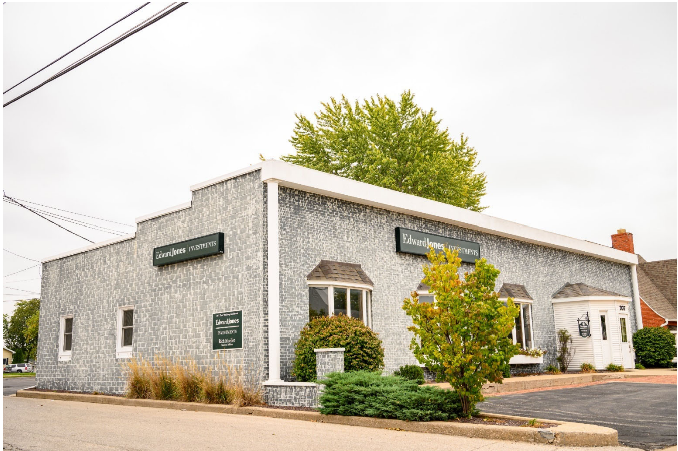
Photograph 44-02268-001. West and south elevations, looking northeast (October 2023)
