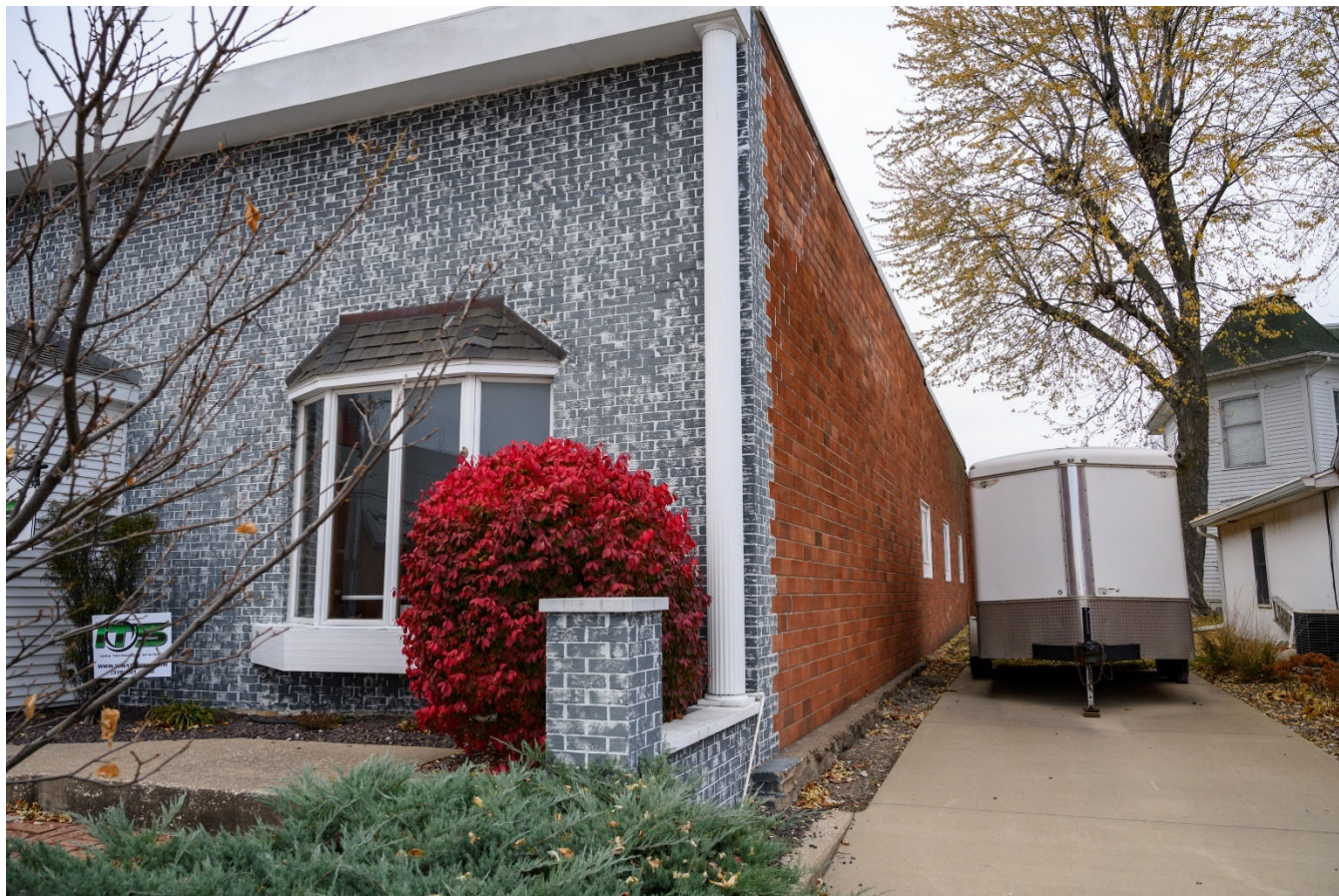
Photograph 44-02268-003. East elevation, looking northeast (October 2023)
