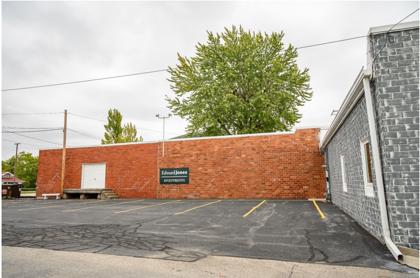
Photograph 44-02268-004. West elevation of rear section, looking east (October 2023)
