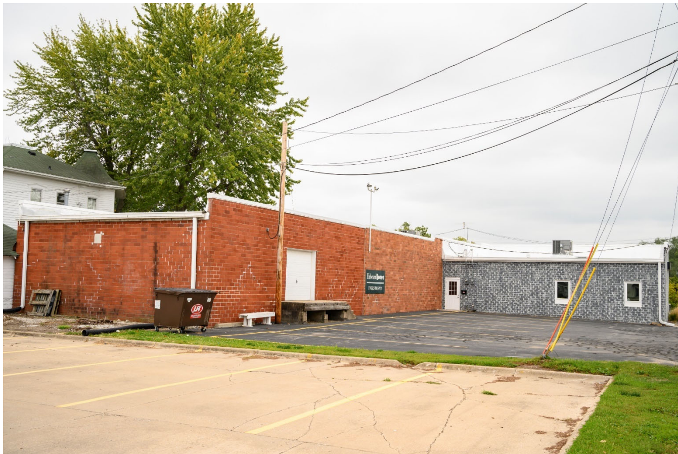
Photograph 44-02268-005. North and east elevations, looking southeast (October 2023)
