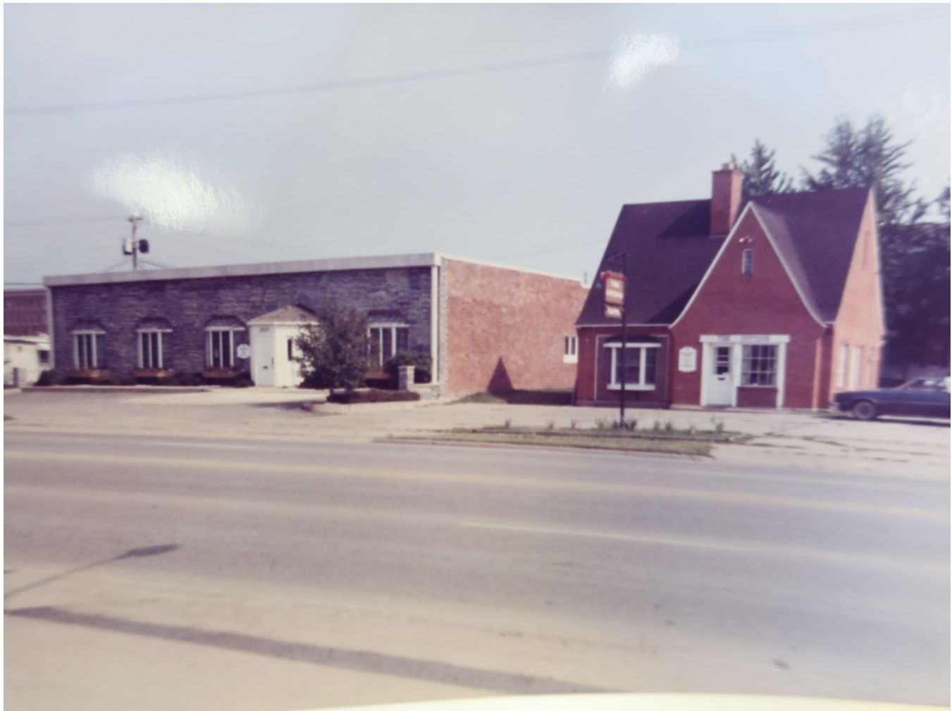
Building in the 1980s (City of Mt Pleasant building permits)
