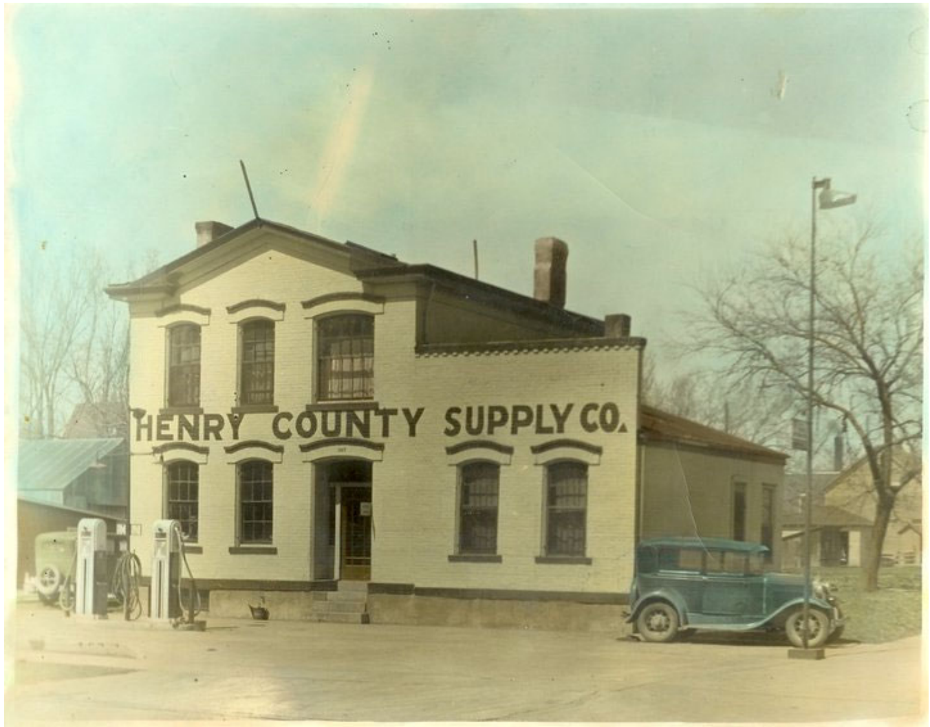
Earlier building of Henry County Supply Co
