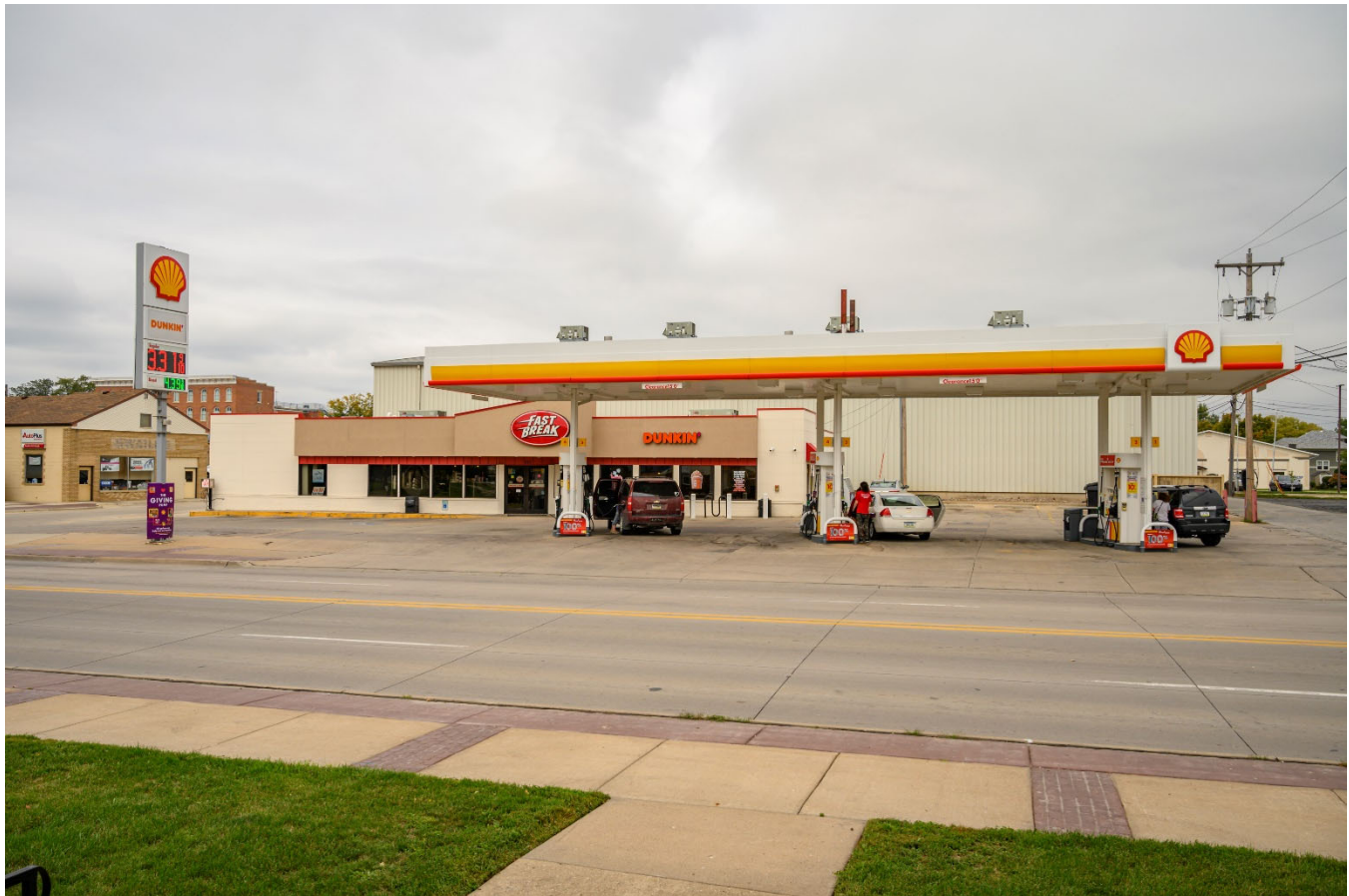
Photograph 44-02267-001. South elevation, looking north (October 2023)
