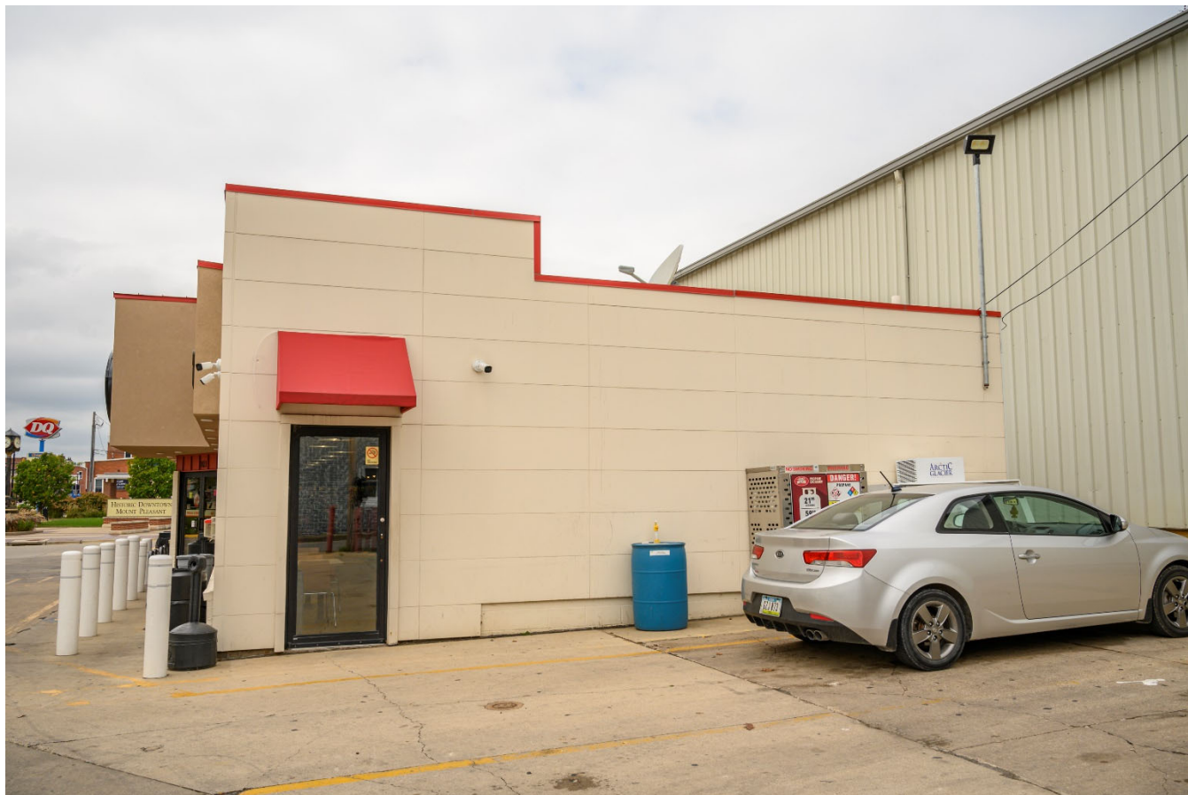
Photograph 44-02267-003. East elevation, looking west (October 2023)
