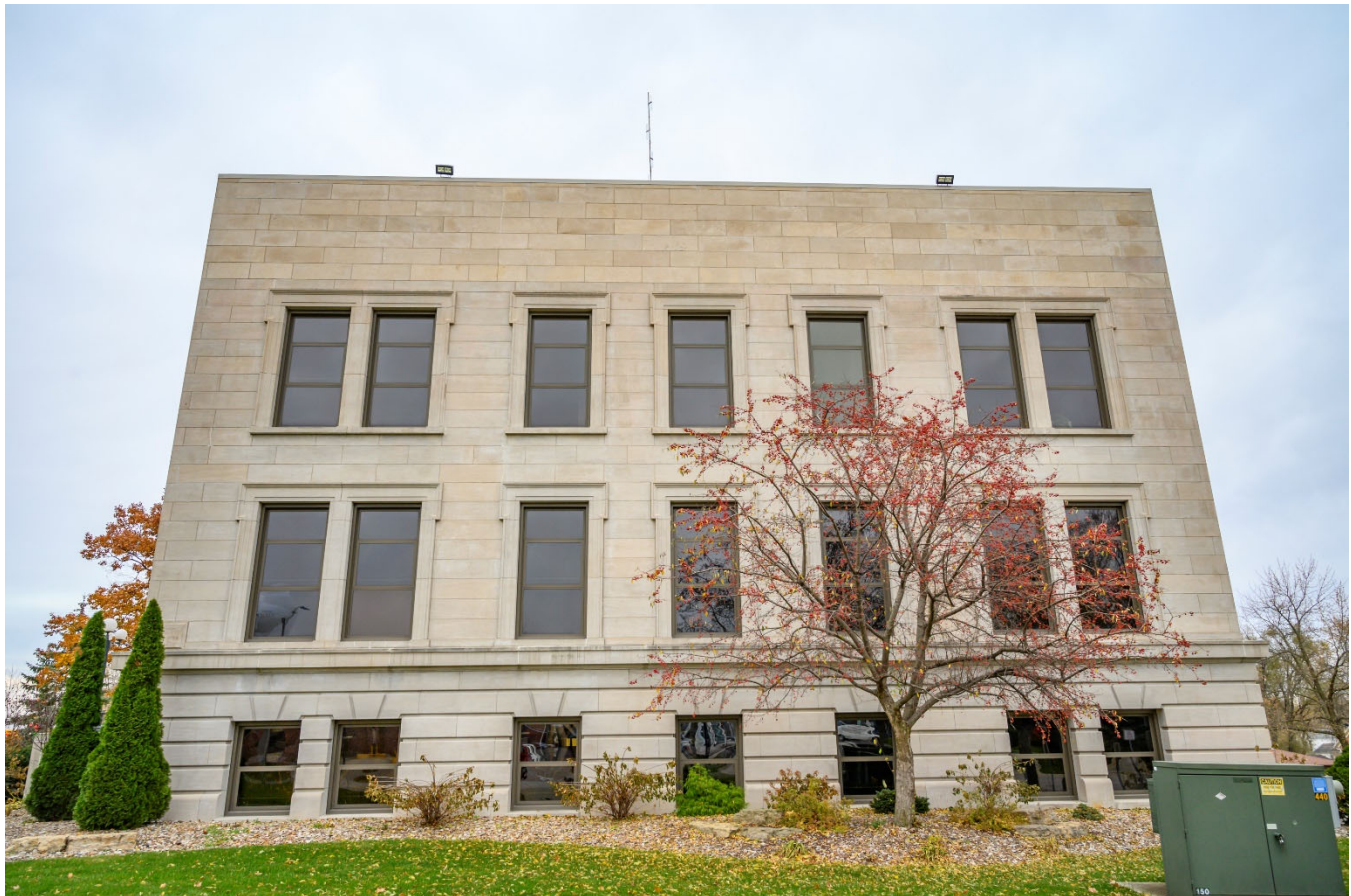
Photograph 44-00442-004. West elevation, looking east (October 2023)
