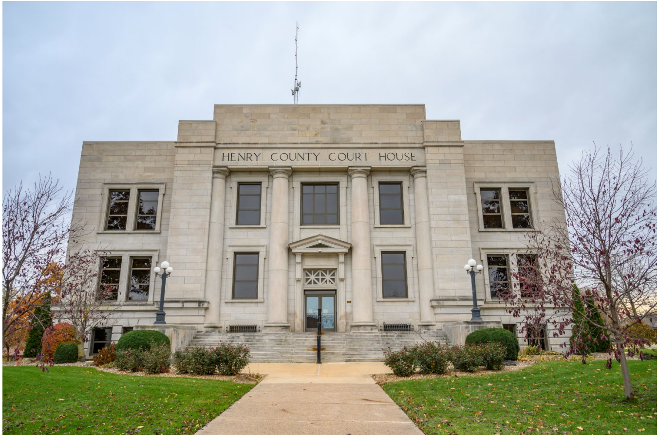
Photograph 44-00442-002. North elevation, looking south (October 2023)
