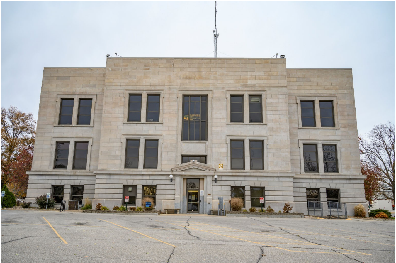
Photograph 44-00442-005. South elevation, looking north (October 2023)
