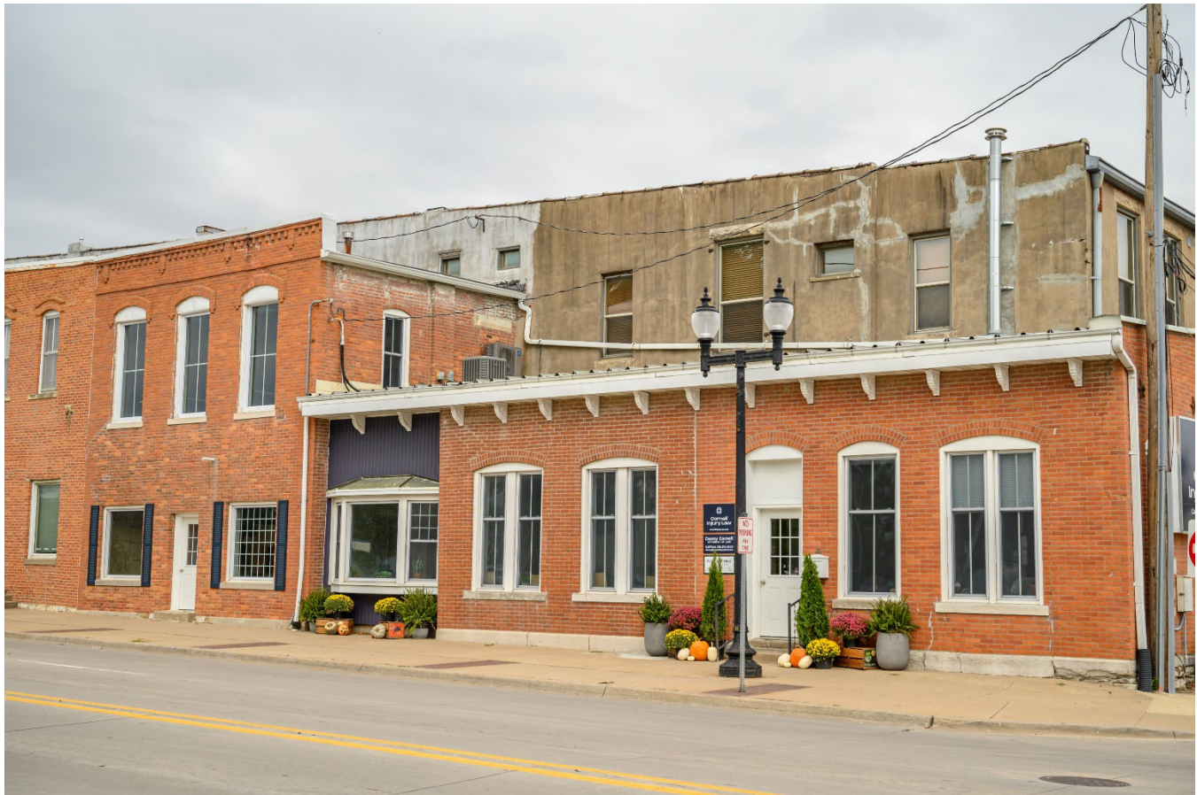
Photograph 44-00414-001. South elevation, looking northwest (October 2023)
