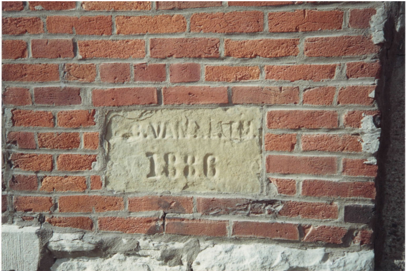
Photograph 44-00414-003. Corner stone on east elevation, looking west (October 2023)
