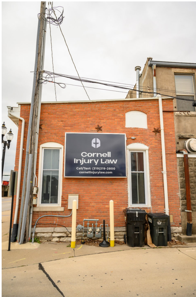
Photograph 44-00414-002. East elevation, looking west (October 2023)
