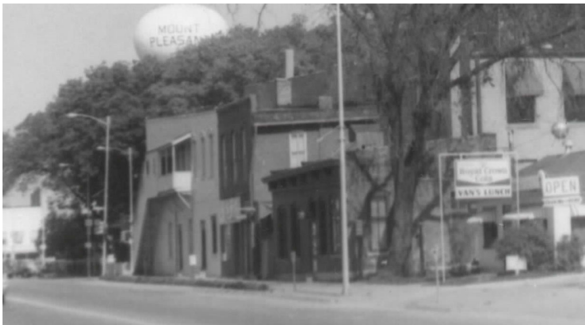
Side/rear of building in July 1965, looking northwest from Washington St (HCHT collection)
