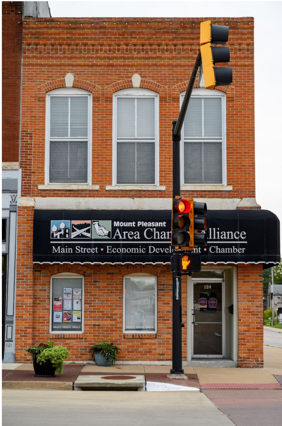
Photograph 44-00302-001. West elevation, looking east (October 2023)
