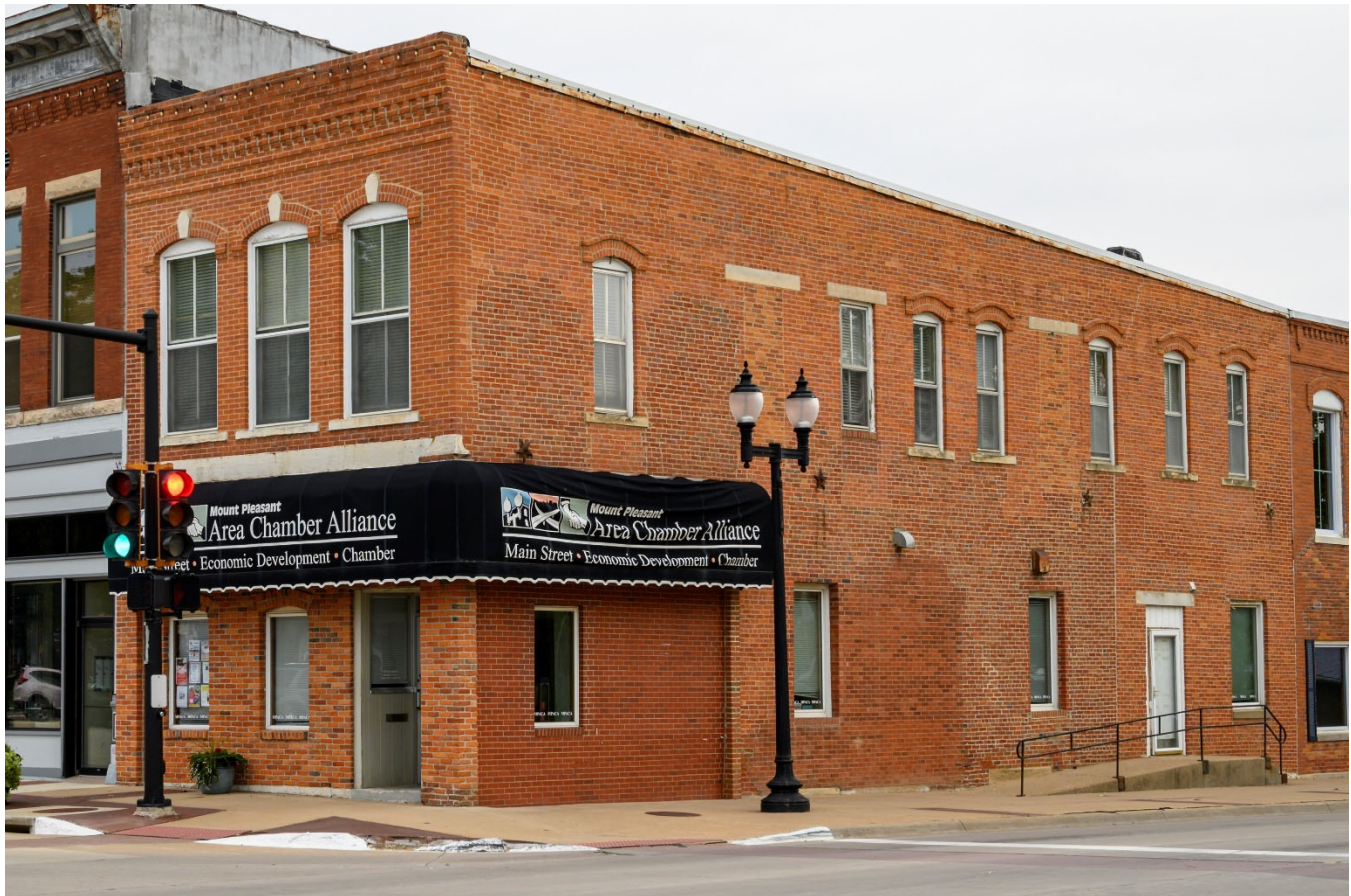
Photograph 44-00302-002. West and south elevations, looking northeast (October 2023)
