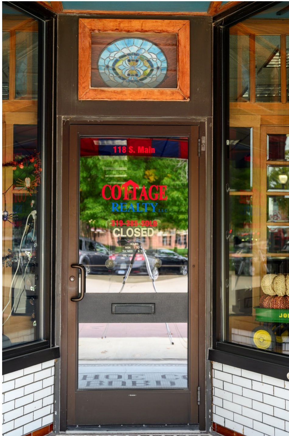
Photograph 44-00300-002. Detail of entry on west elevation, looking east (October 2023)
