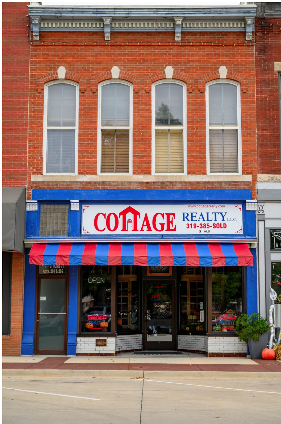
Photograph 44-00300-001. West elevation, looking east (October 2023)
