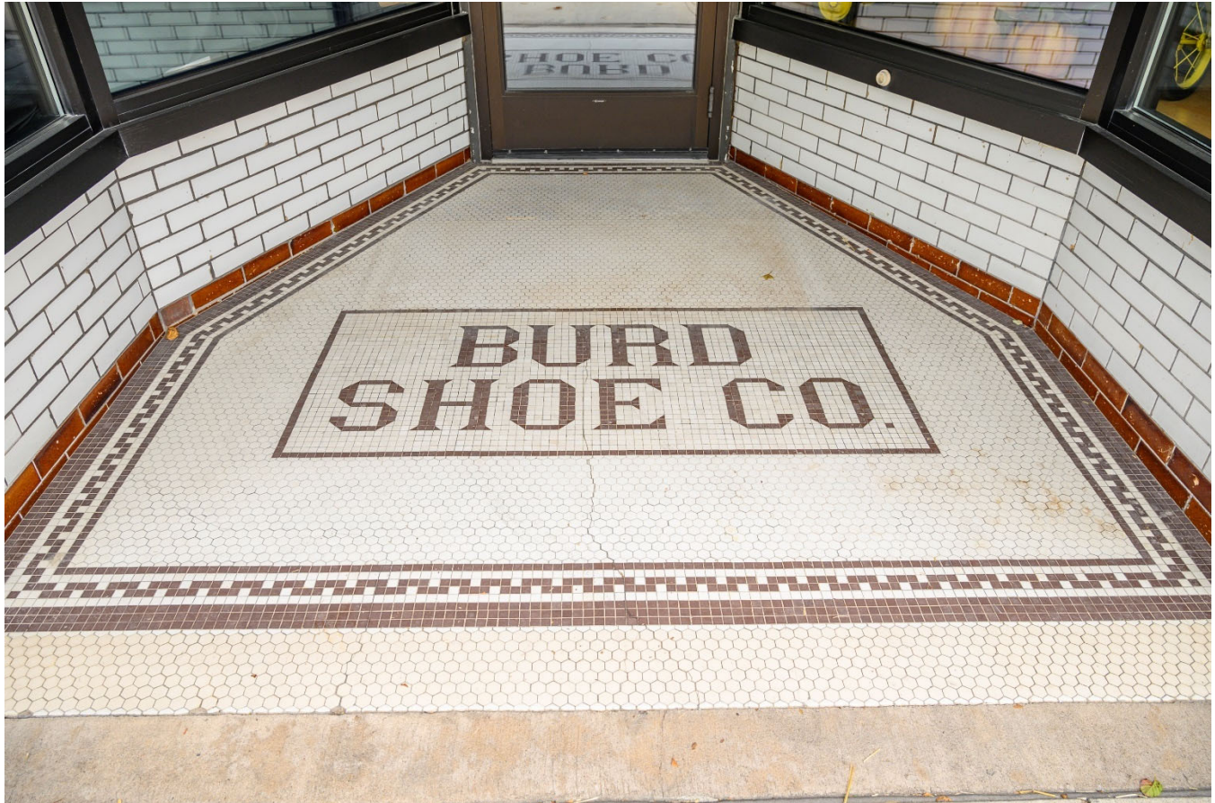
Photograph 44-00300-003. Detail of entry tile on west elevation, looking east (October 2023)
