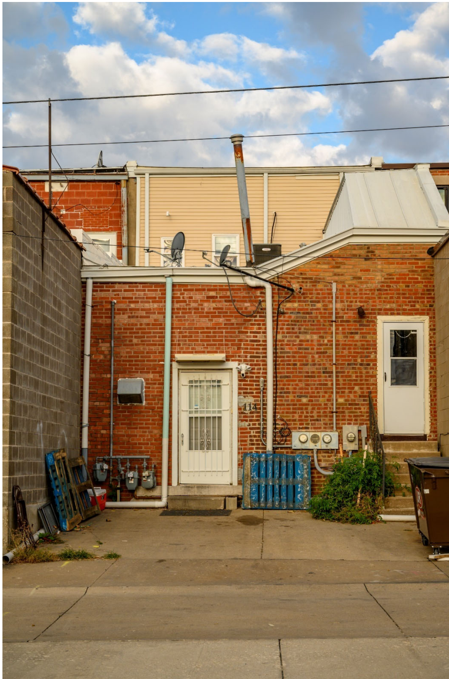
Photograph 44-00298-002. East elevation, looking west (October 2023)
