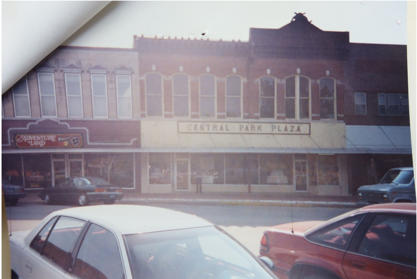
Building in 1994 (City of Mt Pleasant building permits)
