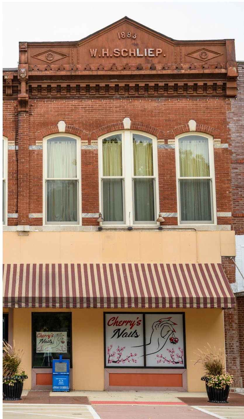
Photograph 44-00297-003. West elevation of 112 section, looking east (October 2023)
