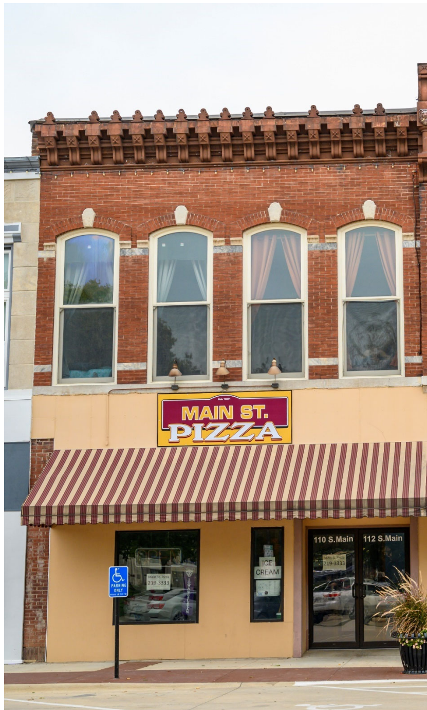
Photograph 44-00297-002. West elevation of 110 section, looking east (October 2023)
