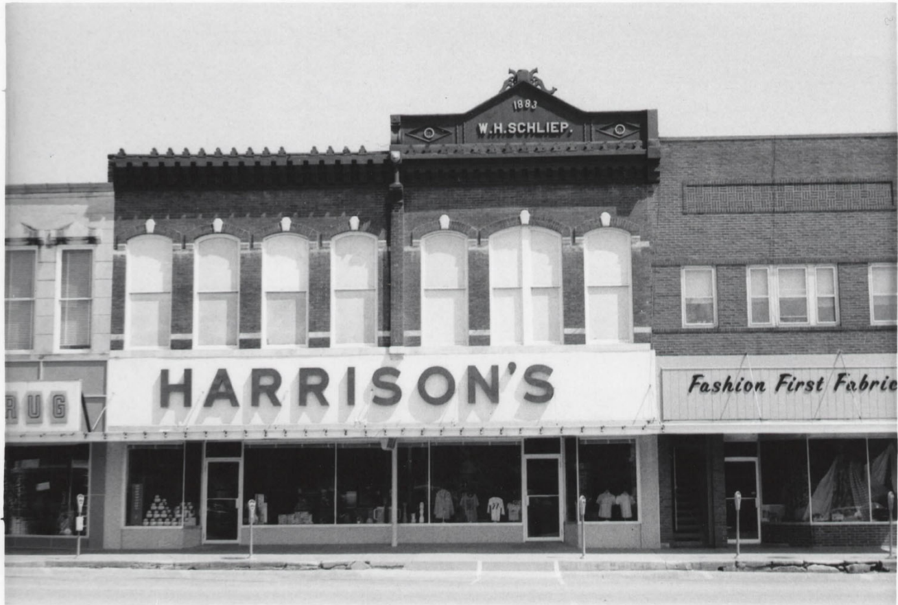
Building in early 1970s (HCHT files)
