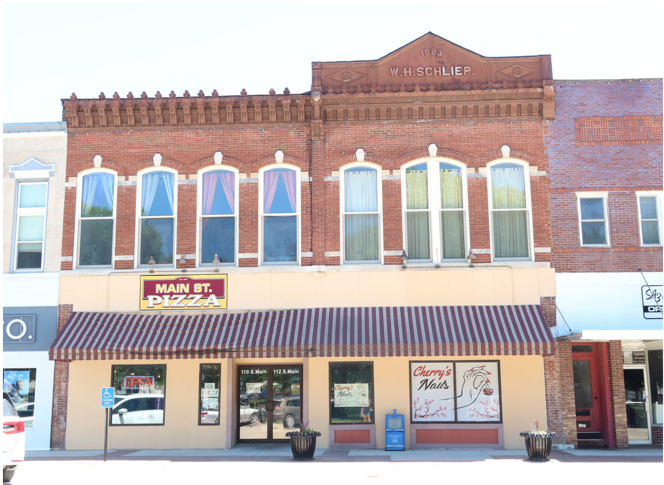
Photograph 44-00297-001. West elevation, looking east (June 2024)
