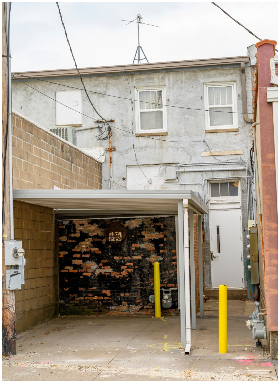
Photograph 44-00296-002. East elevation, looking west (October 2023)
