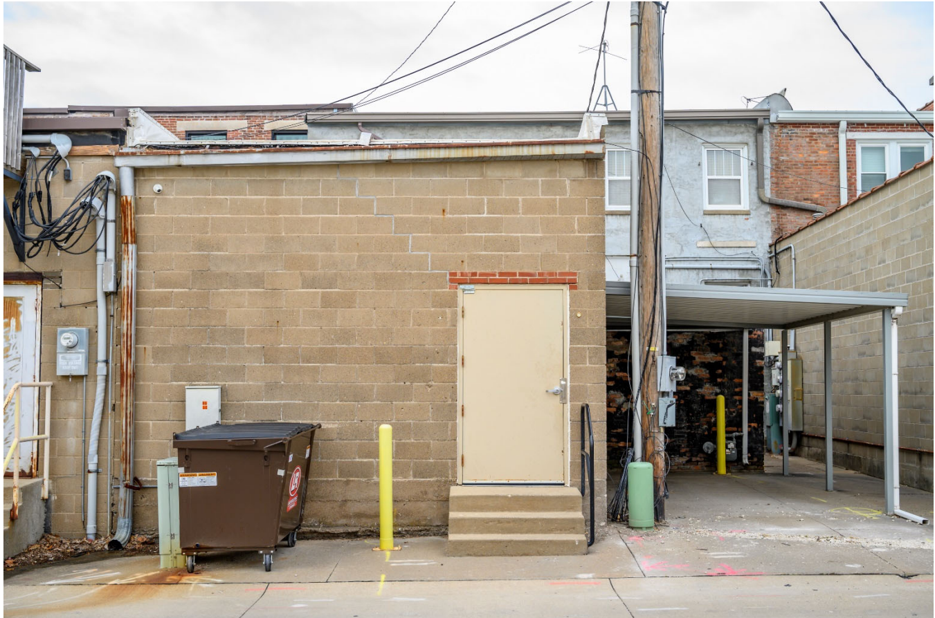
Photograph 44-00296-003. East elevation, looking west (October 2023)
