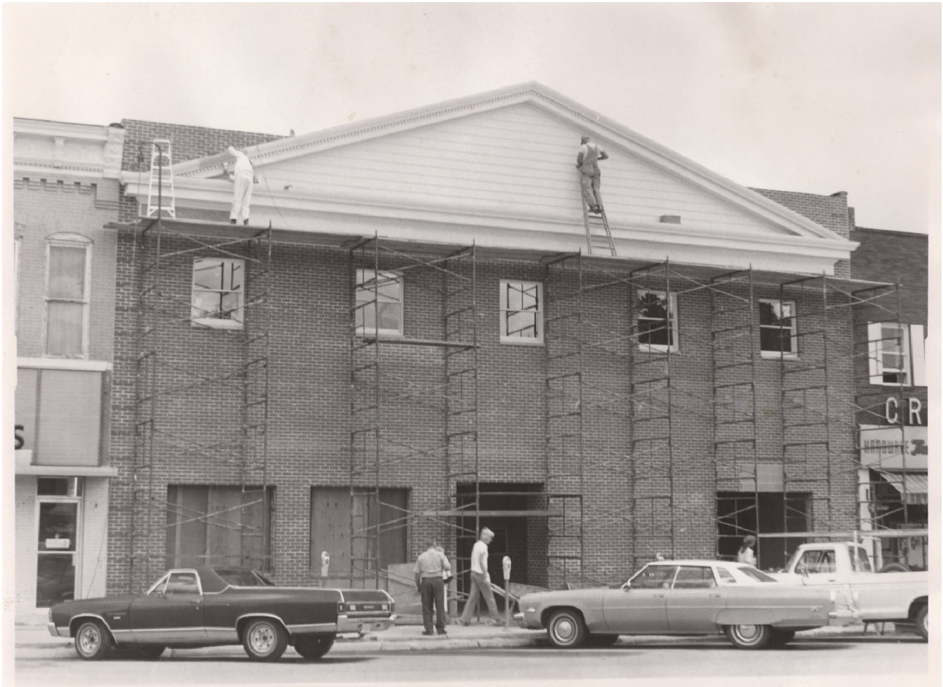
Bank façade remodel in progress on July 19, 1975 (HCHT files)
