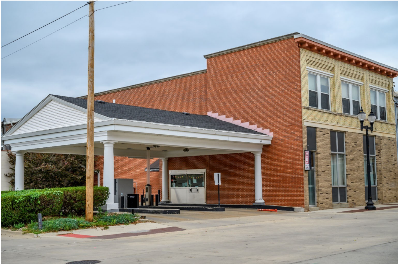
Photograph 44-00294-002. East and north elevations, looking southwest (October 2023)
