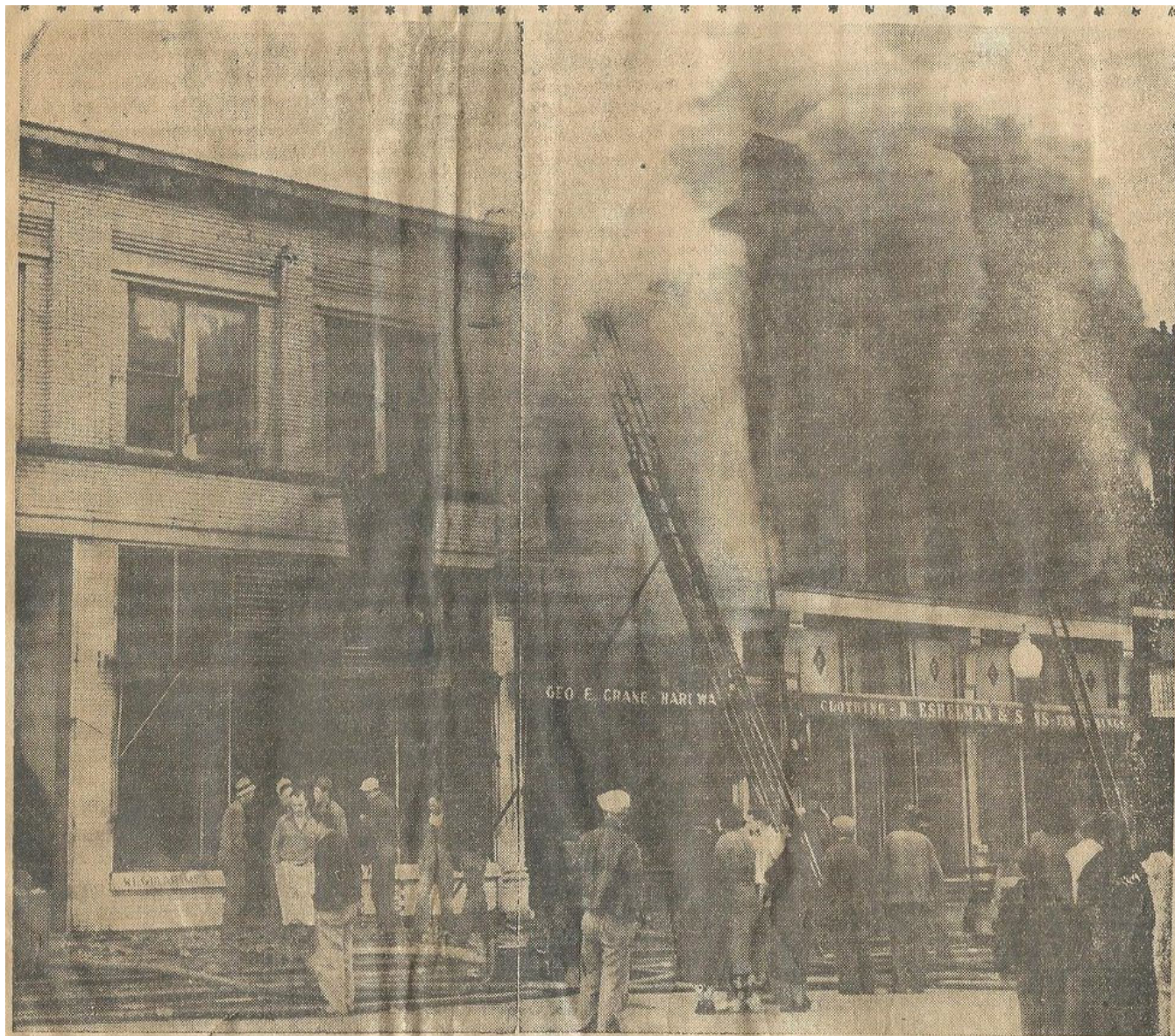
Fire on the east side of the square started in the Hi-Hat Café at the left and then spread to the Crane building to its south and to the Eshelman building ( Mt Pleasant News , June 10, 1938, 1; HCHT clipping)
