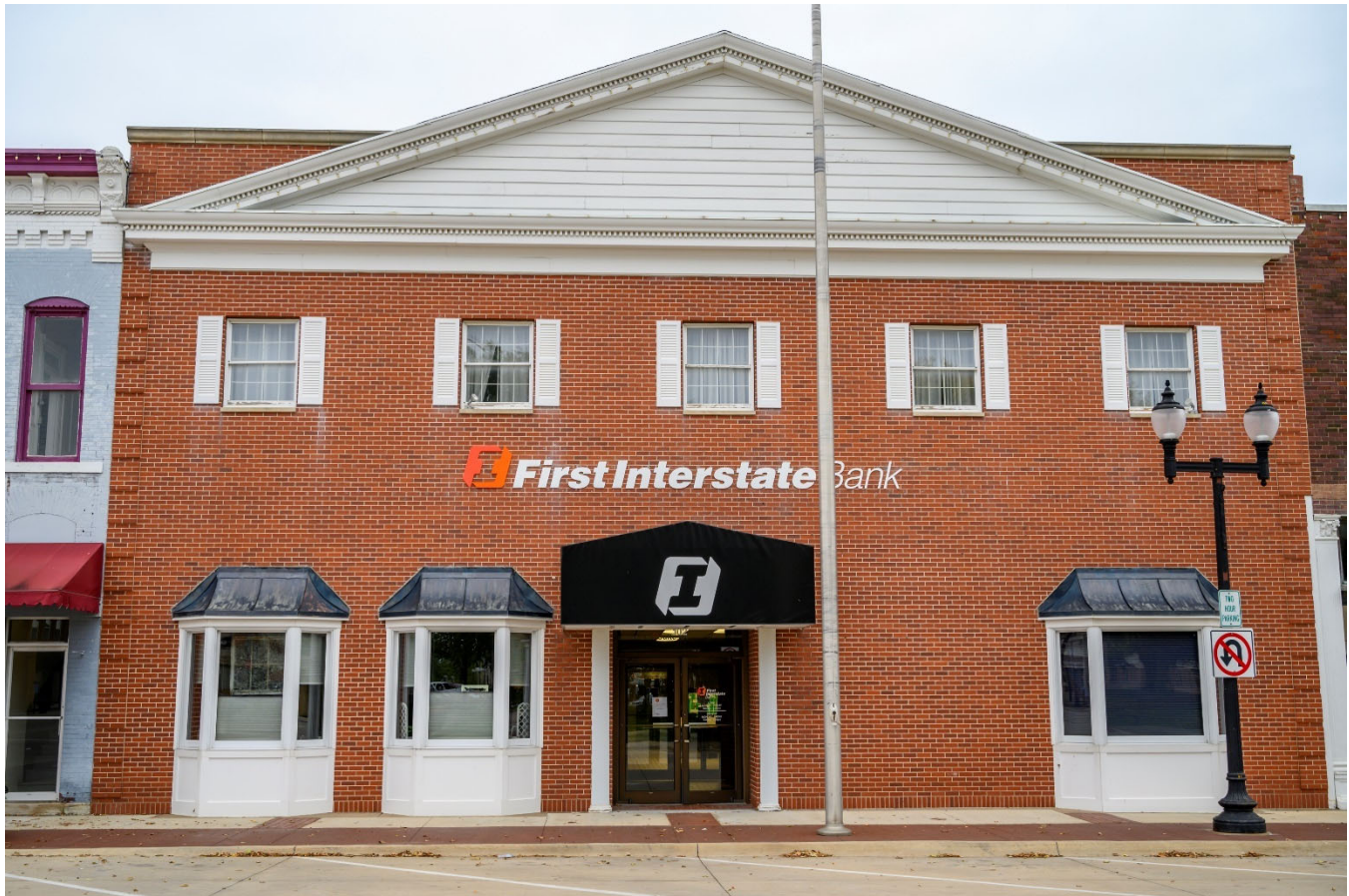
Photograph 44-00294-001. West elevation, looking east (October 2023)
