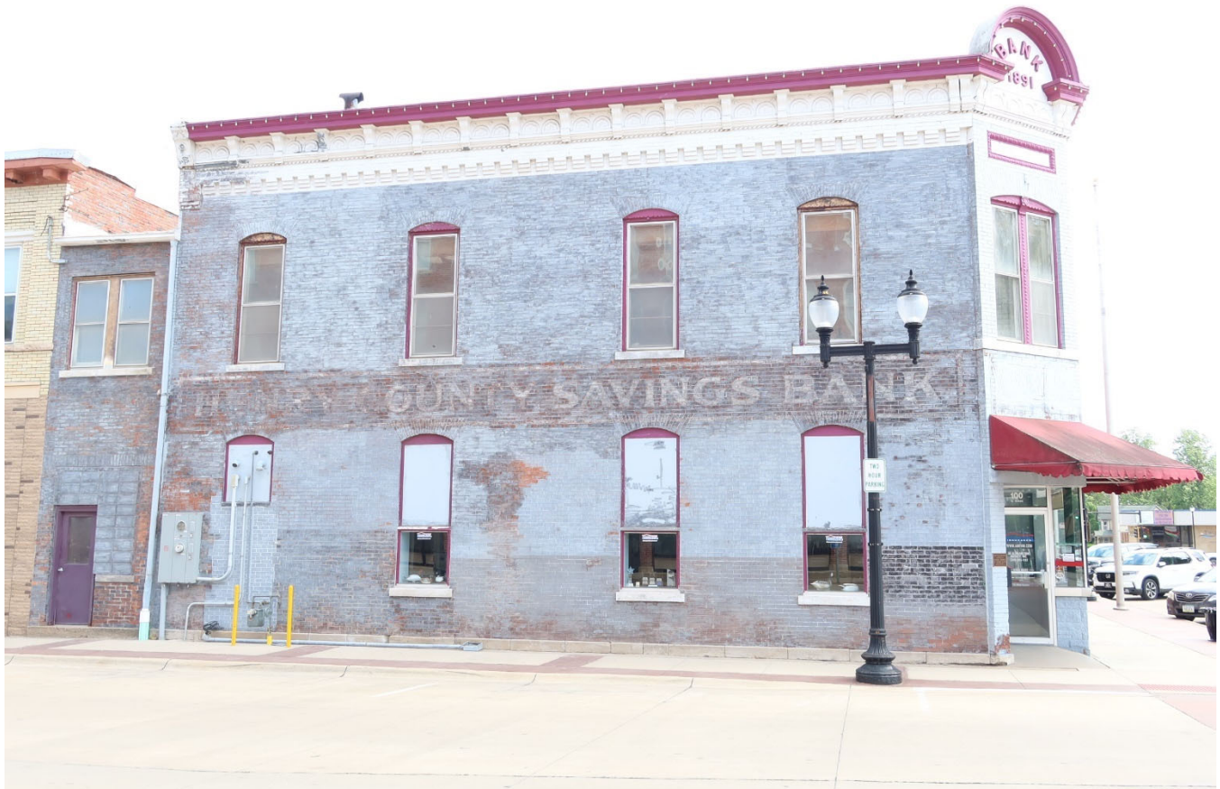
Photograph 44-00293-003. North elevation in June 2024 with paint removal underway and old sign visible, looking south (June 2024)
