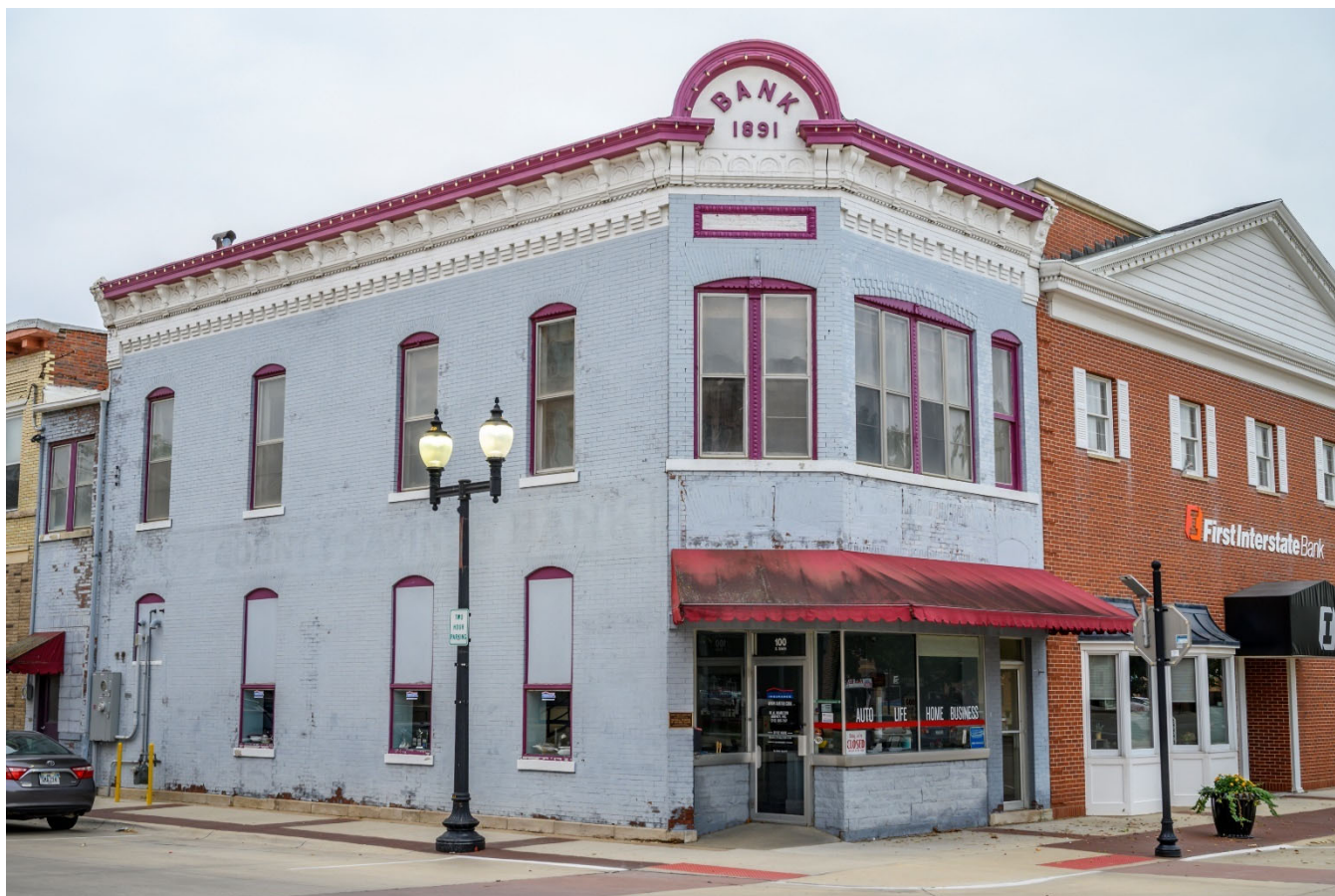
Photograph 44-00293-001. North and west elevations, looking southeast (October 2023)
