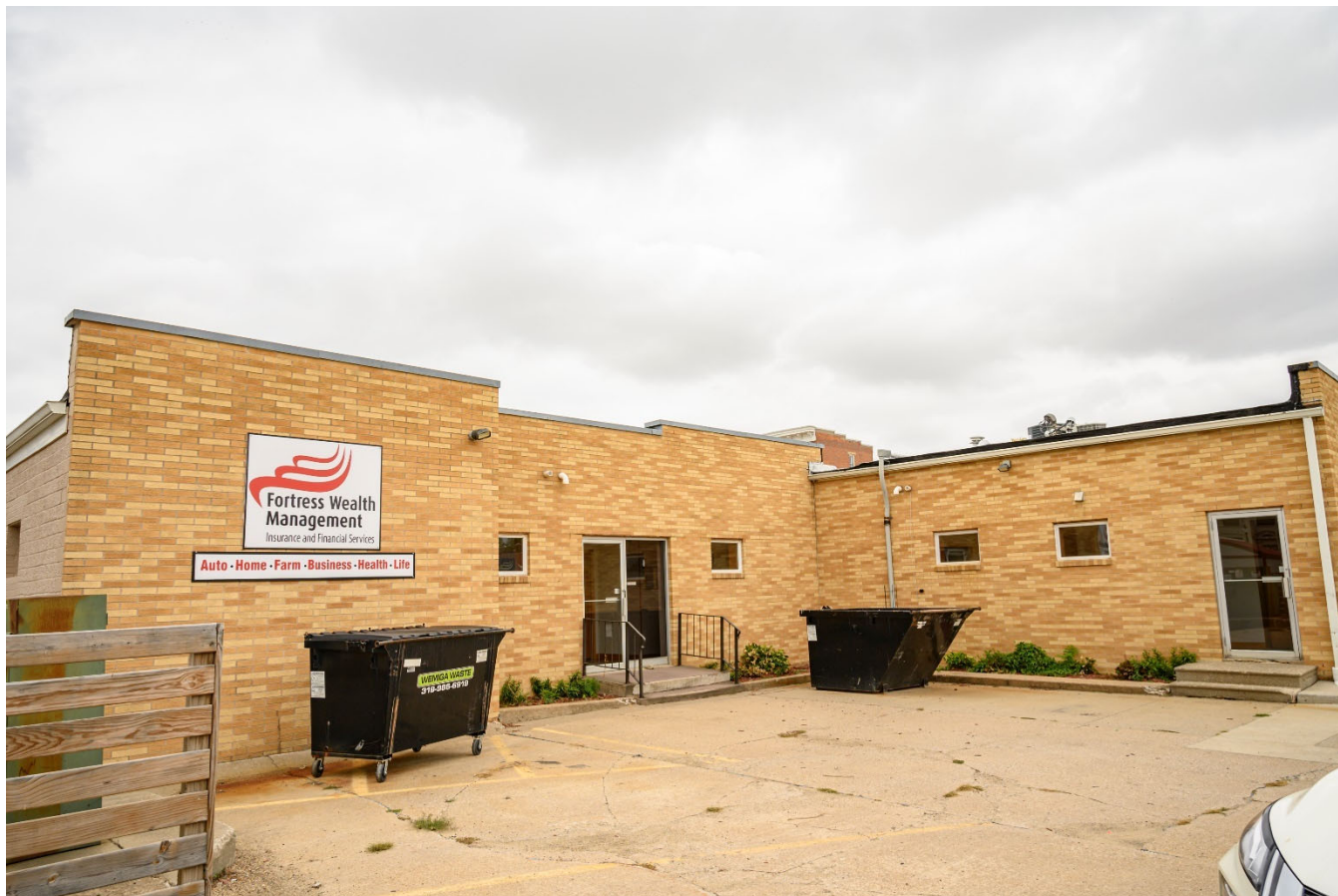
Photograph 44-00330-005. South elevation, looking northwest (October 2023)
