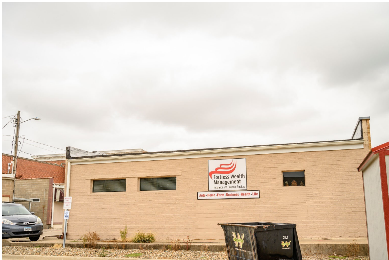
Photograph 44-00330-004. South elevation, looking north (October 2023)
