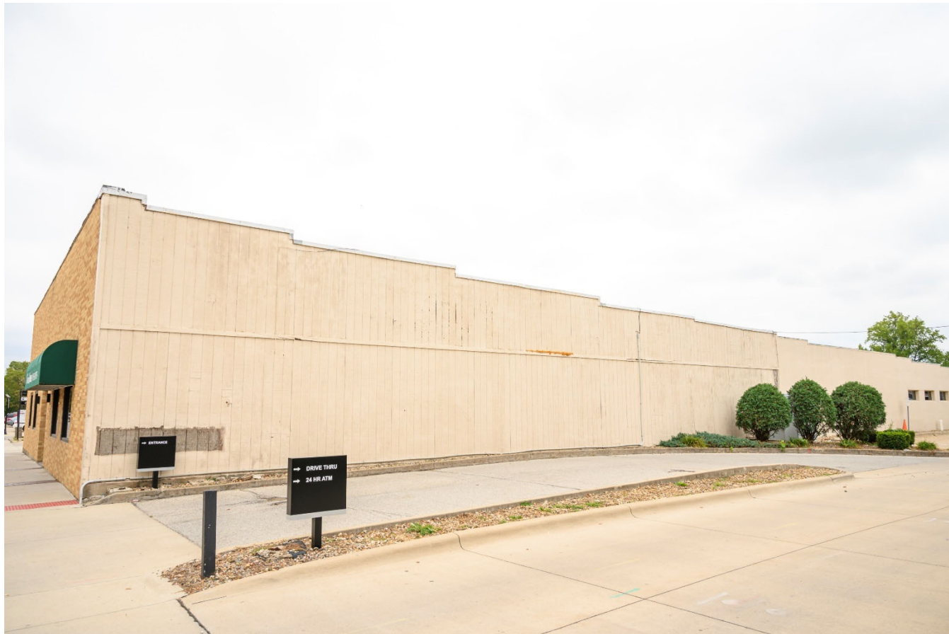
Photograph 44-00330-003. West elevation, looking east (October 2023)
