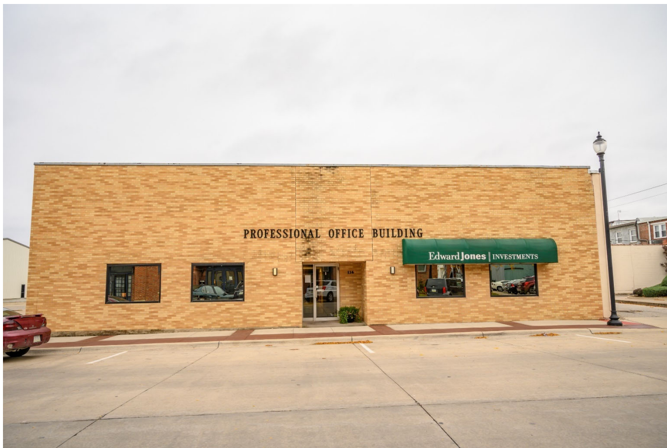
Photograph 44-00330-001. North elevation, looking south (October 2023)
