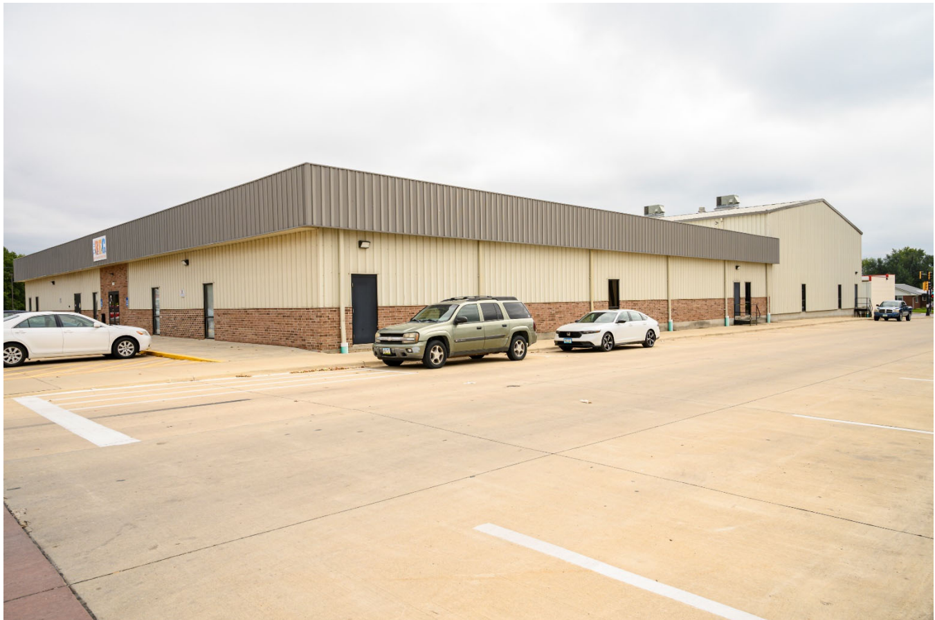
Photograph 44-02262-002. North and west elevations, looking southeast (October 2023)
