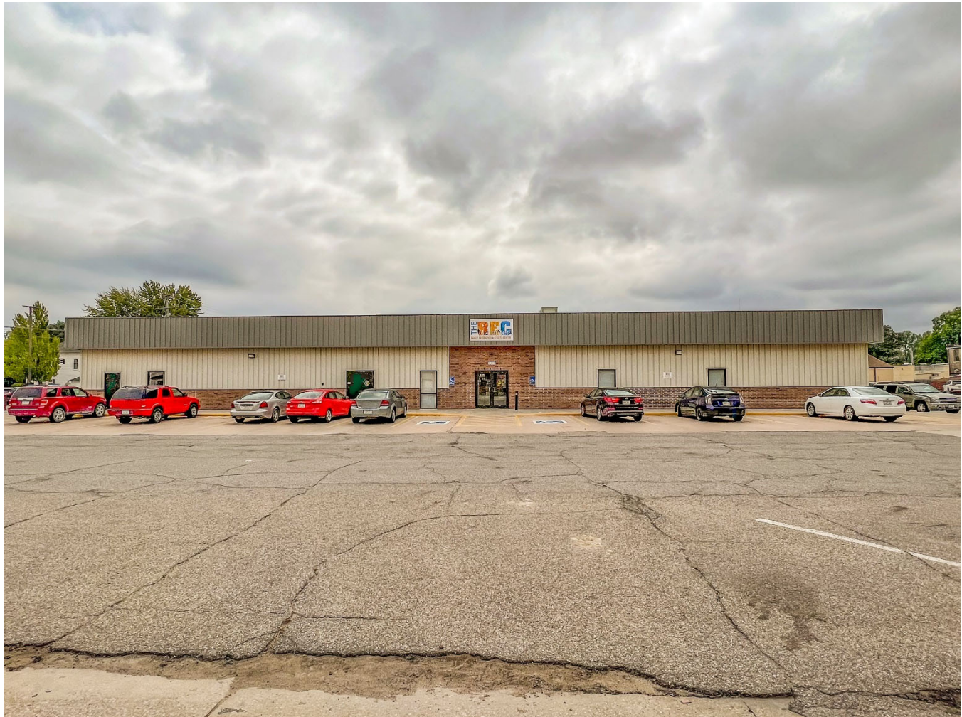
Photograph 44-02262-001. North elevation, looking south (October 2023)
