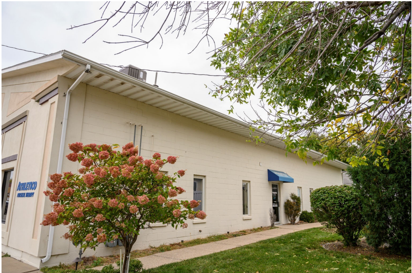
Photograph 44-002261-003. East elevation, looking northwest (October 2023)
