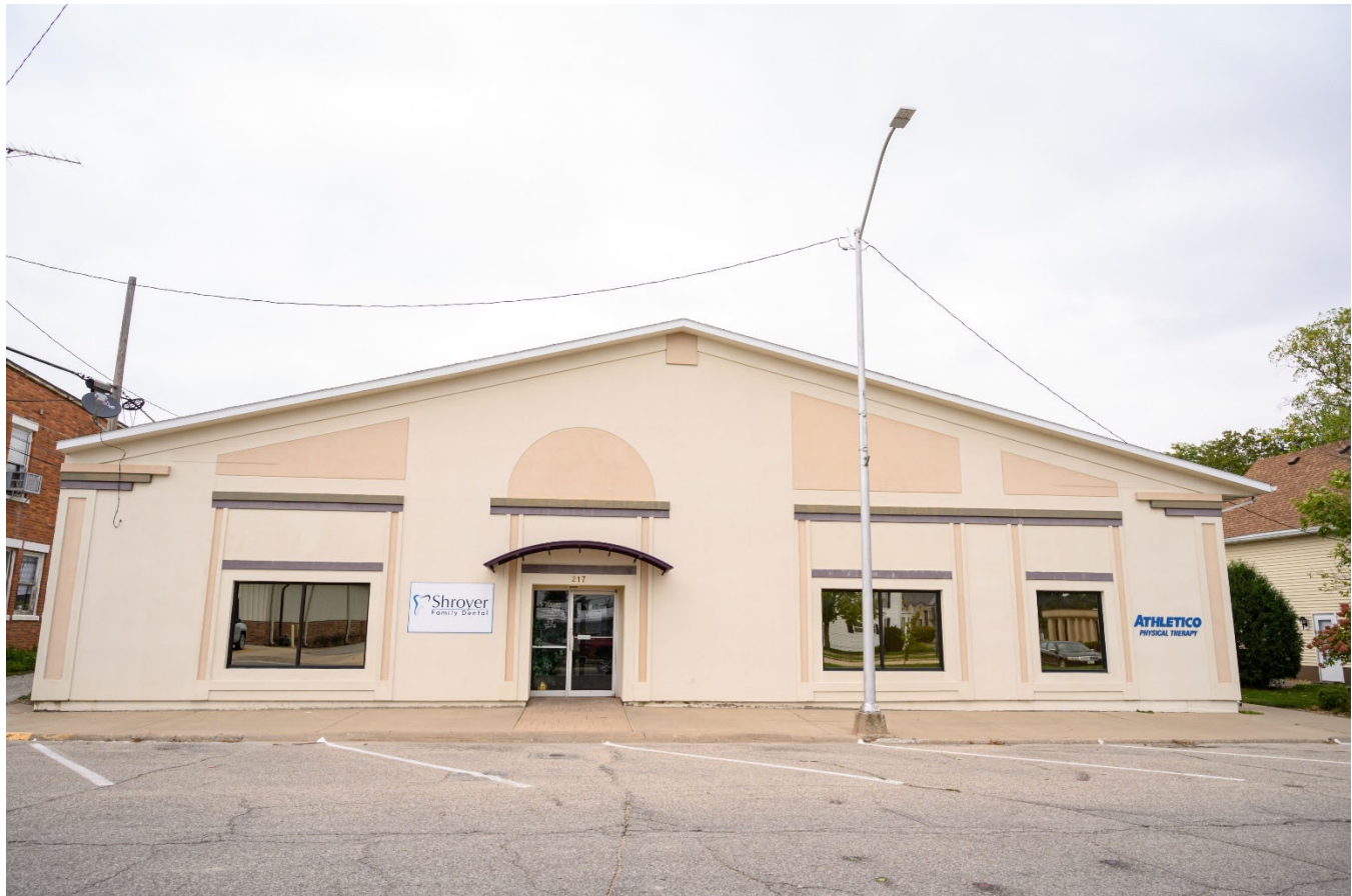
Photograph 44-002261-002. South elevation, looking north (October 2023)
