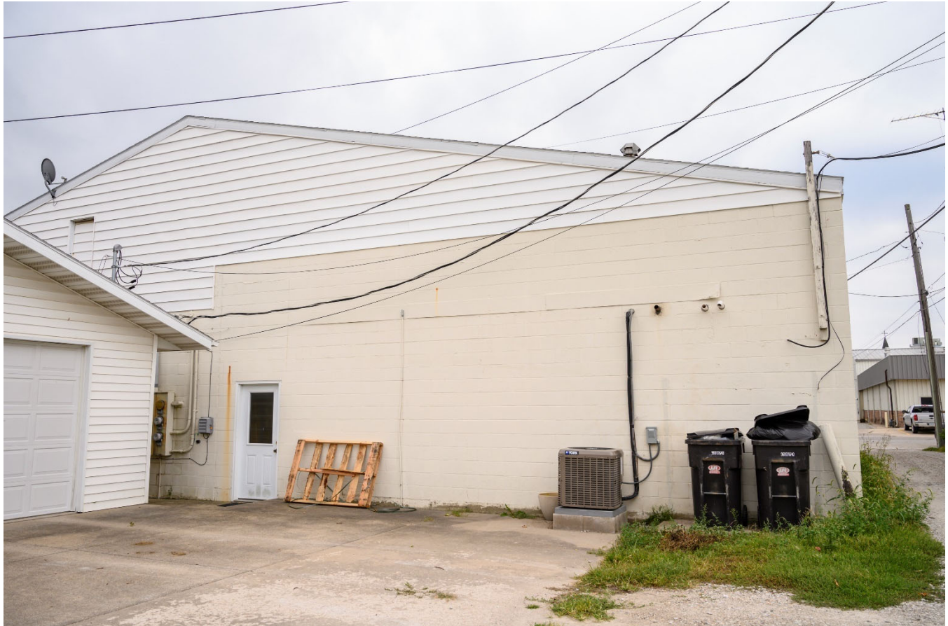
Photograph 44-002261-004. North elevation, looking south (October 2023)
