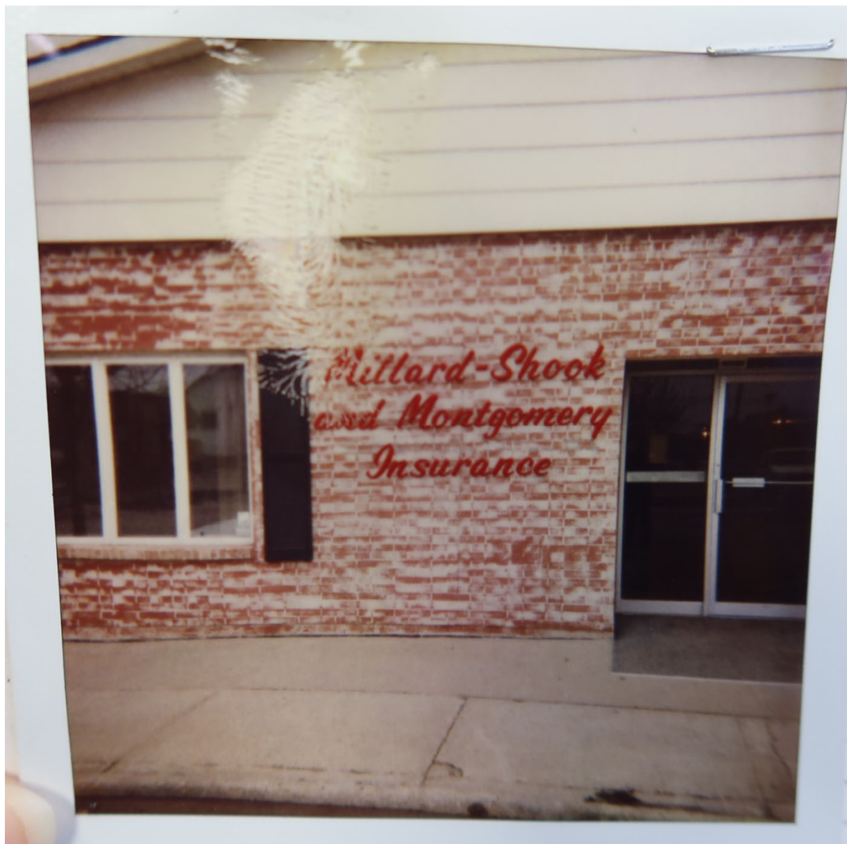
Photograph for January 1992 sign permit (City of Mt Pleasant building permits) stained brick from 1979 remodel visible
