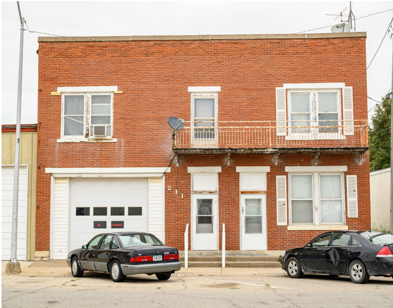
Photograph 44-02260-002. South elevation, looking north (October 2023)
