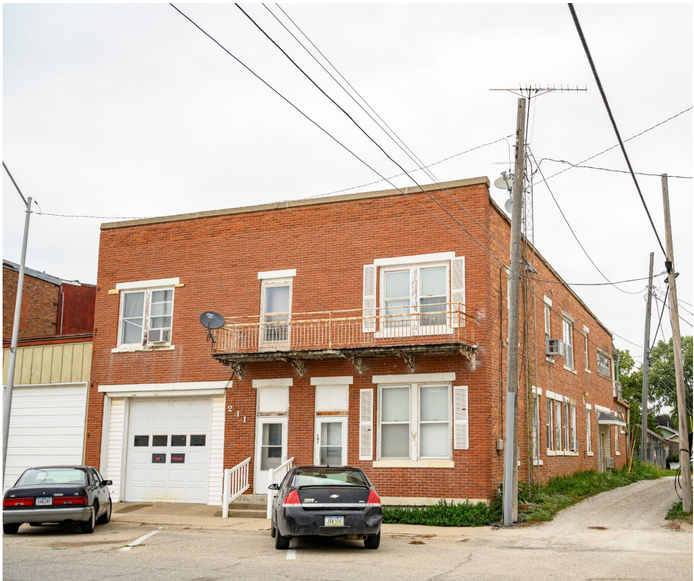
Photograph 44-02260-001. South elevation, looking northwest (October 2023)
