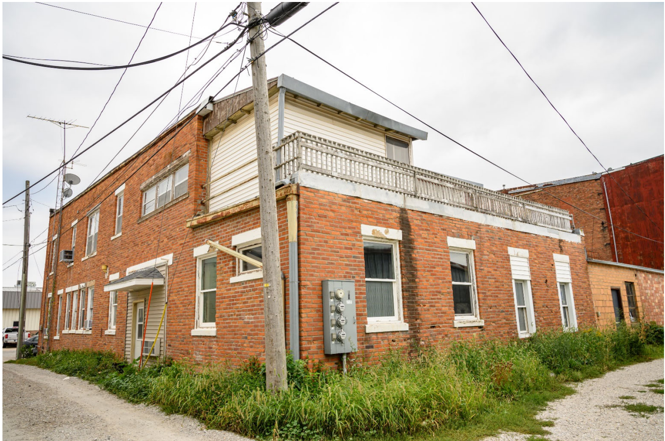
Photograph 44-02260-003. East and north elevations, looking southeast (October 2023)
