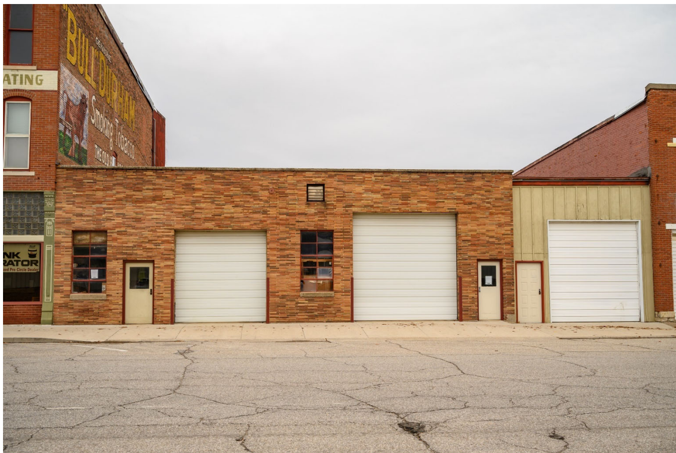
Photograph 44-02259-001. South elevation, looking north (October 2023)
