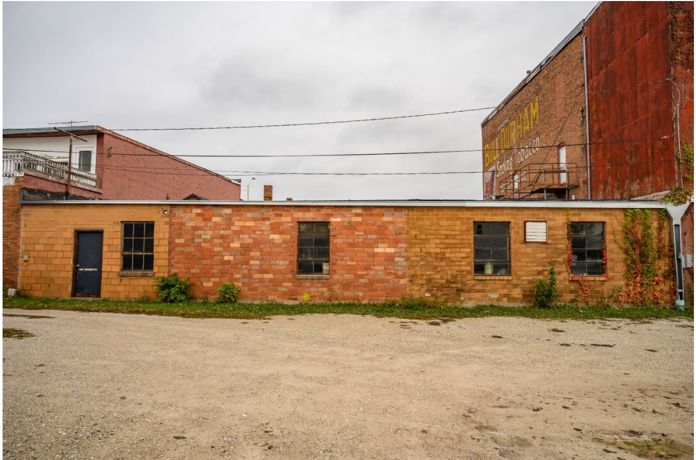
Photograph 44-02259-002. North elevation, looking south (October 2023)
