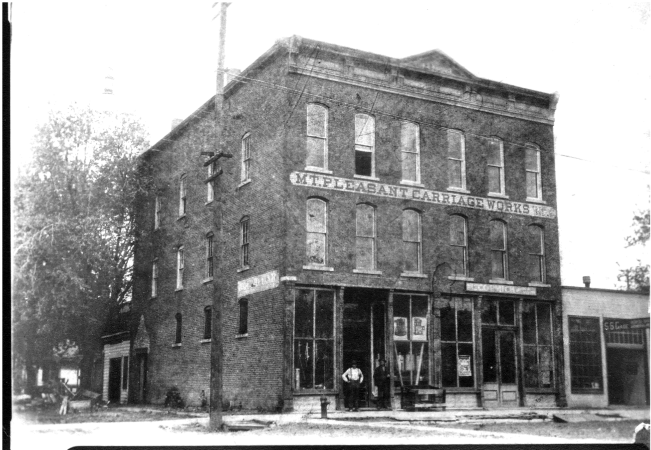
Edge of one-story building (S.S. Case) at right in 1900s (HCHT Facebook album)
