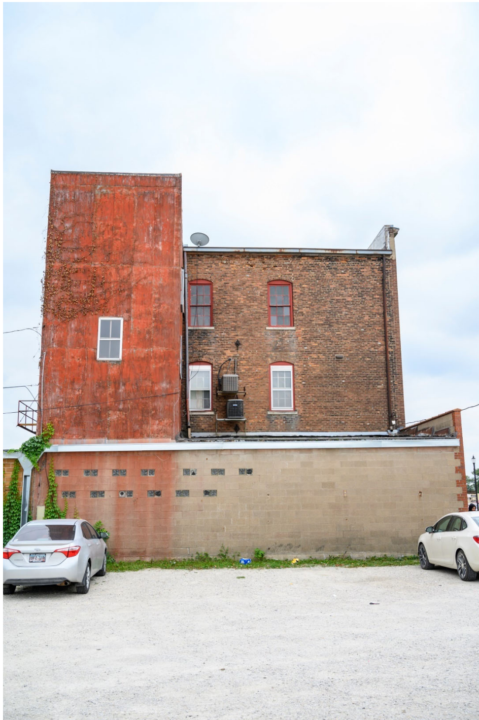
Photograph 44-00332-005. North elevations, looking south (October 2023)
