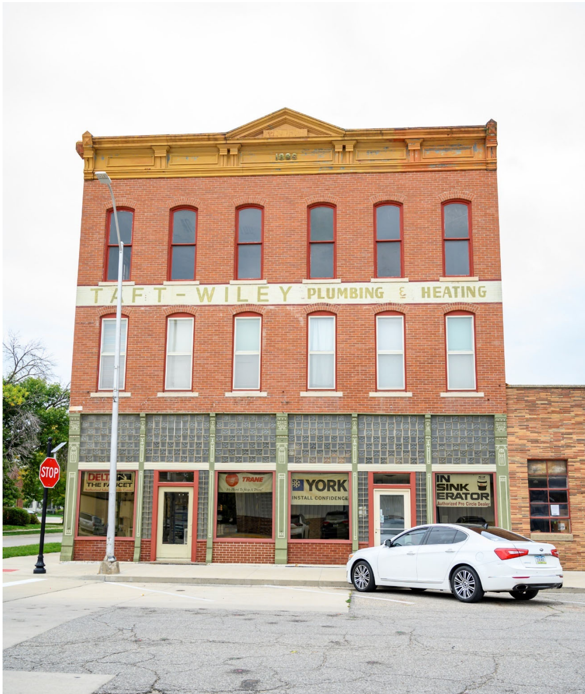
Photograph 44-00332-001. South elevation, looking north (October 2023)
