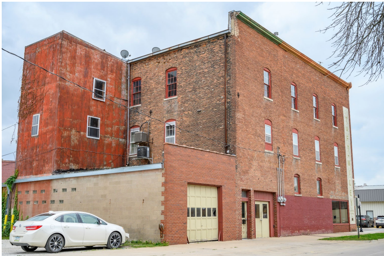
Photograph 44-00332-004. North and west elevations, looking southeast (October 2023)
