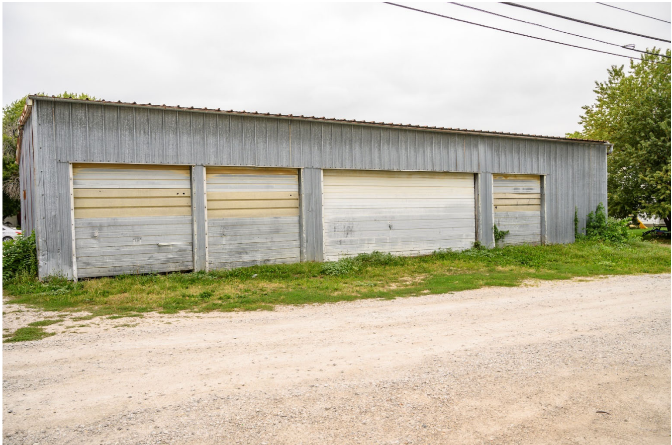
Photograph 44-02231-002. East elevation, looking west (October 2023)
