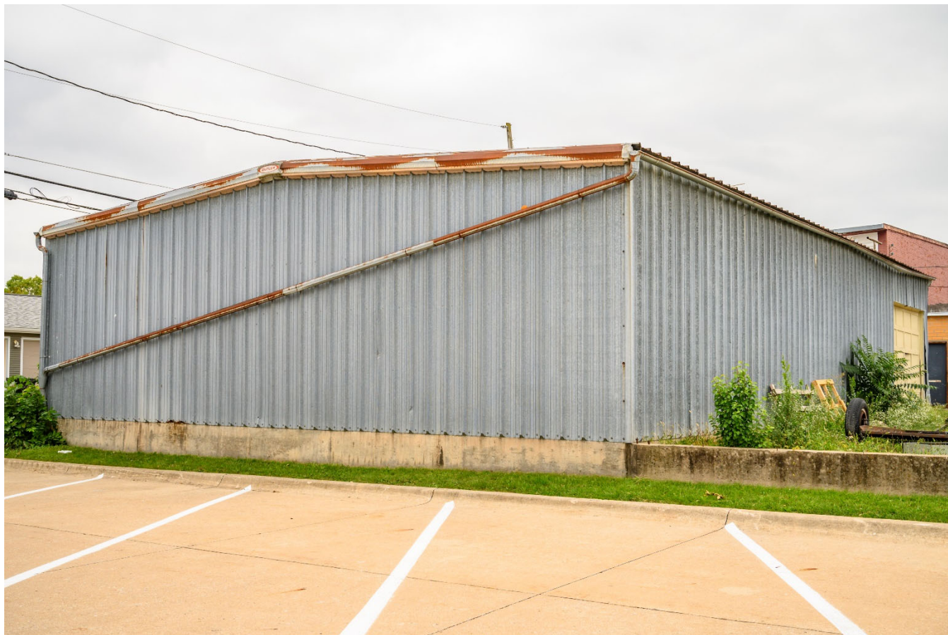
Photograph 44-02231-004. North elevation, looking southeast (October 2023)
