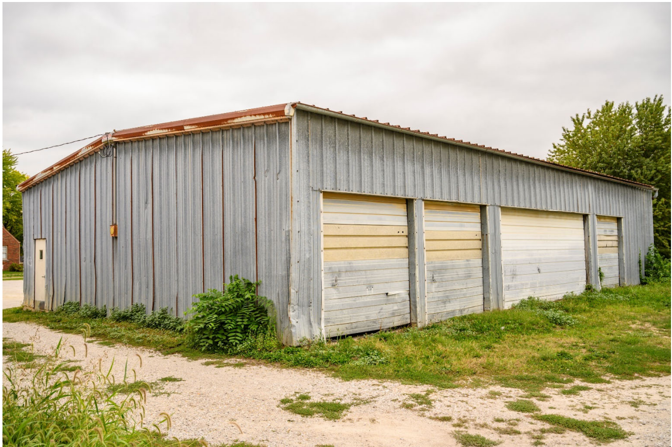
Photograph 44-02231-001. South and east elevations, looking northwest (October 2023)
