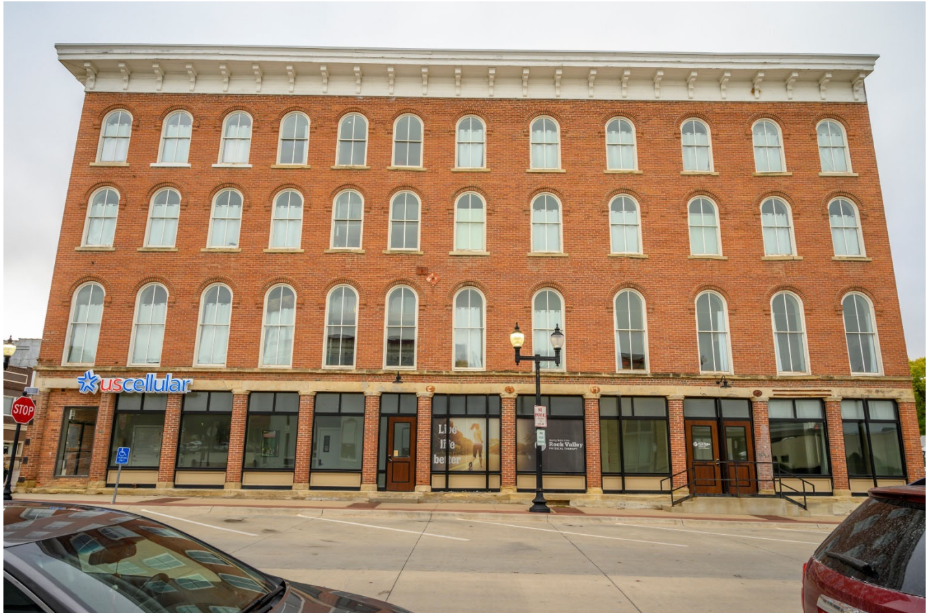
Photograph 44-00239-004. South elevation, looking north (October 2023)
