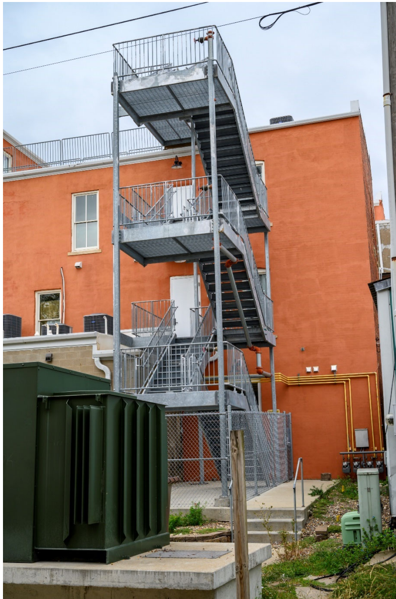
Photograph 44-00239-007. East elevation, looking west (October 2023)
