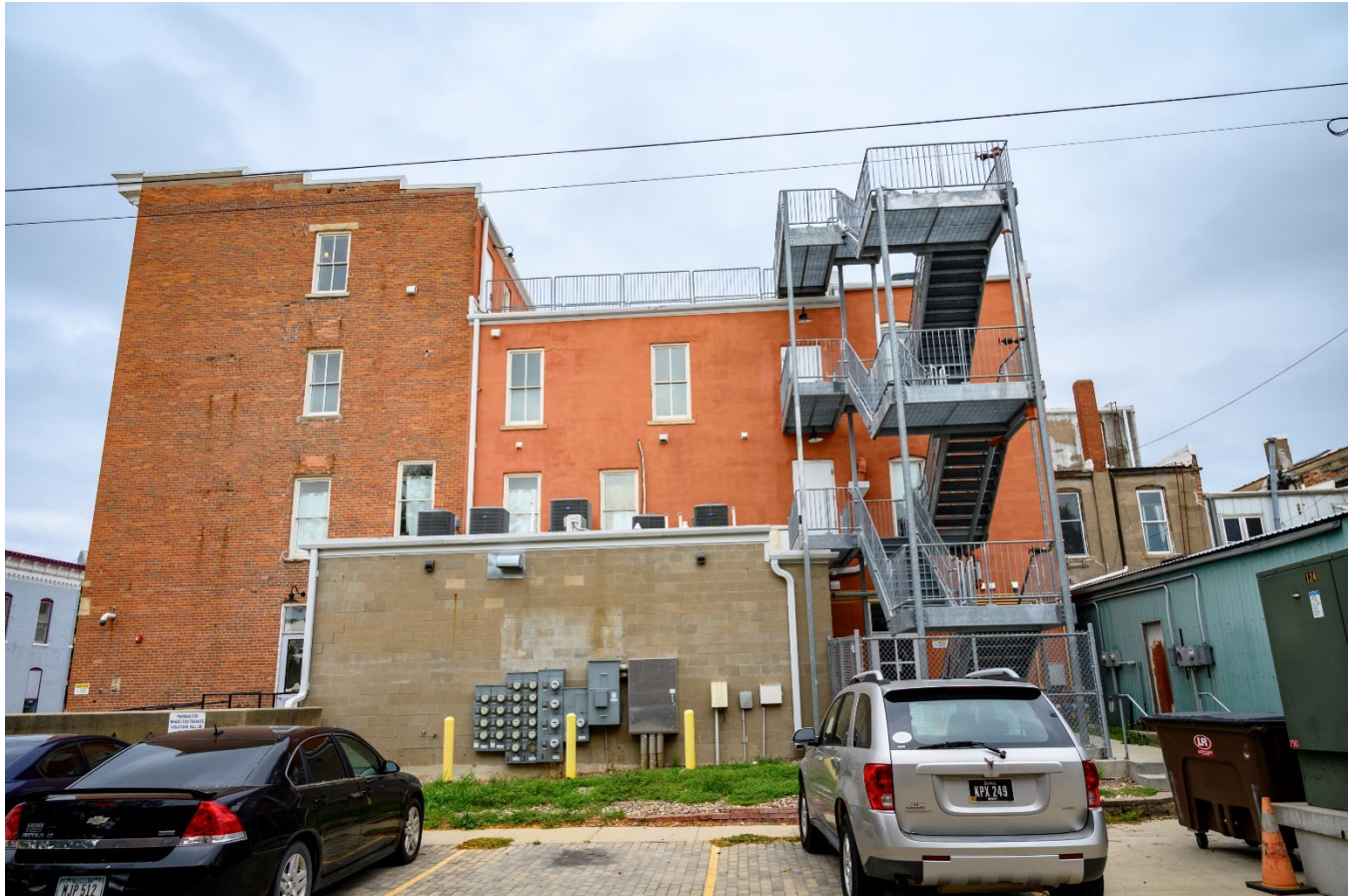
Photograph 44-00239-006. East elevation, looking west (October 2023)
