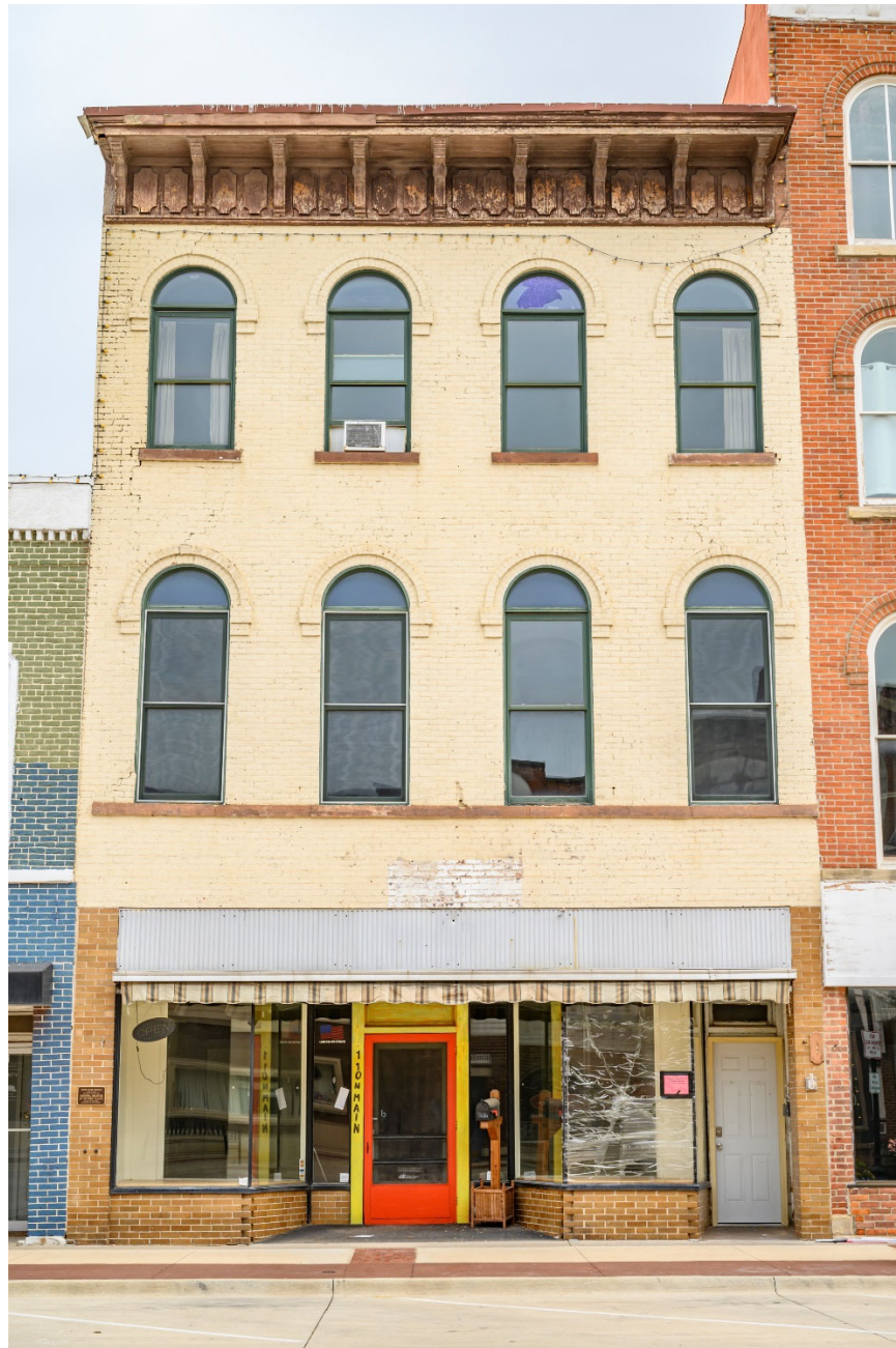
Photograph 44-00243-001. West elevation, looking east (October 2023)
