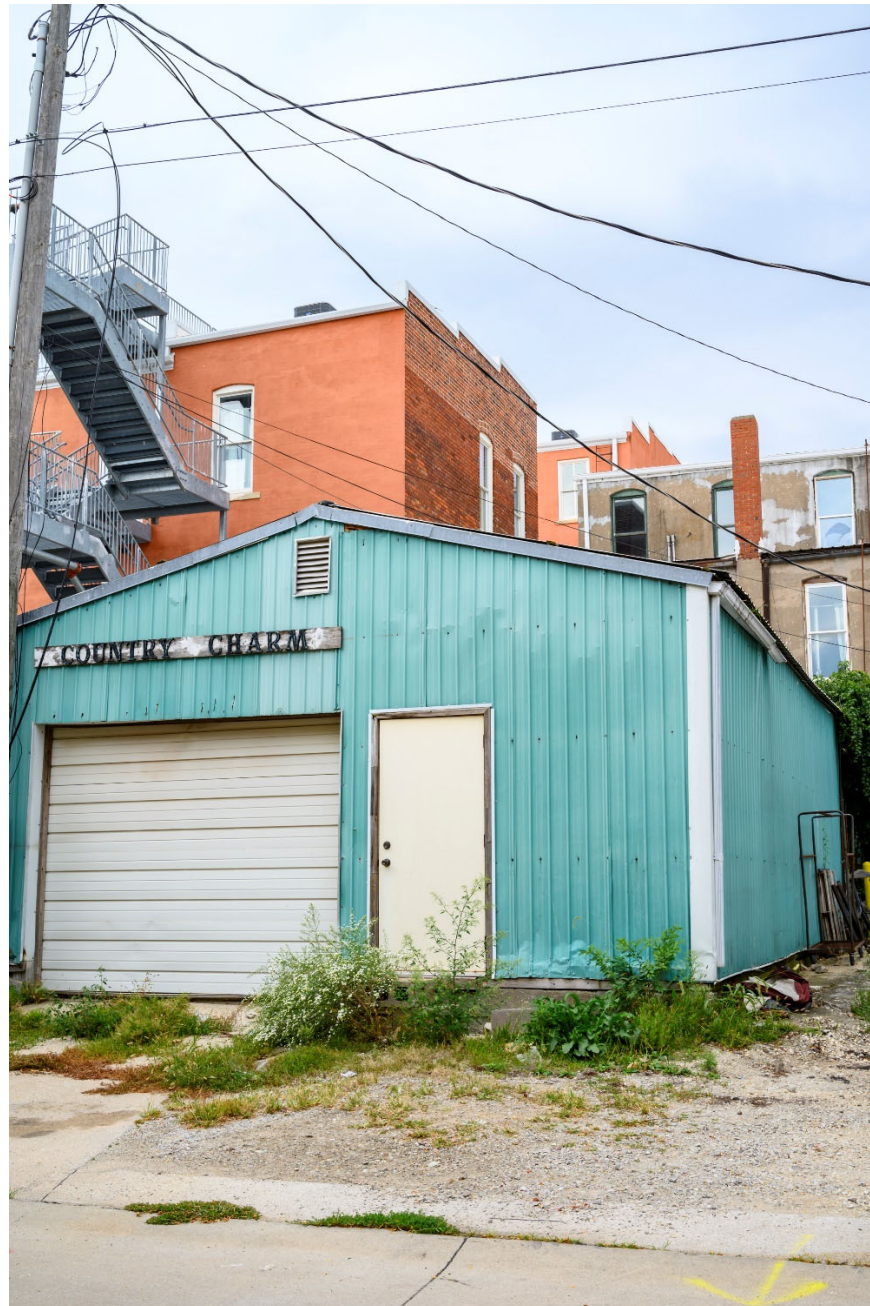
Photograph 44-00243-002. East elevation, looking west (October 2023)
