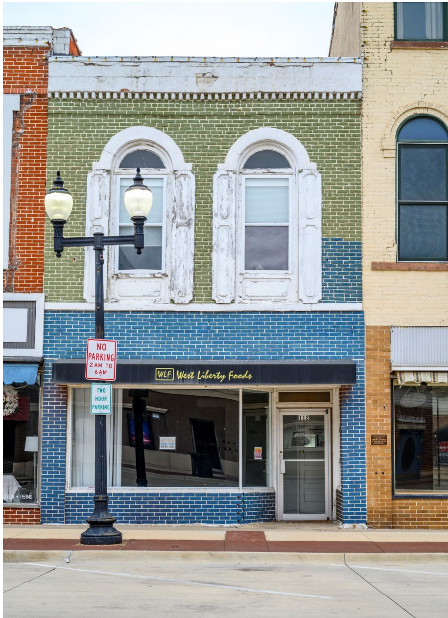
Photograph 44-00244-001. West elevation, looking east (October 2023)
