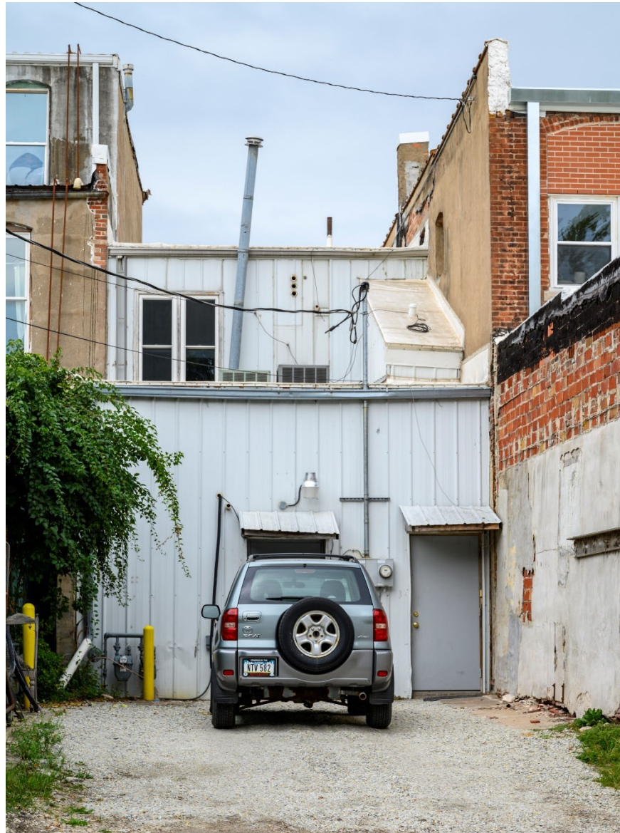
Photograph 44-00244-002. East elevation, looking west (October 2023)
