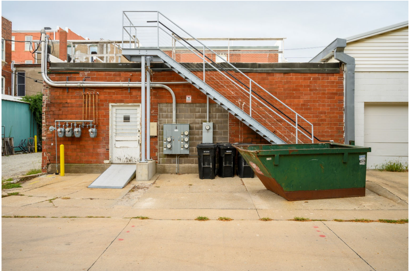
Photograph 44-00245-003. East elevation, looking west (October 2023)
