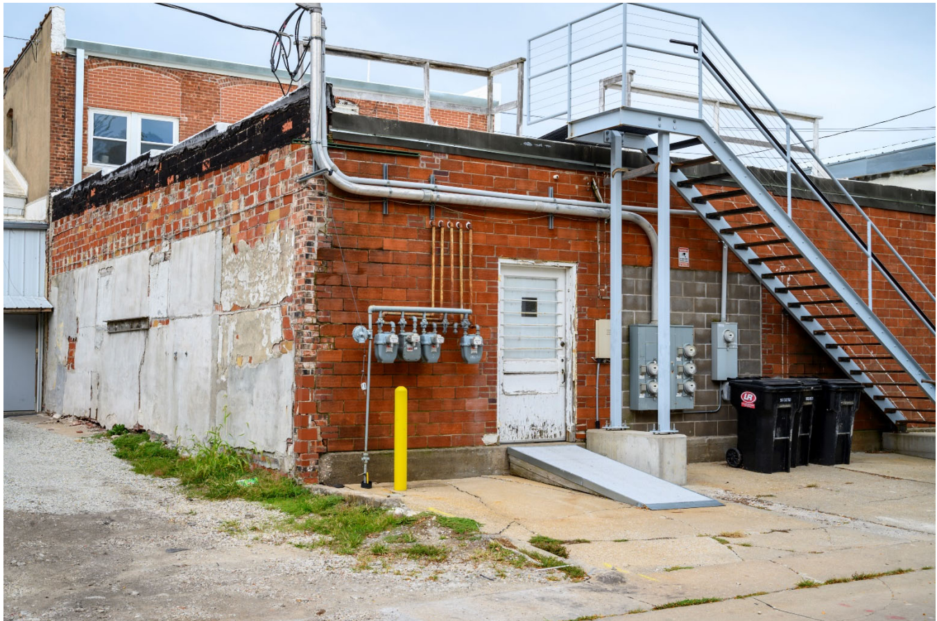
Photograph 44-00245-002. South and east elevation, looking northwest (October 2023)
