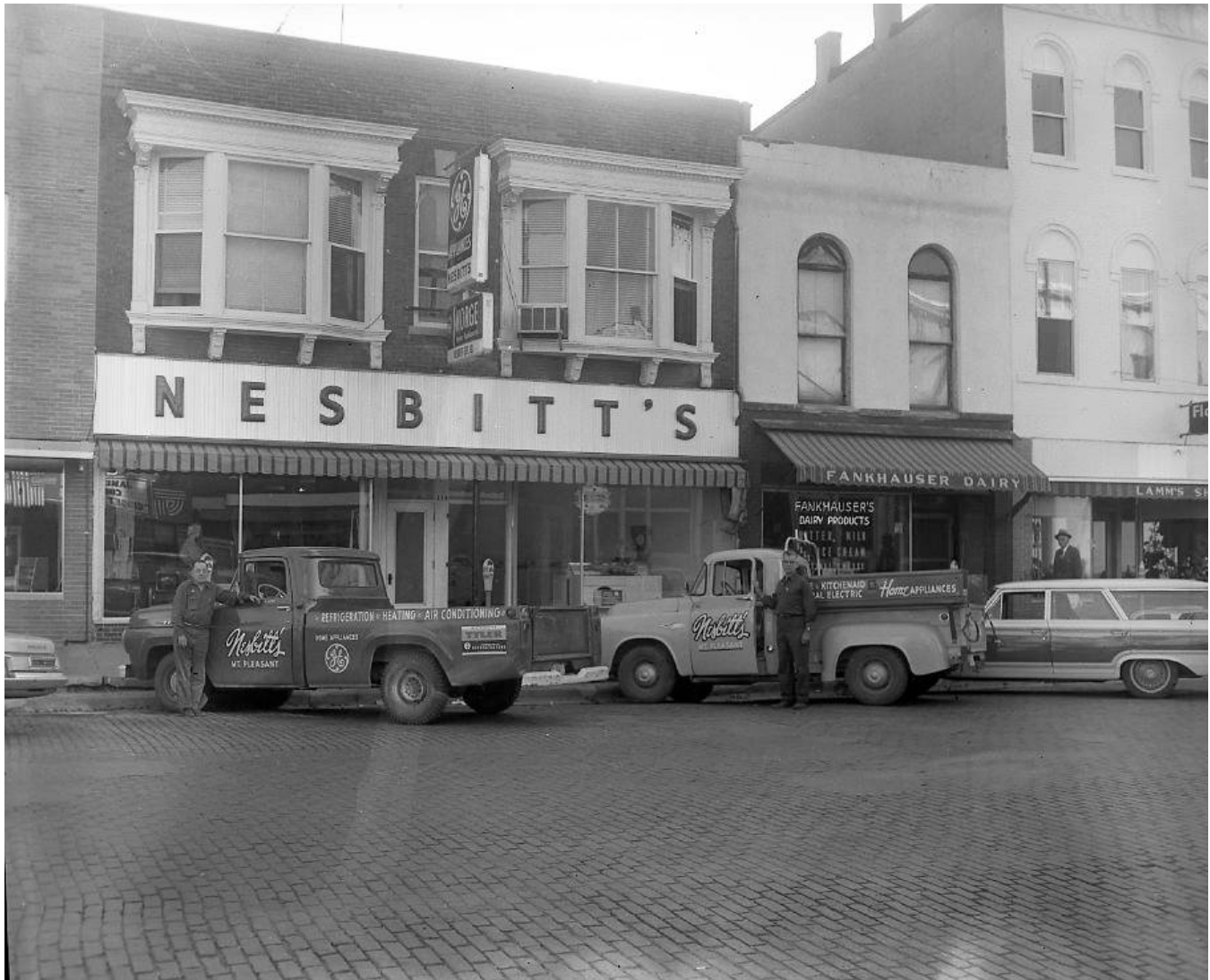
Edge of building on left on November 11, 1963 (Nesbitt's opening) (HCHT Facebook album) new façade brick by this date
