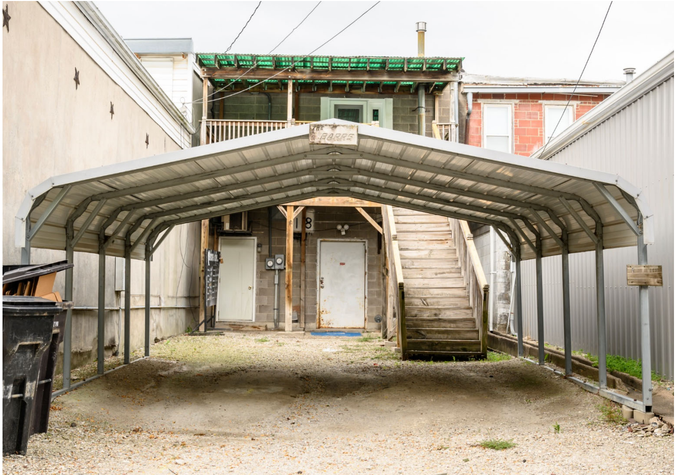
Photograph 44-00248-002. East elevation, looking west (October 2023)
