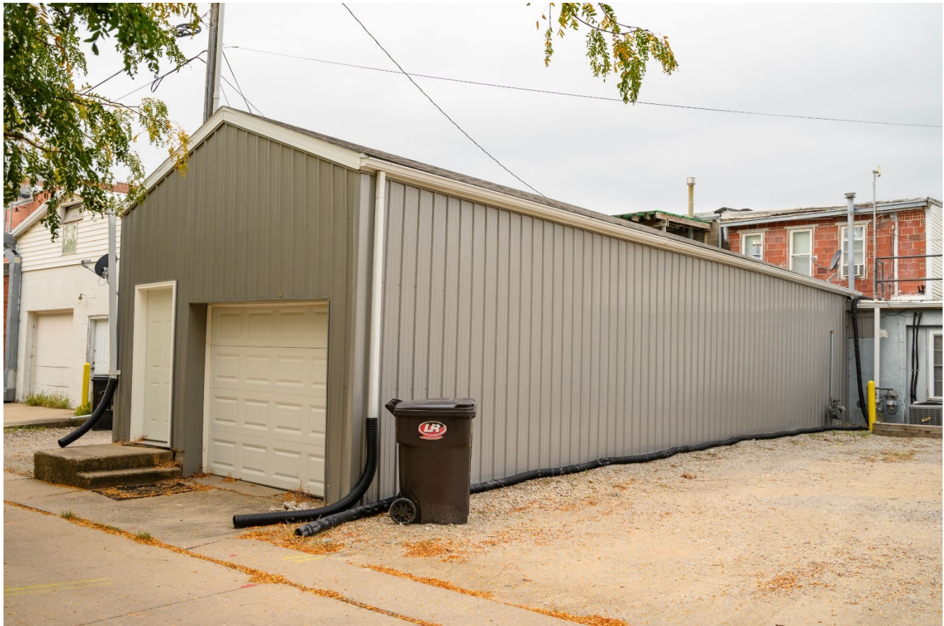
Photograph 44-00250-002. Rear addition and east elevation, looking southwest (October 2023)
