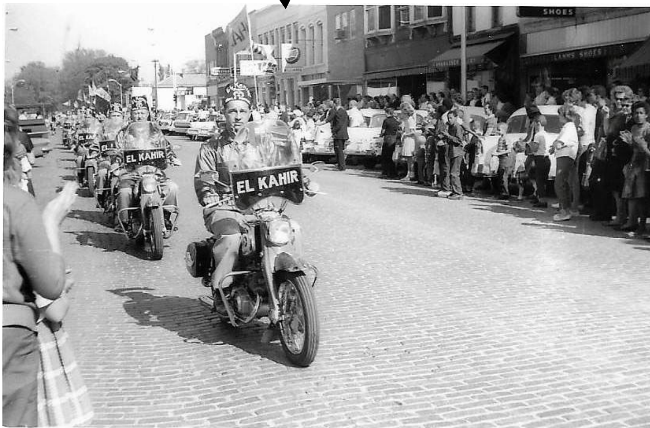
East side of 100 block of N. Main St in October 1960 (HCHT Facebook album)
