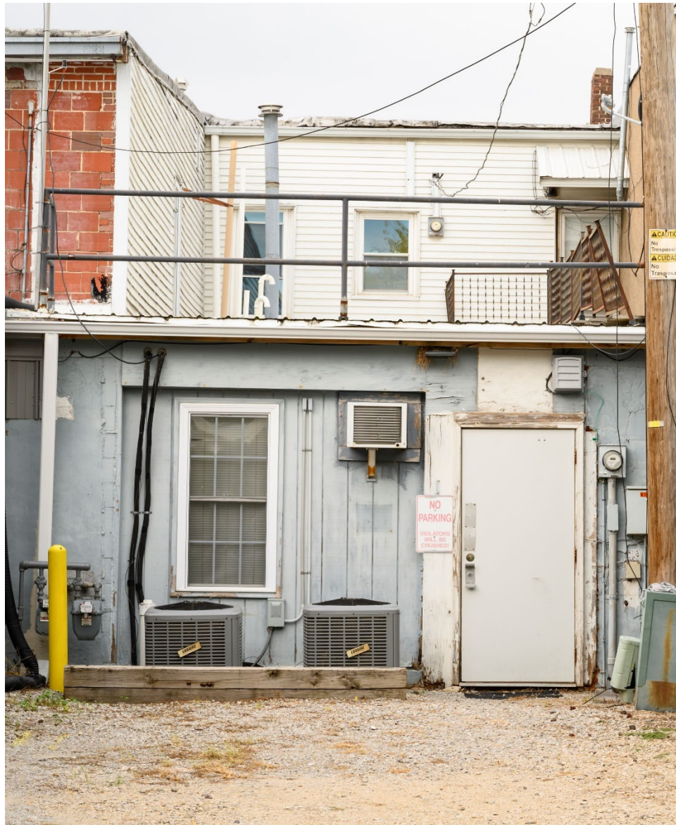
Photograph 44-00252-002. East elevation, looking west (October 2023)
