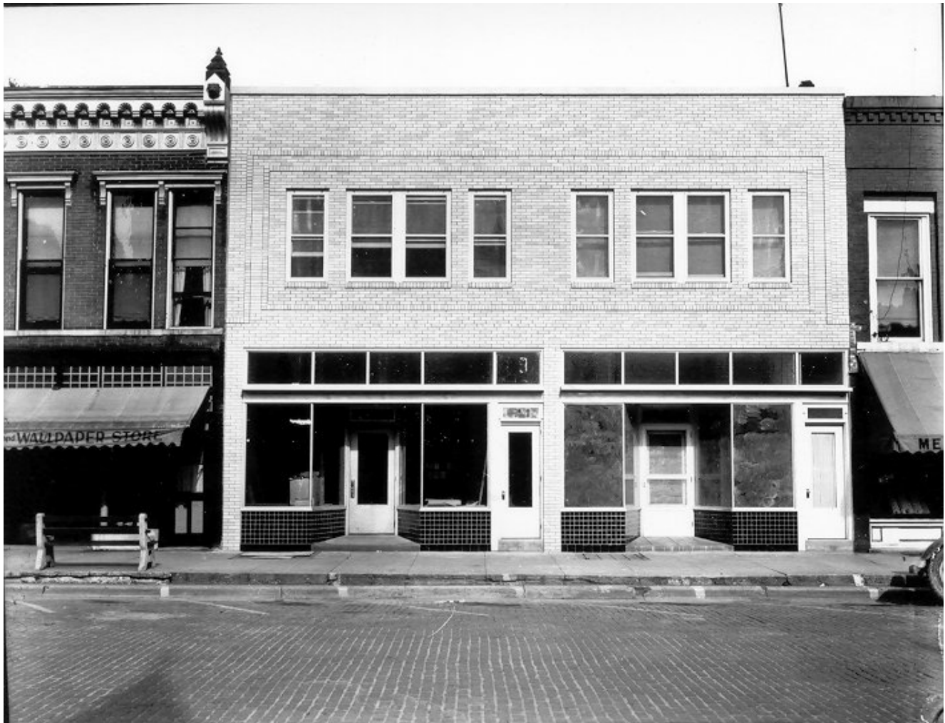
Edge of building at far right in late 1930s (HCHT Facebook album)
