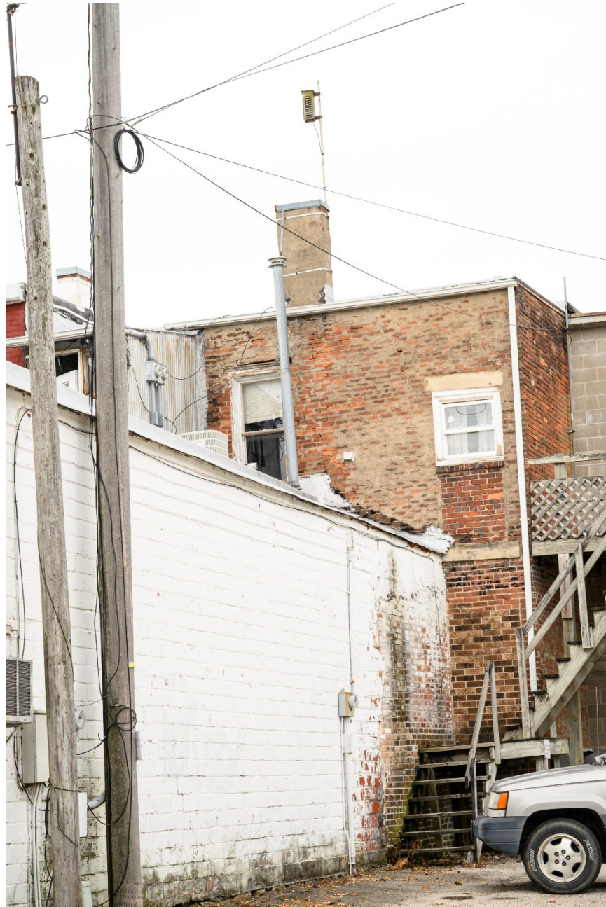
Photograph 44-00255-002. East elevation, looking southwest (October 2023)
