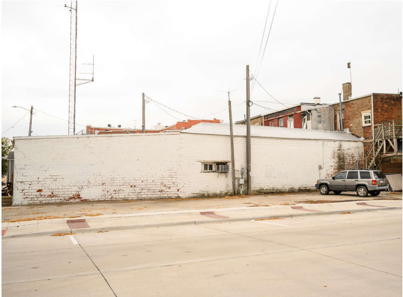
Photograph 44-00255-003. North elevation, looking south (October 2023)
