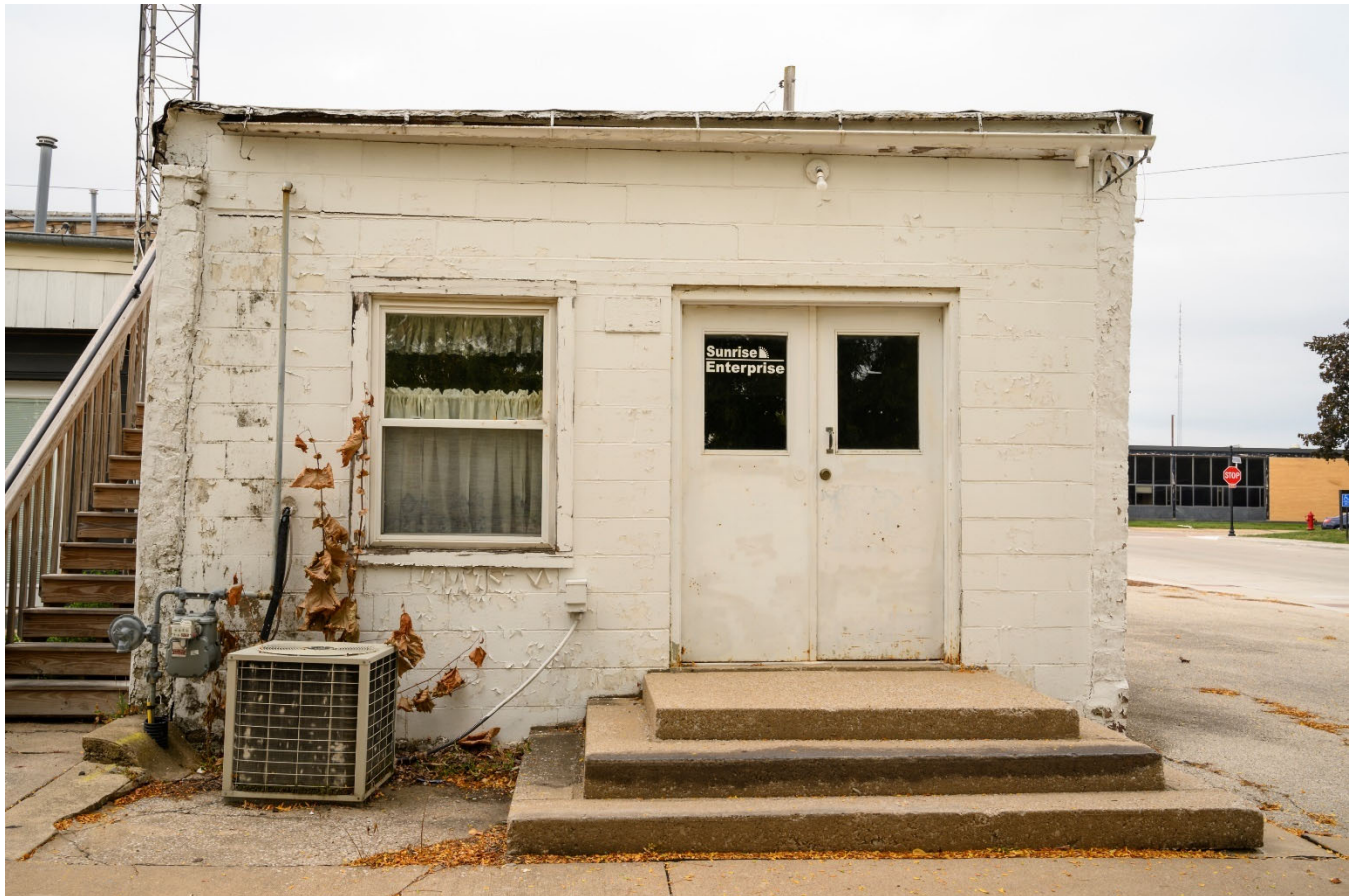
Photograph 44-00255-004. East elevation, looking west (October 2023)
