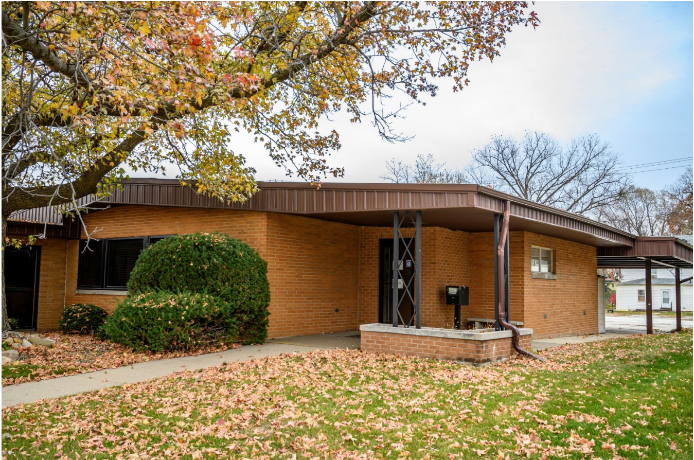
Photograph 44-02255-003. West and south elevations of original building, looking northeast (October 2023)
