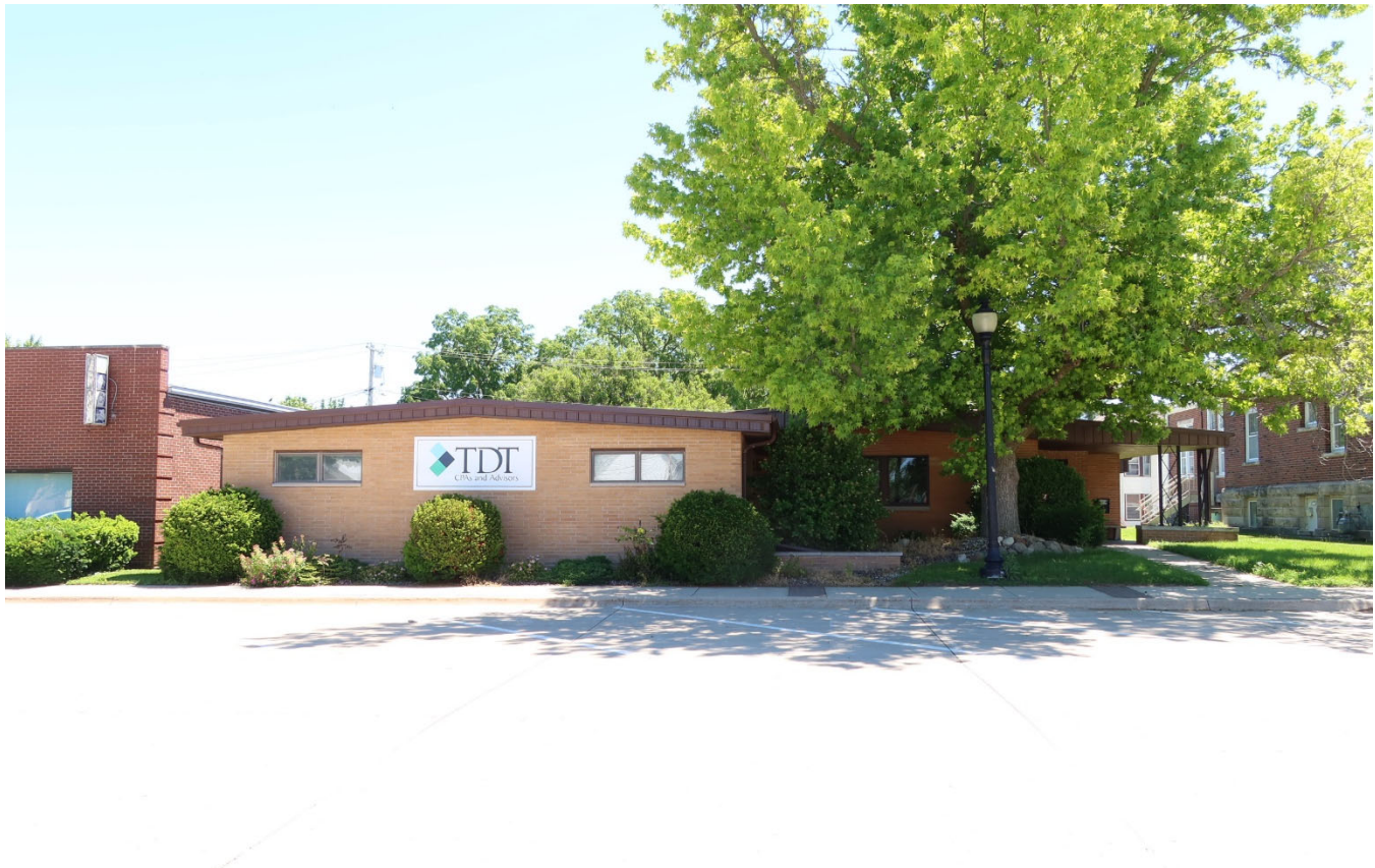
Photograph 44-02255-001. West elevation of building, looking east (June 2024)
