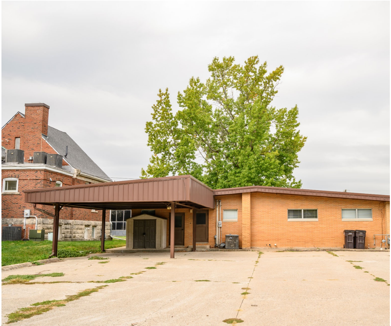
Photograph 44-02255-004. East elevations, looking west (October 2023)
