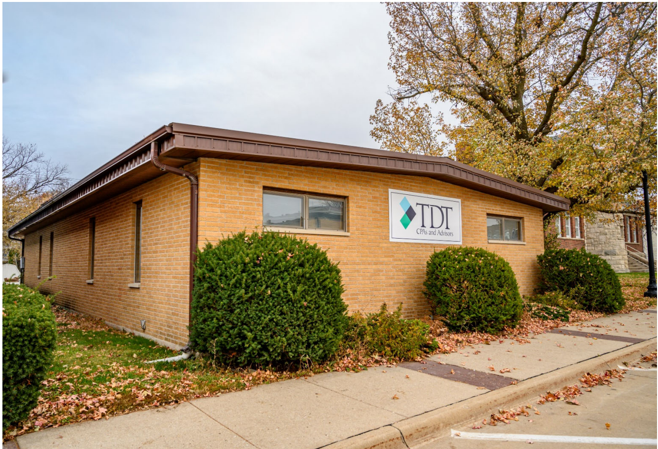
Photograph 44-02255-005. North and west elevations of north addition, looking southeast (October 2023)
