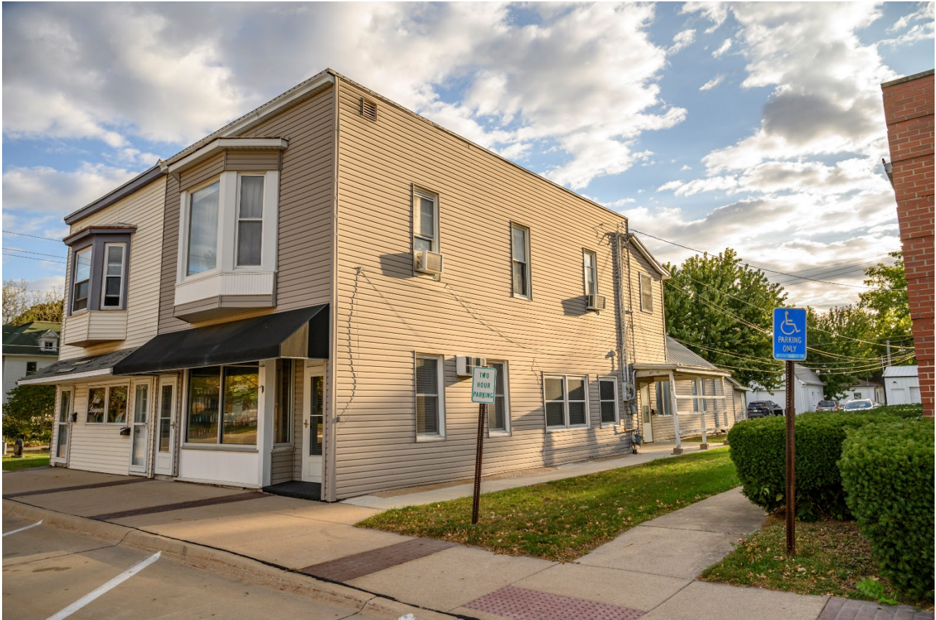
Photograph 44-00258-002. West and south elevations, looking northeast (October 2023)
