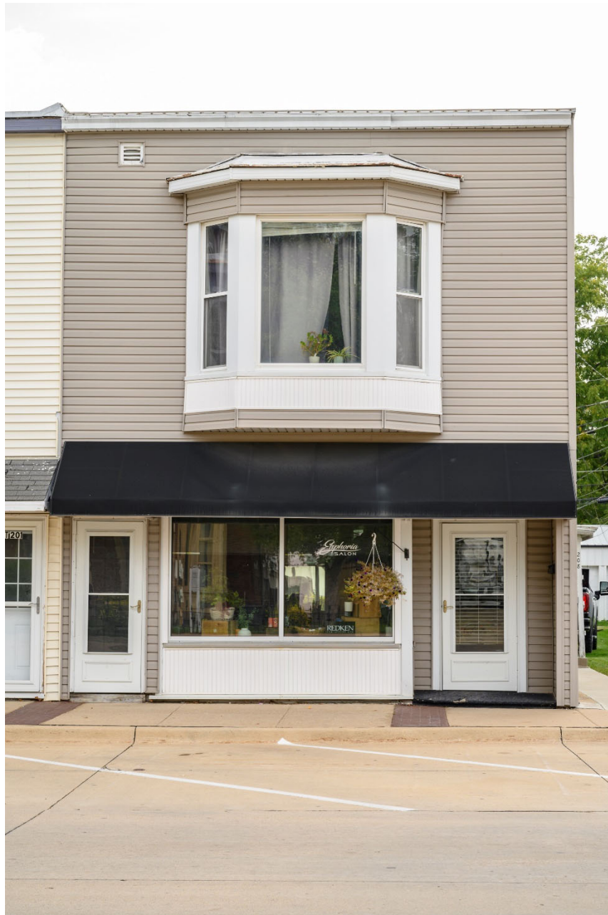
Photograph 44-00258-001. West elevation, looking east (October 2023)
