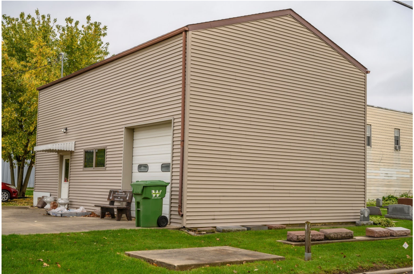
Photograph 44-02258-002. East and north elevations, looking southwest (October 2023)
