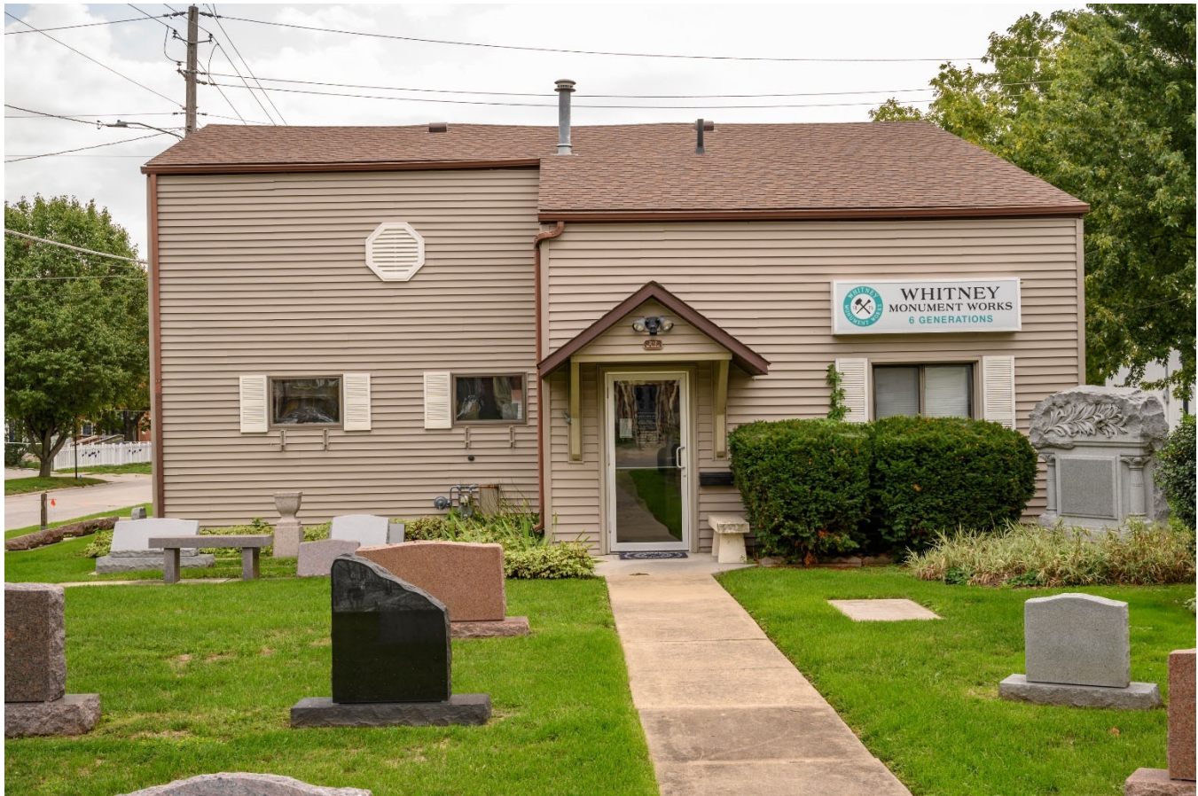
Photograph 44-02258-001. West elevation, looking east (October 2023)
