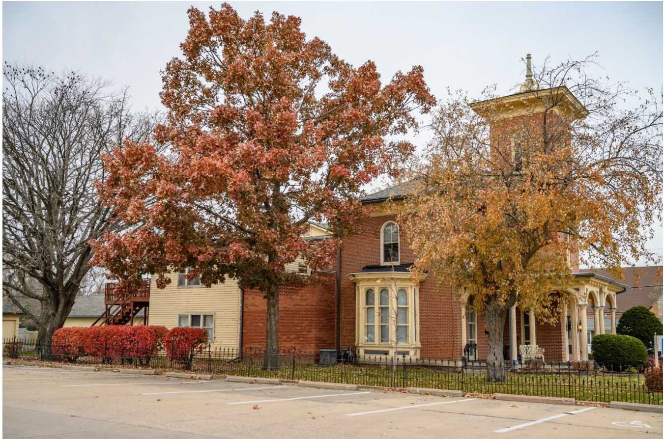
Photograph 44-00259-003. South elevation, looking northwest (October 2023)
