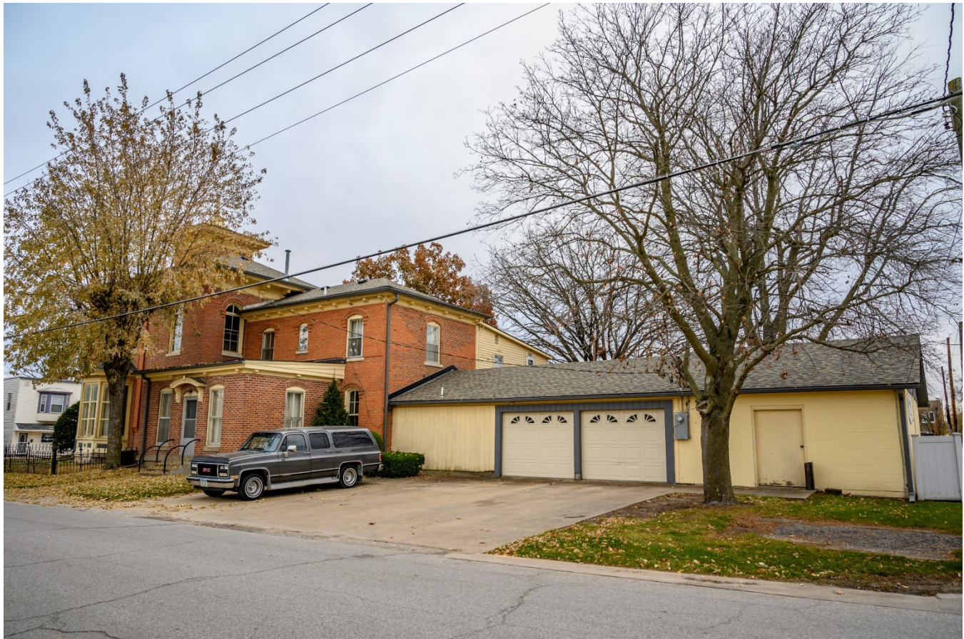
Photograph 44-00259-005. North and west elevations, looking southeast (October 2023)
