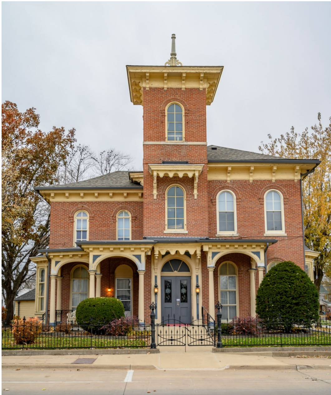
Photograph 44-00259-001. East elevation, looking west (October 2023)
