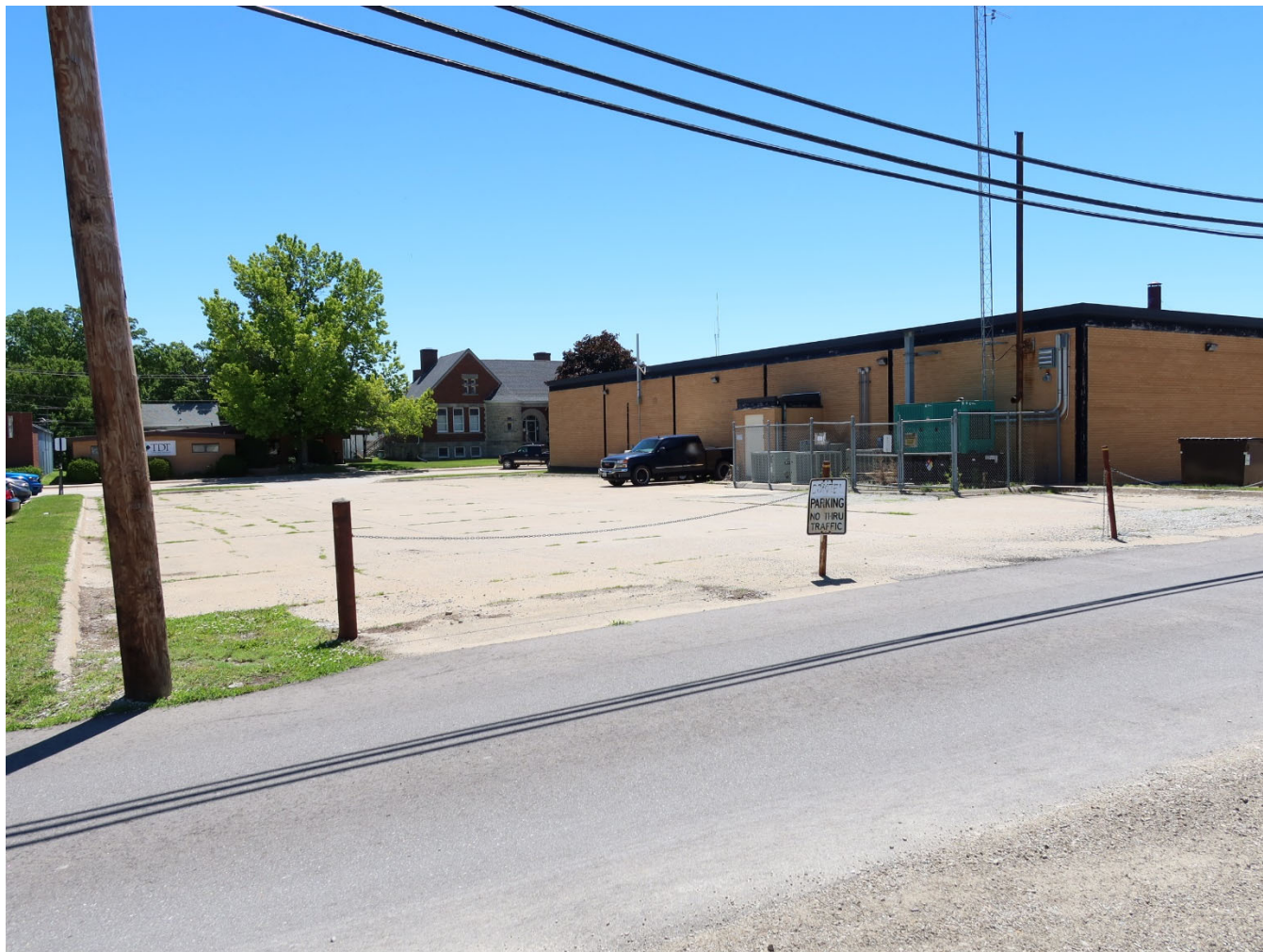
Photograph 44-02252-005. Parking lot, looking southeast (October 2023)
