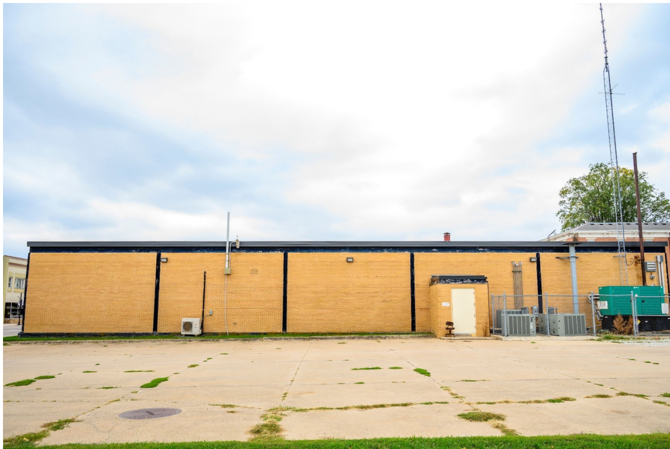
Photograph 44-02252-003. North elevation, looking south (October 2023)
