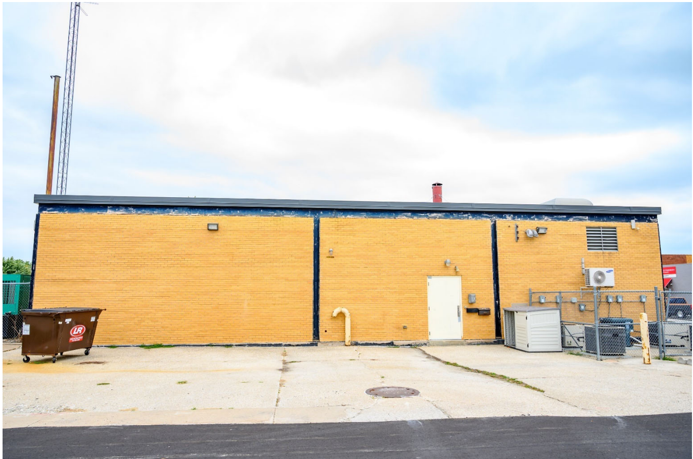
Photograph 44-02252-002. West elevation, looking east (October 2023)
