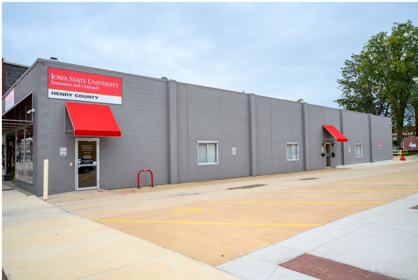
Photograph 44-00254-003. North elevation, looking southwest (October 2023)
