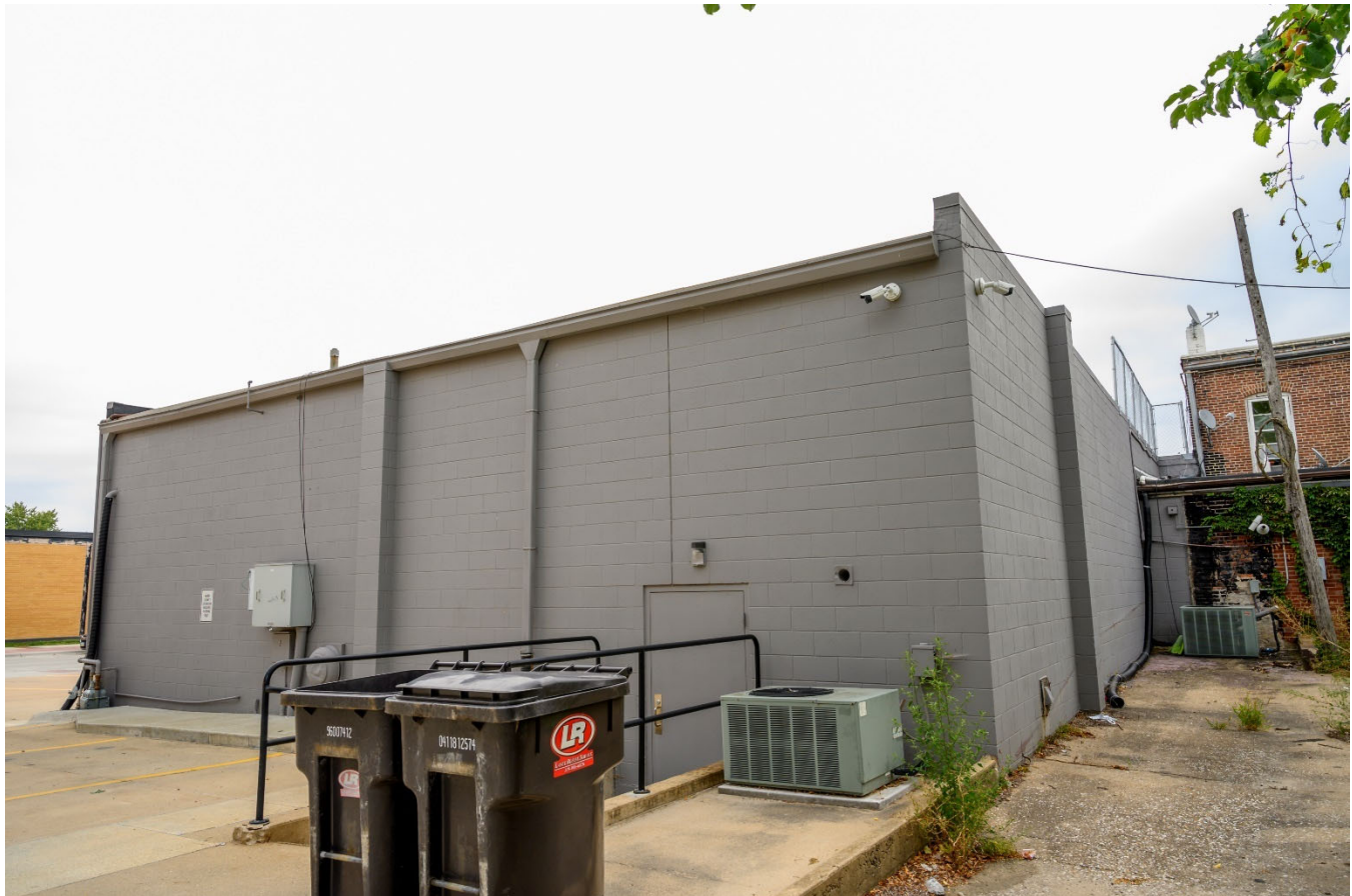
Photograph 44-00254-004. West and south elevations, looking northeast (October 2023)
