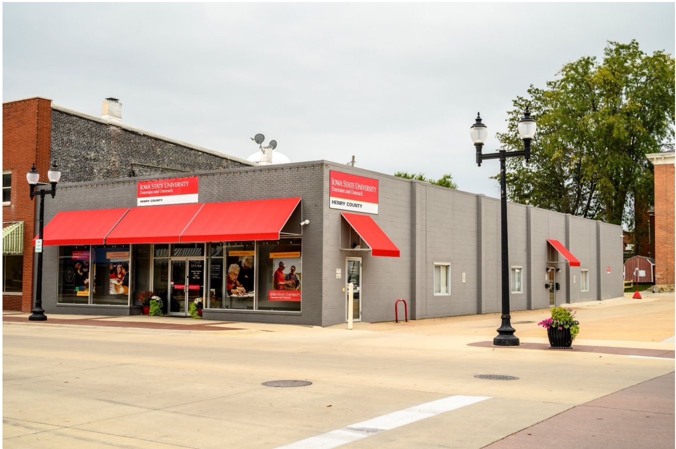
Photograph 44-00254-001. East and north elevations, looking southwest (October 2023)
