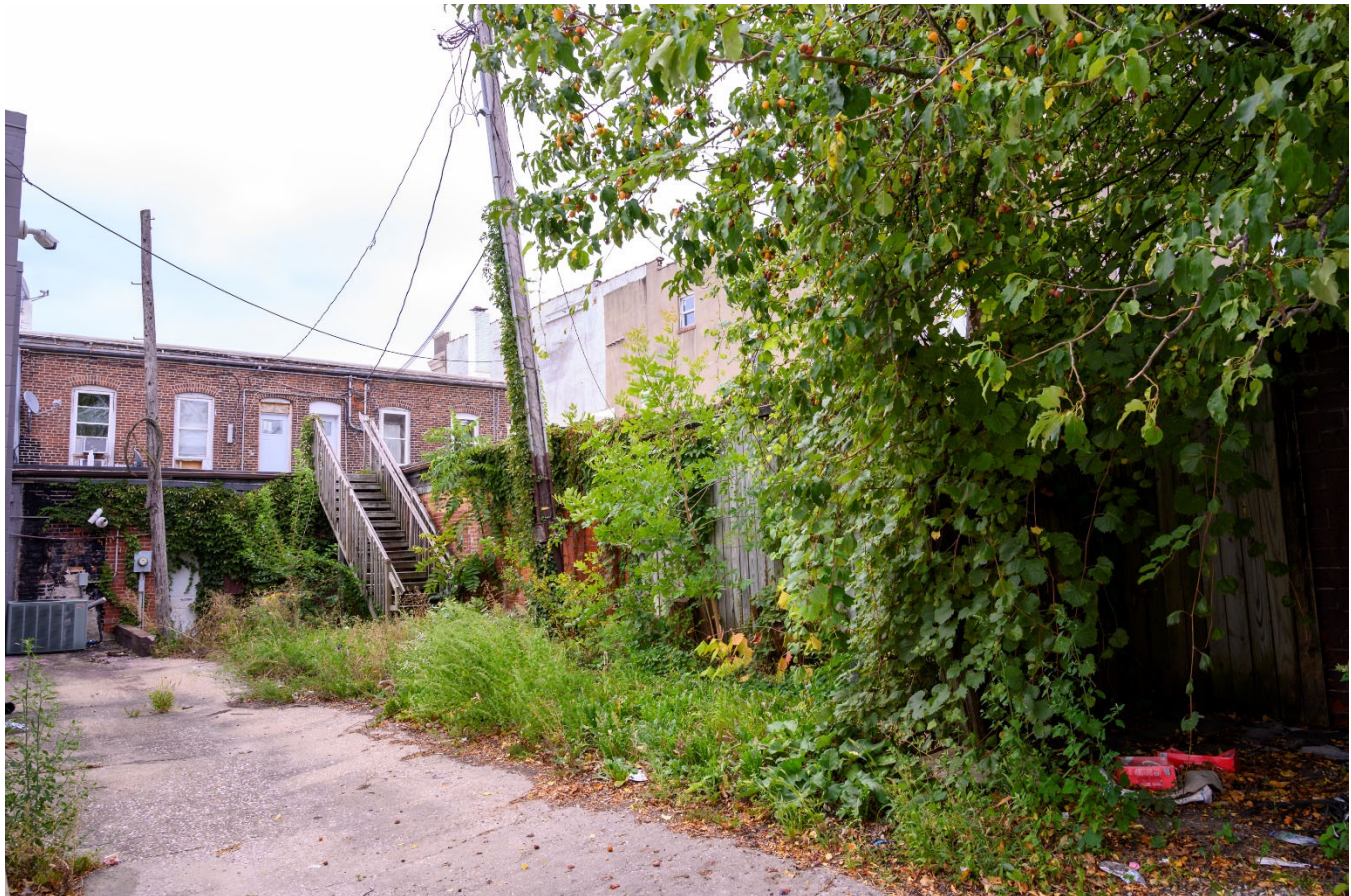
Photograph 44-00251-003. West elevation, looking southeast (October 2023)
