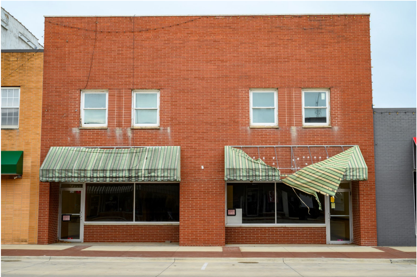
Photograph 44-00251-001. East elevation, looking west (October 2023)
