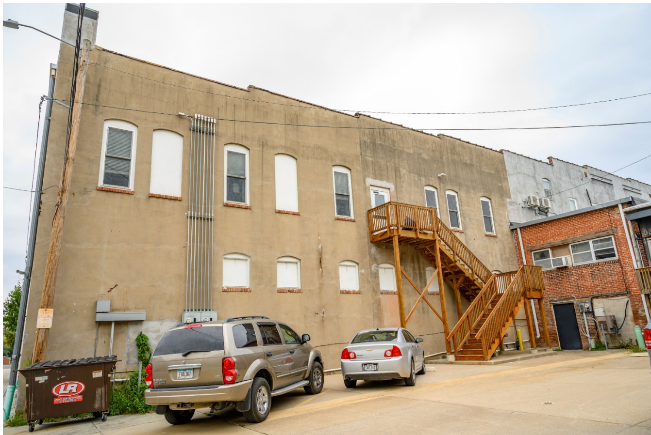
Photograph 44-00246-002. South elevation, looking north (October 2023)
