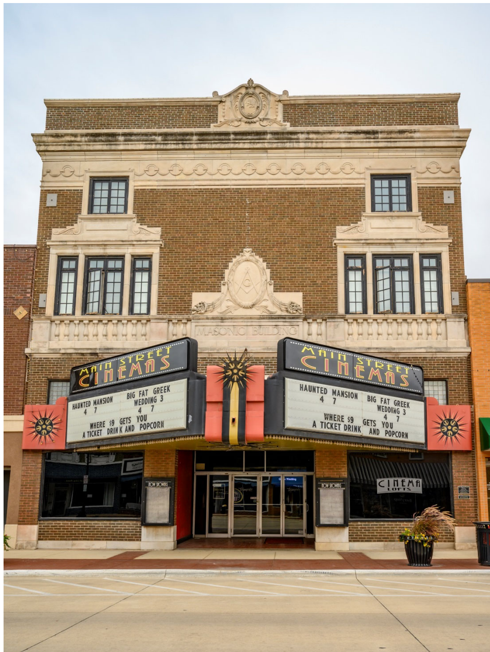
Photograph 44-00246-001. East elevation, looking west (October 2023)
