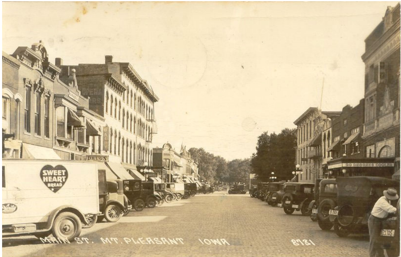
100 block of N. Main St in late 1920s, looking south (HCHT Facebook album)
