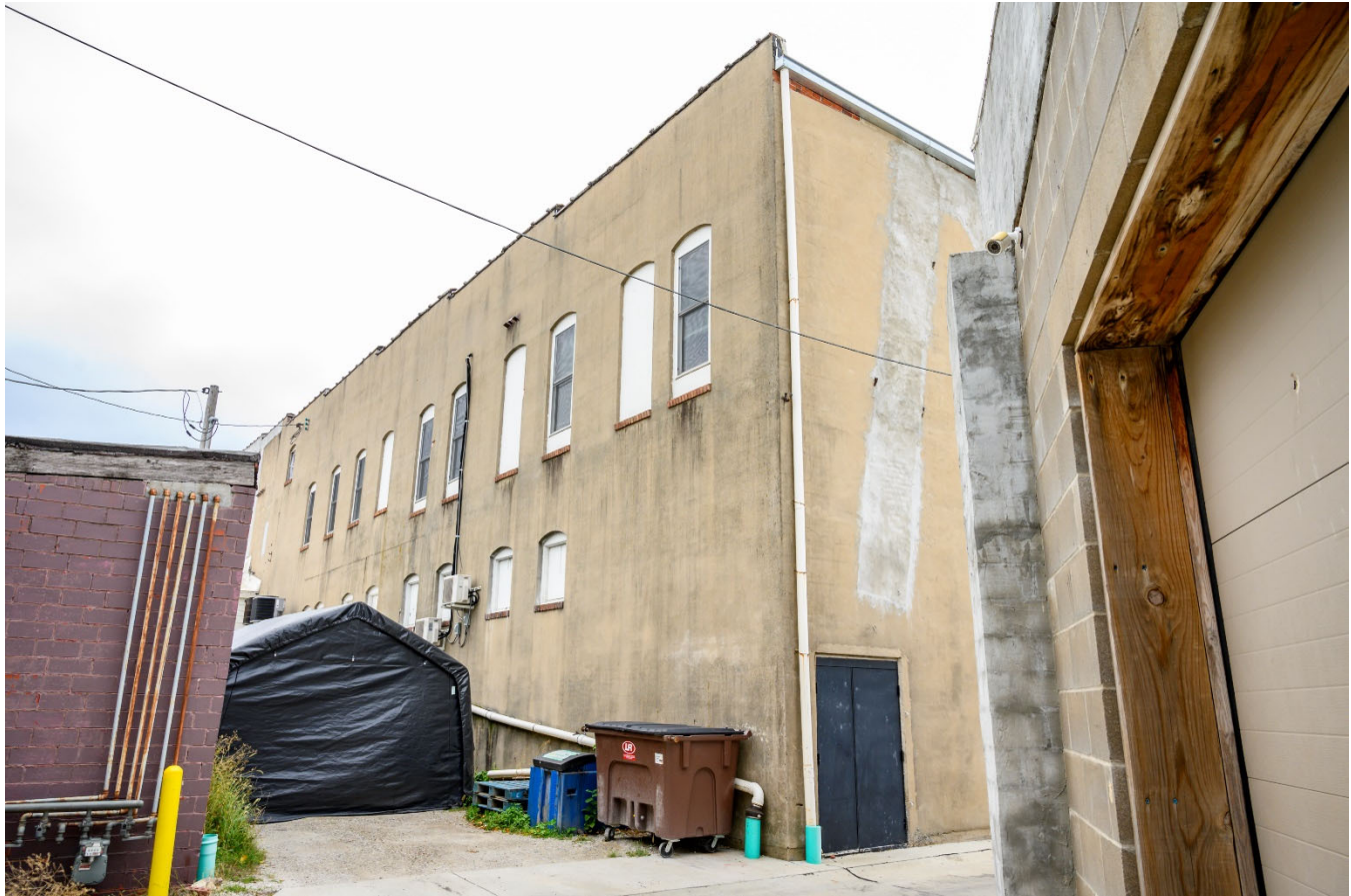
Photograph 44-00246-003. North elevation, looking southeast (October 2023)
