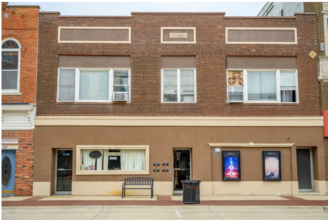
Photograph 44-00242-001. East elevation, looking west (October 2023)
