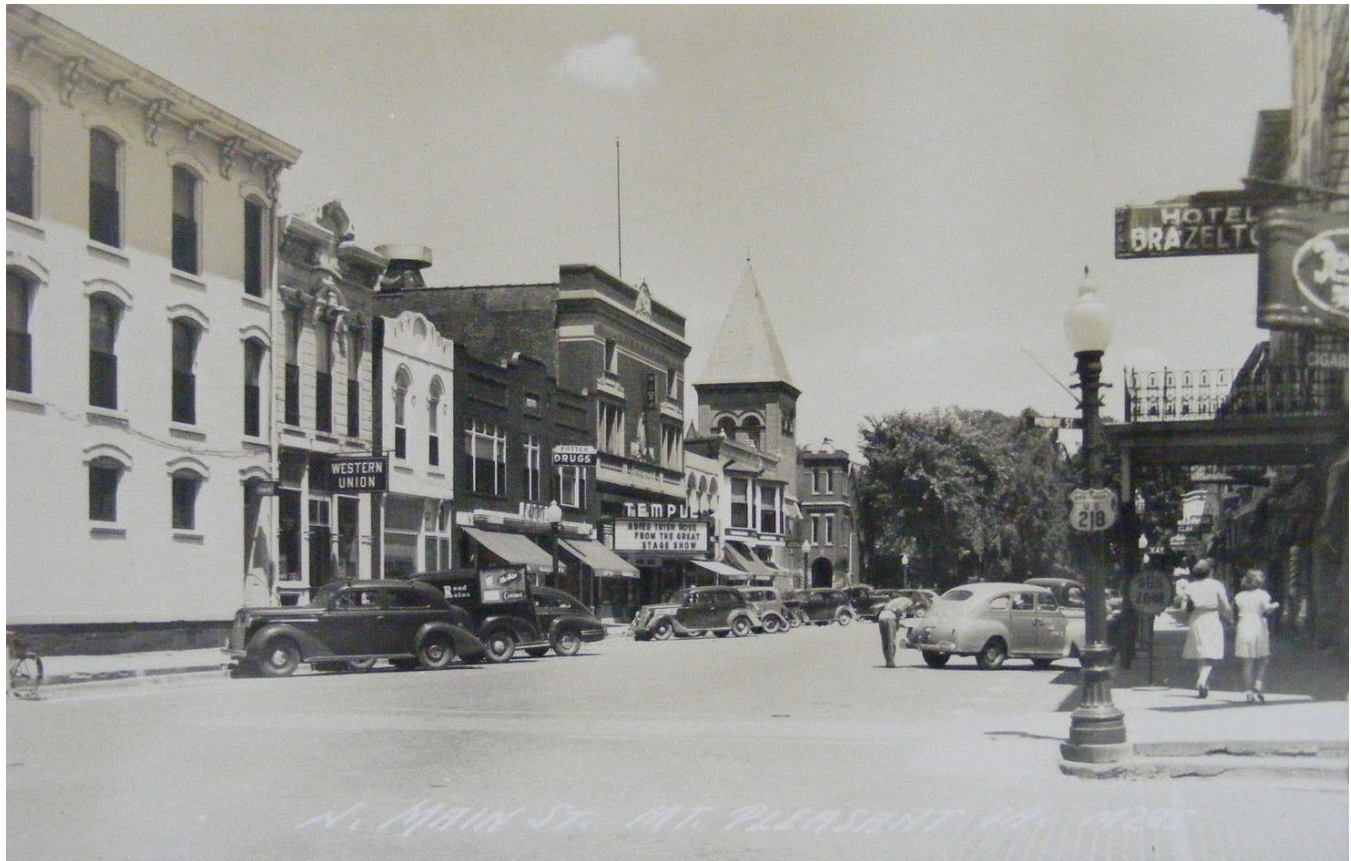
West side of 100 block of N. Main St in late 1940s (HCHT files)
