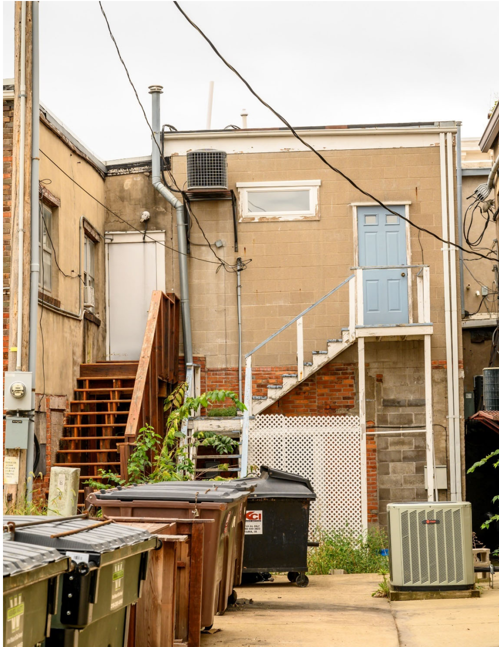
Photograph 44-00241-002. West elevation, looking east (October 2023)
