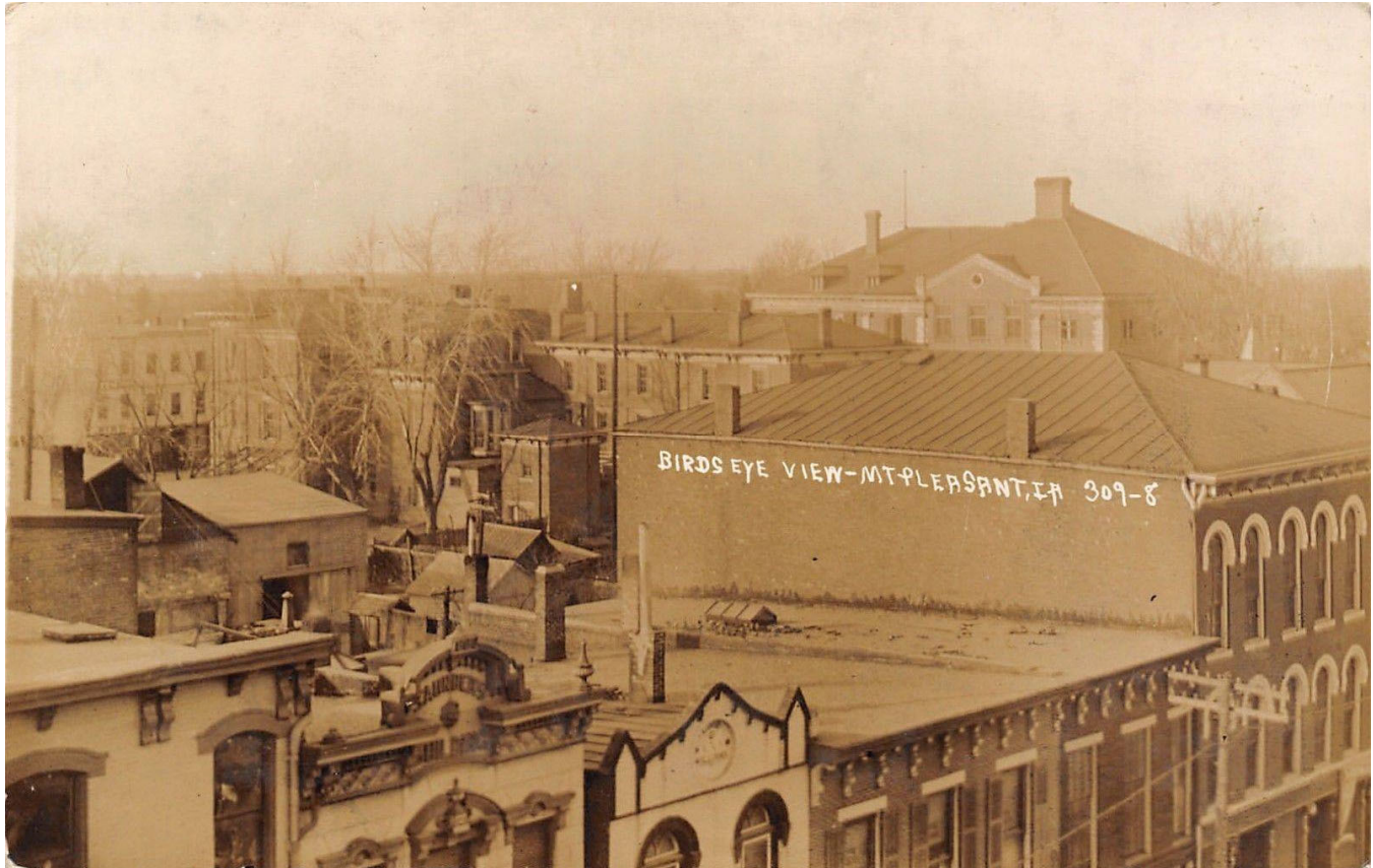
Gable cornice of building visible (HCHT Facebook album)
